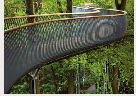
The Viper Elevated Walkway at the Newt in Somers Castle Cary, UK Submitted by: Henry Fagan & Partners
