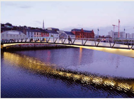
Mary Elmes Bridge Cork City, Ireland Submitted by: Arup
