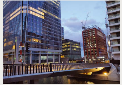
Water Street Bridge London, UK Submitted by: COWI
