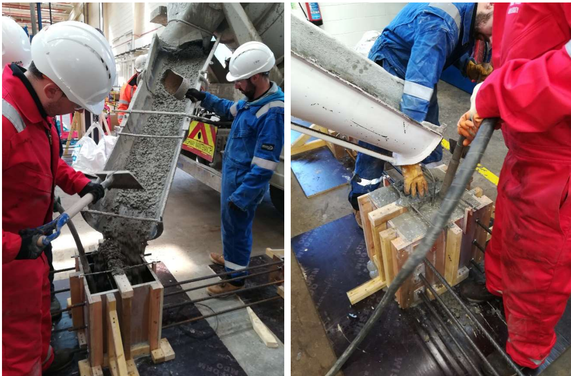
Figure 6. Concrete casting and compaction.
