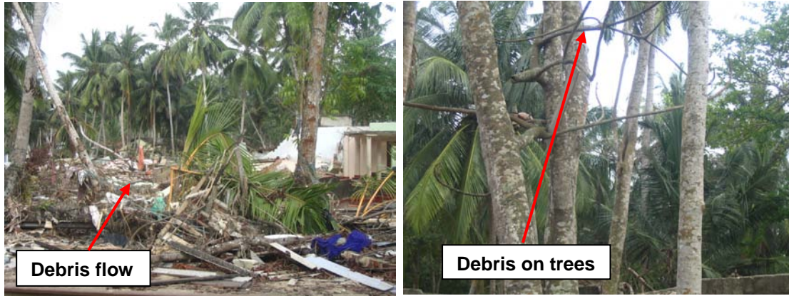
Figure 2.29: Site of debris flow at Peraliya and evidence of water level from debris on trees
