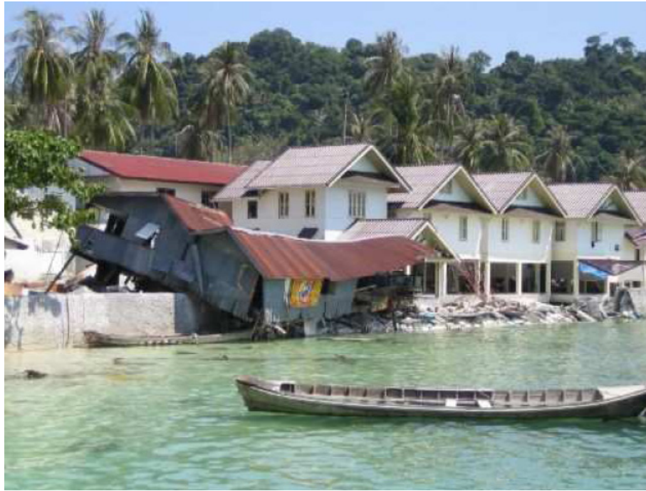
Figure 3. 17: A collapsed timber frame and corrugated iron-clad habitation on the Southeast coast of Ton Sai bay, Phi Phi Island.
