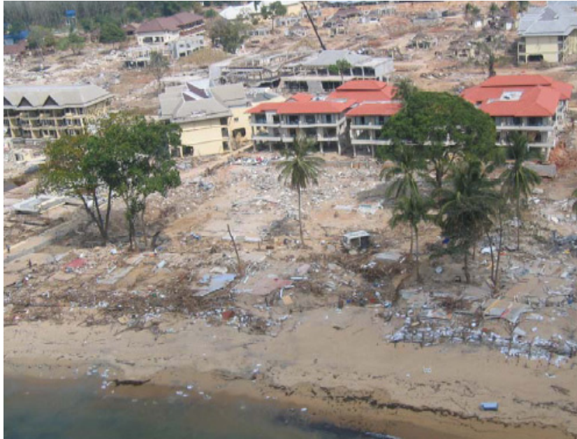
Figure 3. 49: Aerial view of tsunami damage to hotels in the Khao Lak region of Thailand, (Source: http://www.undp.org/bcpr/disred/documents/tsunami/thailand/ocha_assreport1201.pdf )
