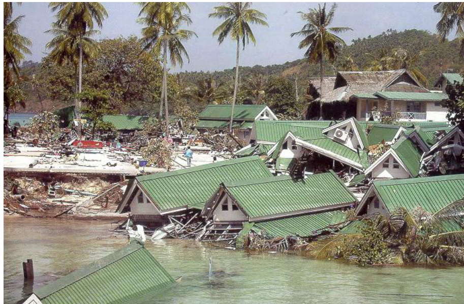
Figure 3. 21: Collapse and transport of wooden detached bungalows by tsunami waters along the south west coast of Ton Sai Bay, Phi Phi Island (Source: Warnitchai 2005).
