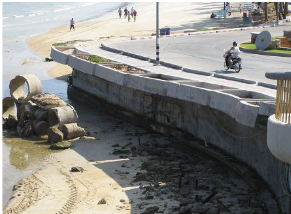
Figure 3. 46: No apparent damage on the RC retaining sea-wall at the south of Patong Beach.
