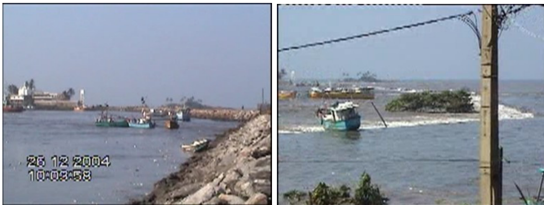
Figure 2.16: State of the Beruwala fishing harbour breakwater during the recede and after the arrival of tsunami waves (Hamza, 2005)
