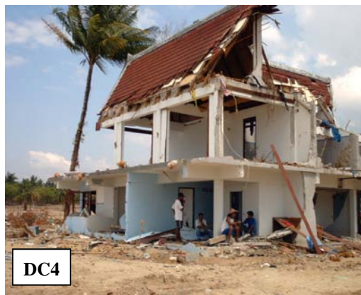
Figure 3. 32: Examples of different categories of damage DC1 to DC4 in low-rise Cat. D (left) and mid-rise (right) Cat. E reinforced concrete structures in Thailand.
