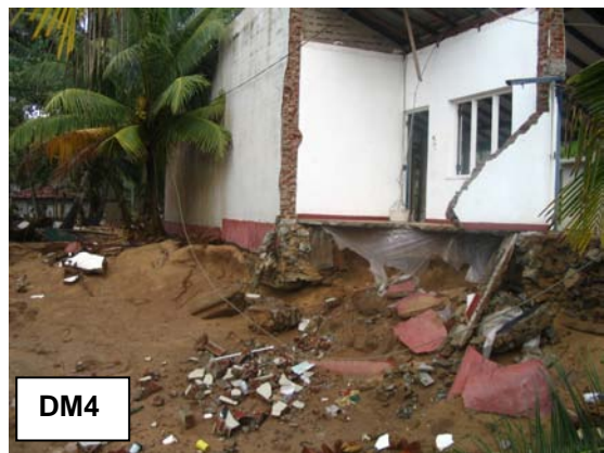
Figure 2.23: Photographs illustrating categories of damage DM1 to DM4 in unreinforced masonry structures in Sri Lanka
