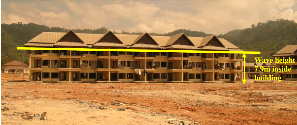
Figure 3. 15: Khao Lak Seaview Resort. Wave height was established from measurements made inside this hotel, sited approximately 150m from the beach and approximately one metre above sea level. There were only small 'bar' and pool type structures between this building and the ocean (all of which had been destroyed). Structural damage to this building was limited to windows and a few masonry infill walls, with the corner columns on the left front side also damaged presumably from debris impact.
