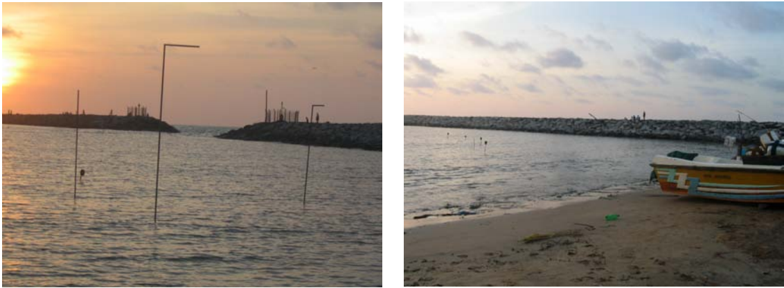
Figure 2.80: Beruwala fishing harbour with no visible damage to the breakwater
