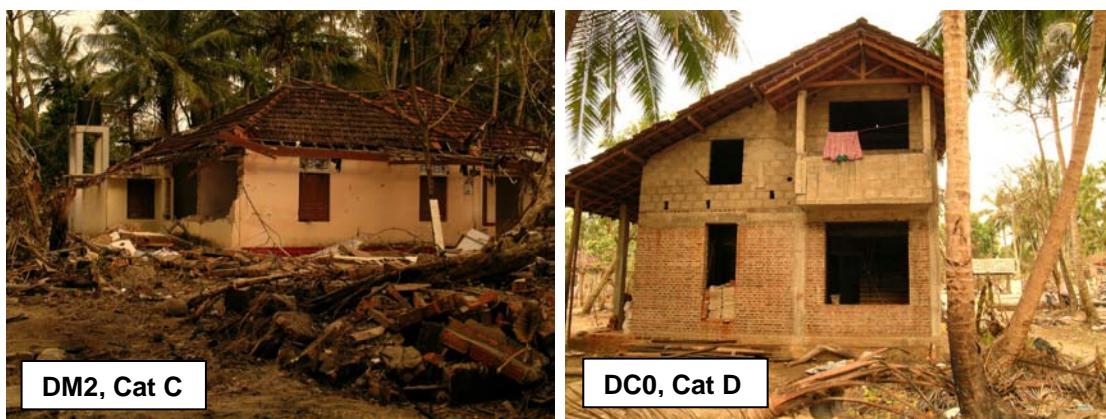
Figure 2.31: Moderately damaged Cat. C masonry house at about 400m from the coastline. Undamaged RC frame and slab structure with masonry infill panels under construction prior to the tsunami
