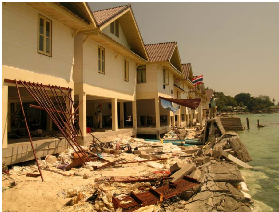
Figure 3. 18: Reinforced concrete frames with open ground stories on the south-eastern side of Ton Sai Bay, Phi Phi Island.
