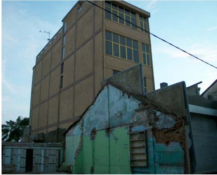
Figure 2.22: Example of mid-rise RC commercial building
