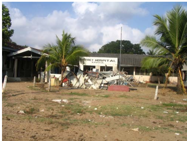
Figure 2.76: Damaged Kinniya district hospital in Trincomalee (Photo by Anton Pillai, Arup)
