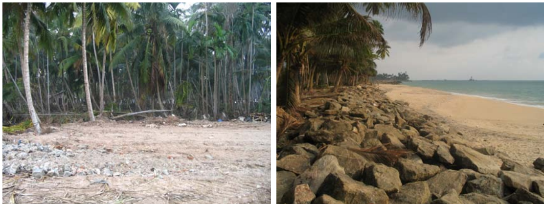
Figure 2.33: Fallen coconut trees at about 800m from the coastline suggesting significant flow velocities at this distance. Coastal protection at the coastline of Peraliya
