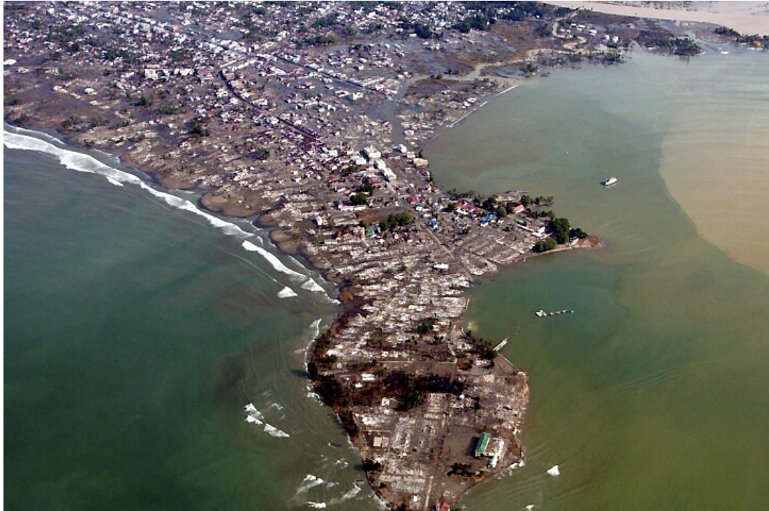
Figure 1.13: The devastating effects of the tsunami on the city of Meulaboh.
