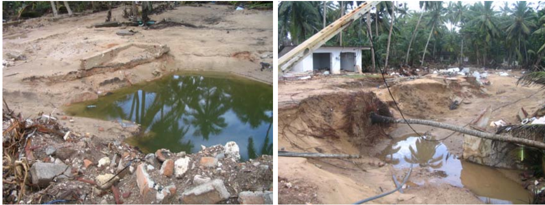
Figure 2.26: Scouring and destruction of houses in Kahawa, Sri Lanka
