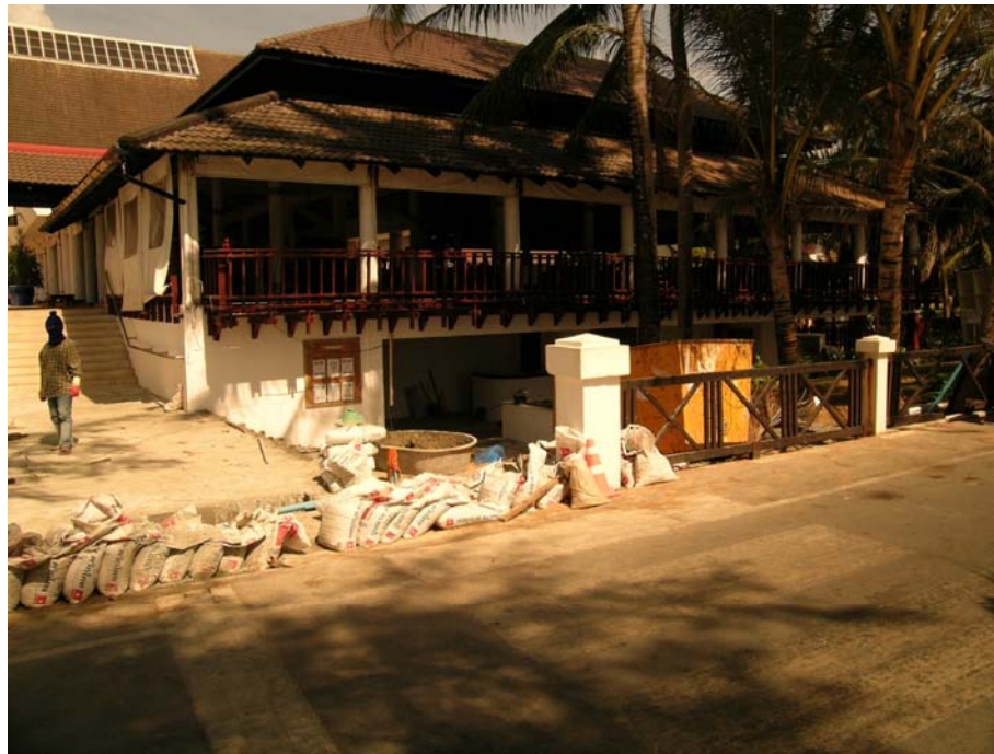
Figure 3. 2: Minor damage to Club Mediteranée Resort at Kata Beach. Damage was mainly restricted to the ground floor and was not structural in nature.
