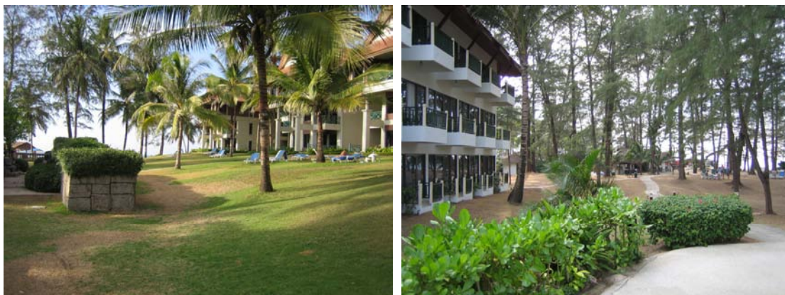
Figure 3. 10: No damage to the Laguna Beach Hotel in Bang Tao Beach (a), which was elevated 3.5m above the shore and set back 100m from the shore. (b) Damage to window curtain walls and non-structural infill panels of the three-storey Rydges Amora Beach Resort on Bang Tao Beach were repaired. These buildings are located at approximately 120m from the coastline.
