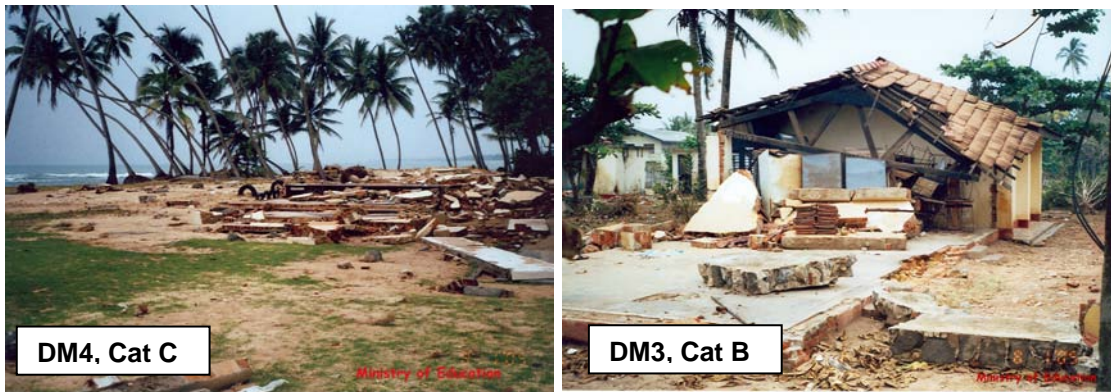
Figure 2.77: Destroyed school (Cat. C) in Akurala and heavily damaged school building (Cat. B) in Gintota (Southern Province)
