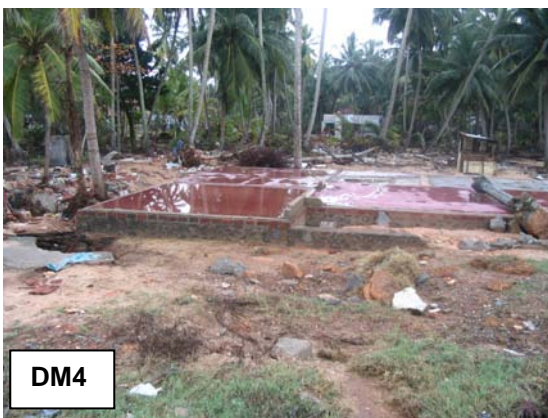
Figure 2.23: Photographs illustrating categories of damage DM1 to DM4 in unreinforced masonry structures in Sri Lanka
