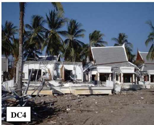
Figure 3. 32: Examples of different categories of damage DC1 to DC4 in low-rise Cat. D (left) and mid-rise (right) Cat. E reinforced concrete structures in Thailand.
