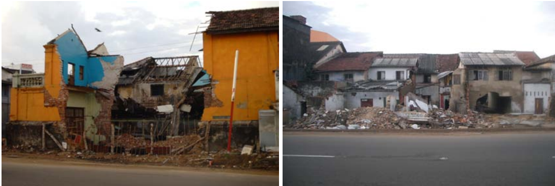
Figure 2.4: Damage to masonry houses in Galle City
