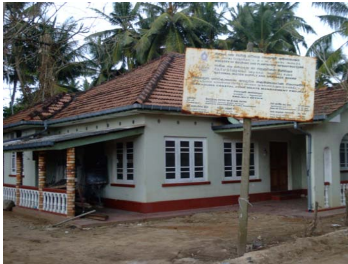
Figure 2.19: Example of the unreinforced masonry detached housing class of building
