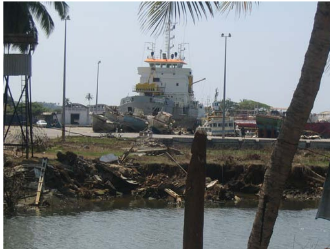
Figure 2.79: Cargo ship displaced on to the concrete quay wall at Galle Port
