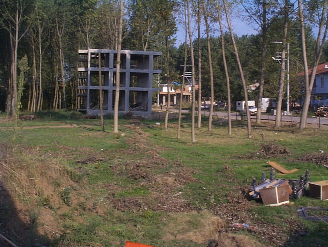
Plate 4.11 Fault rupture 'mole track' at Yuvacik passes beneath a three storey reinforced concrete frame building without causing collapse. At this location the fault was a single rupture oriented 285^\circ with a 1.6m right lateral offset (photograph taken on 18 September 1999).
