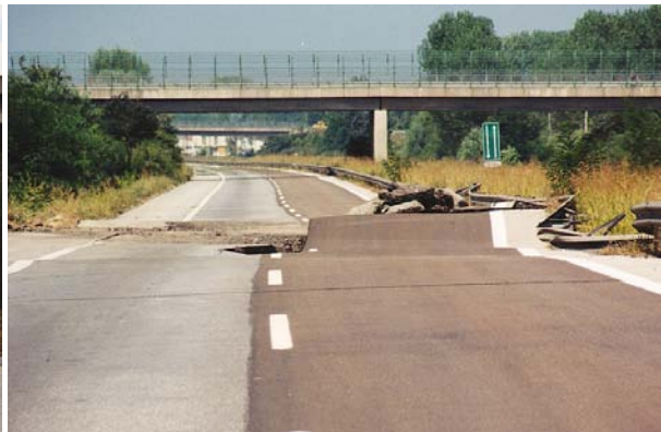
Figure 7.4: Fault rupture crossing the E80 highway (photo H.Aydin)
