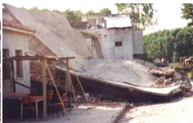
Figure 5.16b: slab damage to the same building of Figure 5.16a
