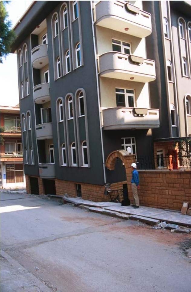
Plate 4.29 Tilting building. Note separation of 1 m between arch and its springing on corner of structure.
