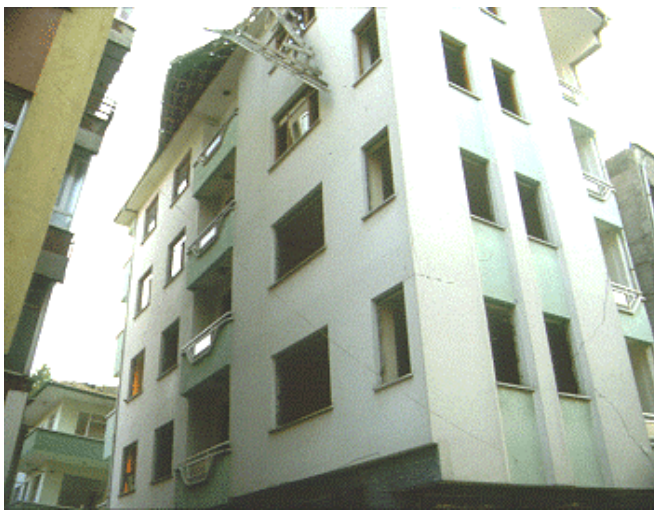
Figure 5.27a: Roof failure in a light damaged building in Adapazari
