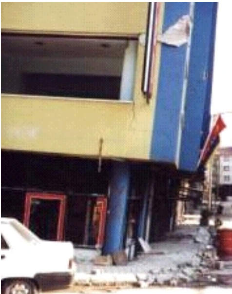
Figure 5.23a: 7 storey hotel building with raft foundation
