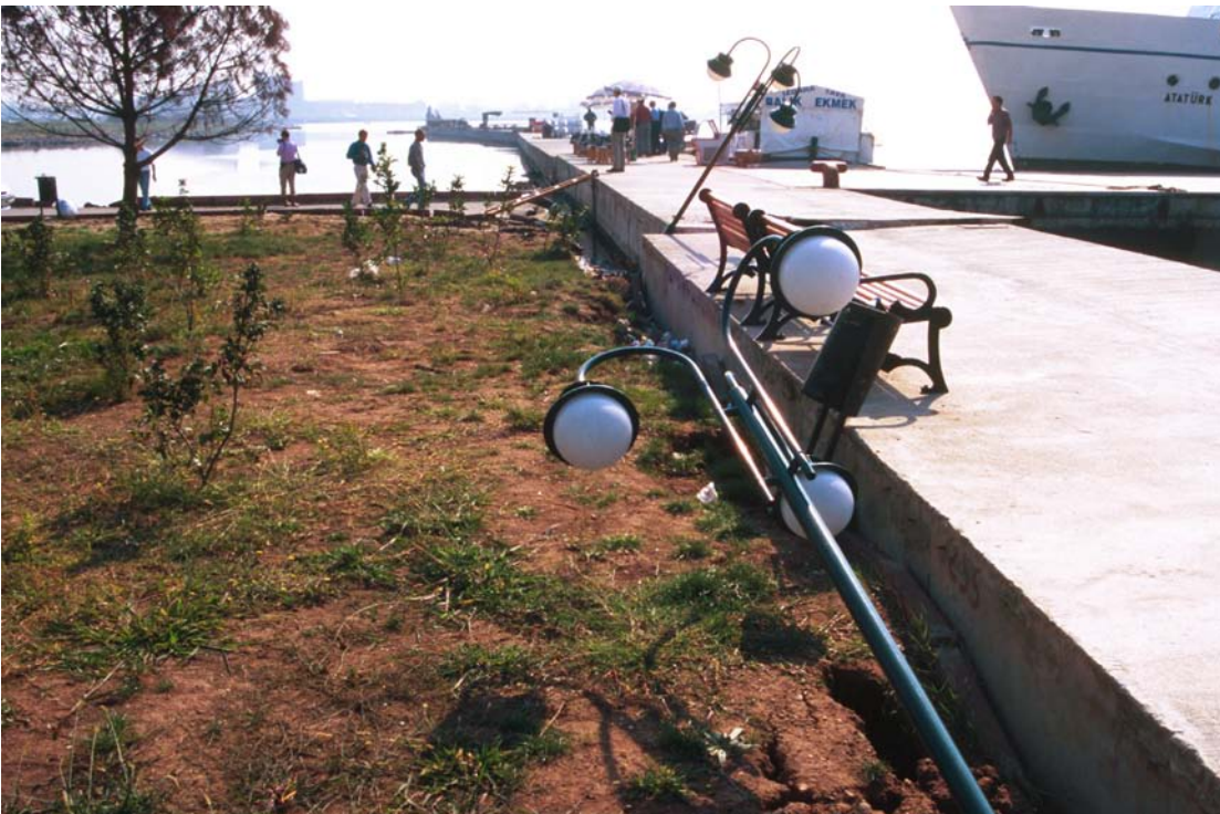
Plate 4.22 Displaced waterfront structure with settled made ground behind at Izmit Steamer Port.
