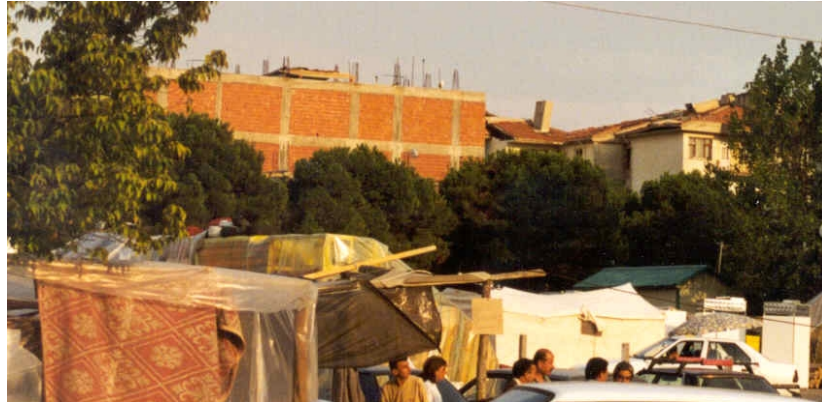
Figure 5.2: Typical r.c. frame building with protruding “waiting” bars
