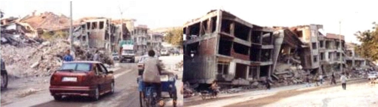
Figure 5.36a, b: Izmit Caddesi, where few buildings survived. Most of the damaged buildings were 5 stories with shops.
