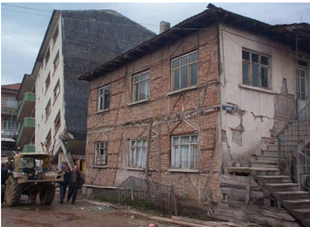
Figure 5.8: Himis timber house standing next to failed r.c. building
