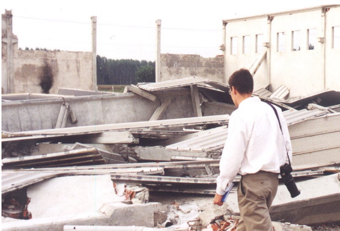
Figure 6.5a: Failure of rafters: note about 1.5m depth at apex giving a very heavy roof
