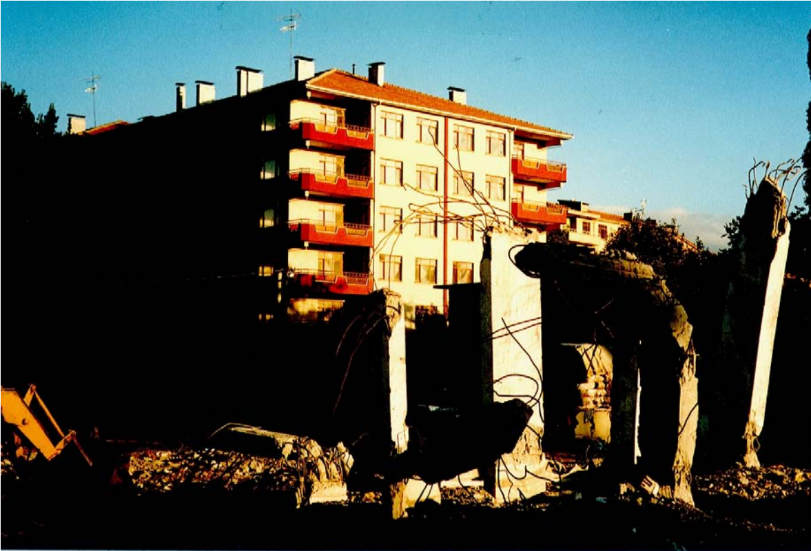
Figure 5.6: The collapsed building in Gölçük from which the sample was taken.
