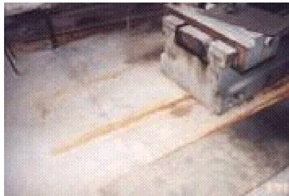
Figure 6.14c: Movement of plant inside factory near Adapazari. This 10t press moved approx 1m in the earthquake. As shown by rust marks
