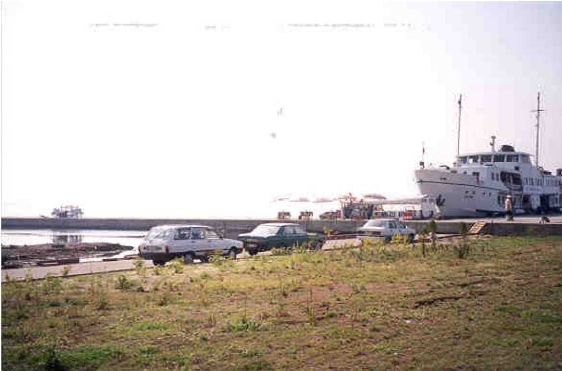
Plate 4.21 Ground settlement and low angle lateral spreading at Izmit Steamer Port. Note approximately 1m differential settlement between piled wharf structure and backfill. Also note tension cracks in foreground and slide toe uplift at centre left (photographs taken 11 September 1999).
