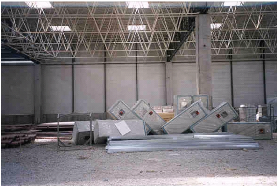
Plate 6.2: Ford Otosan Plant, Golcuk. Body Shop. Overturned electronic equipment. The plant was not operational at the time of the earthquake. Ground beams and floor slab were not complete in this area. Equipment was standing on aggregate layer. Note that columns and roof appear to be in good condition for most buildings (5 September 1999).
