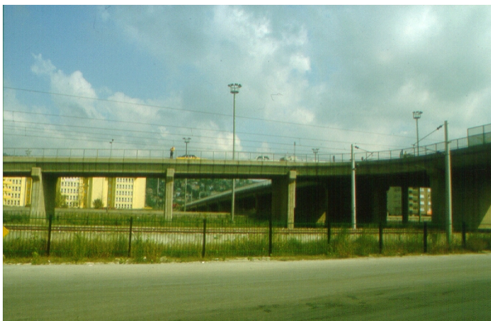
Figure 7.10: General view of viaduct in Izmit
