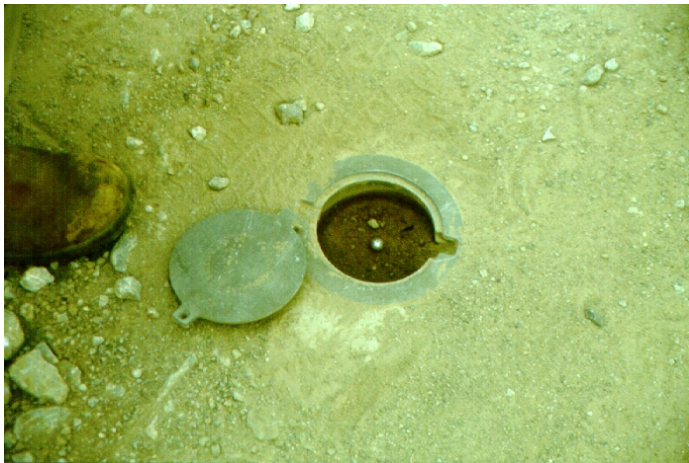
Figure 7.20 Survey Point on Yuvacik Dam Crest
