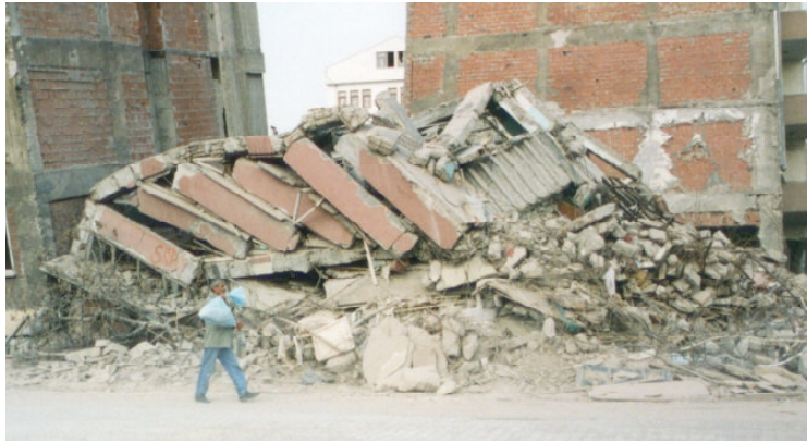
Figure 5.14b: Slender building with column oriented in the direction orthogonal to failure plane. Lack of reinforcement continuity
