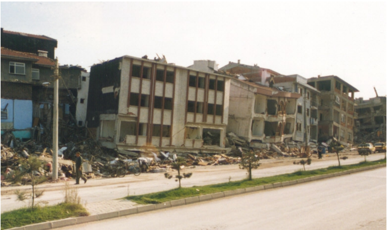
Figure 5.34b: Nato Cad. north showing numerous soft storey collapses
