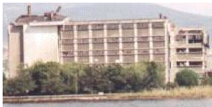
Figure 6.13c: Failure of steel frame on top of RC concrete framed building near Izmit
