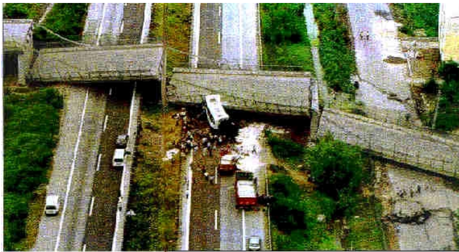
Figure 7.2: Collapse of Highway Bridge From News Footage
