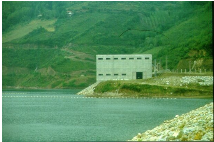
Figure 7.18: Gokce Dam: Intake Structure
