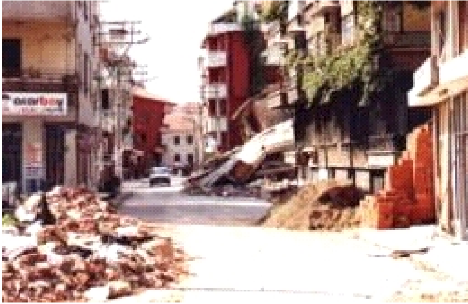
Figure 5.35: Bahcivan Sokak, showing some damage, but the majority of buildings surviving
