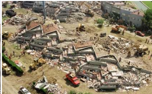
Figure 5.15b: Site with three buildings collapsed and one standing
