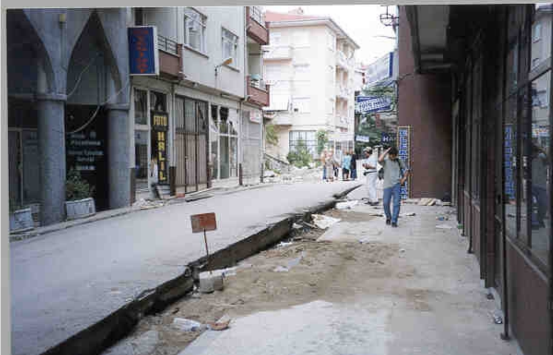
Plate 4.15 Sand venting and 300mm differential settlement of pavement in central Adapazari interpreted to be associated with liquefaction (photograph taken on 6 September 1999).
