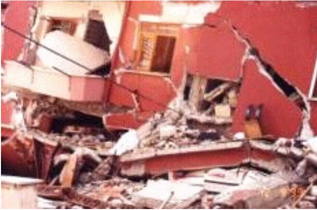
Figure 5.19 a: Lower storey collapse of a 4 storey building and failure of infill panels
