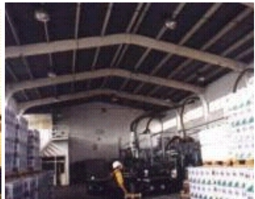
Fig 6.20b: Precast concrete warehouse - undamaged
