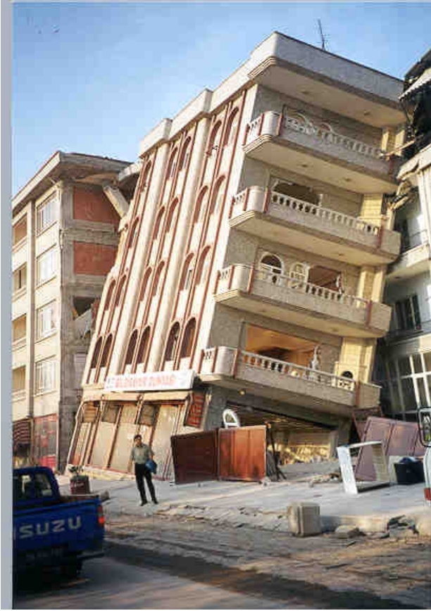
Plate 4.27 Bearing capacity failure of five storey building in Sedat Sokak in central Adapazari. Failure is interpreted to be due to liquefaction as building has settled into ground by 0.5m to 2m. Overturning has been arrested by neighbouring building (photograph taken 8 September 1999).
