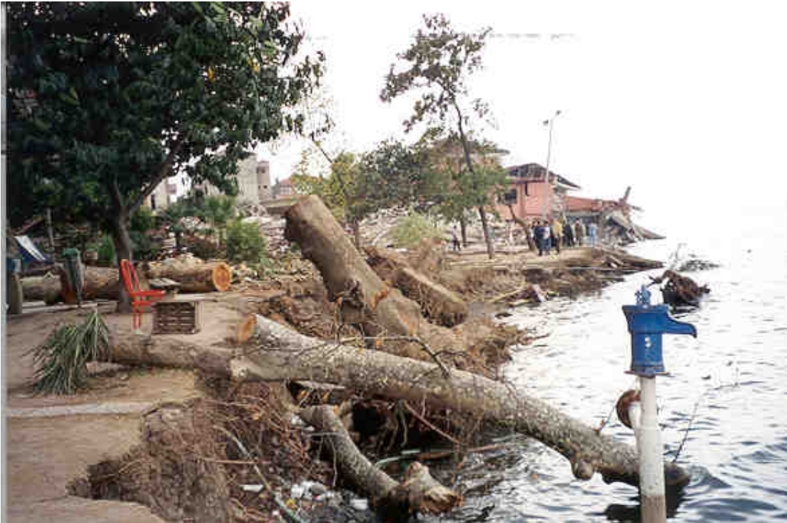
Plate 4.25 Back scarp of low angle slide or lateral spread at Degimendere. Approximately 20m of waterfront promenade is understood to have failed (photograph taken on 10 September 1999).
