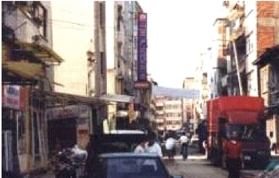
Figure 5.34a: Nato Cad. south showing relatively little damage
