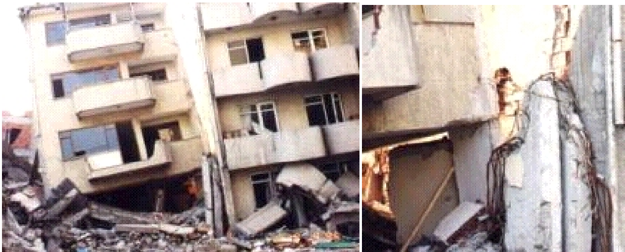
Figure 5.18a: Collapse of the lower 2 storeys
