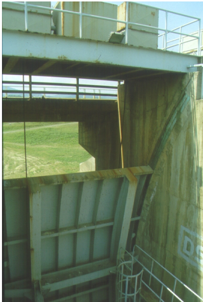
Figure 7.17: Gokce Dam: Radial Gate Structure
