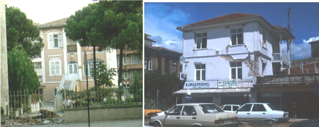
Figure 5.12: Adapazari. XIX century restored 3 storey masonry building survived undamaged in an area of numerous collapses, while another similar building suffered damage level D3, with diagonal cracks around the openings.
