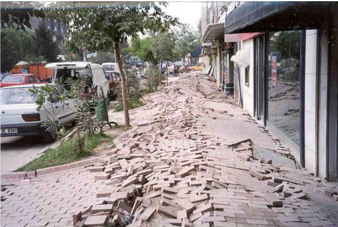
Plate 4.16 Differential settlement of pavement and buildings in central Adapazari on Pamuklar Sokak interpreted to be associated with liquefaction. Distortion of pavement may also be attributed to uplift of services due to buoyancy of buried pipes (photograph taken on 6 September 1999).
