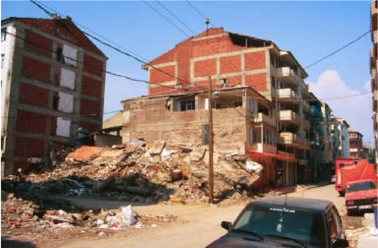
Figure 5.3: Typical medium-high density urban block in Yalova. Notice the failure of the corner building
