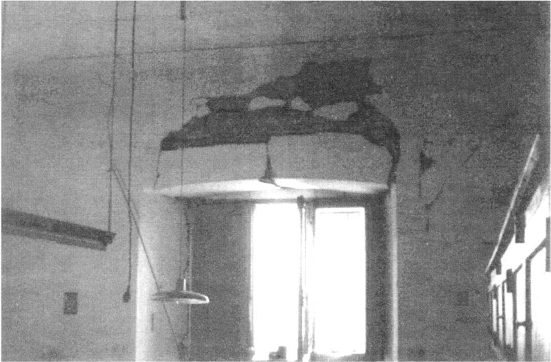
Plate 3.15: Santa Chiara Convent: the internal elevation of the south wall
