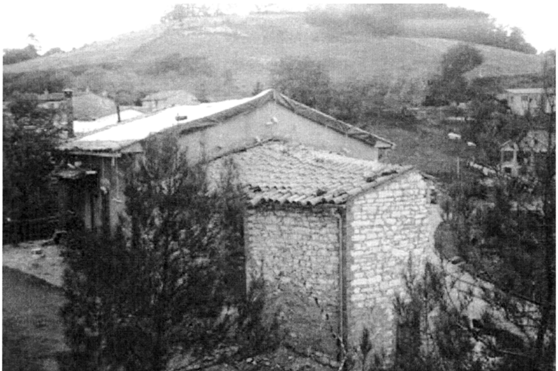
Plate 2.2: Stone masonry wall construction: example from Annifo village
