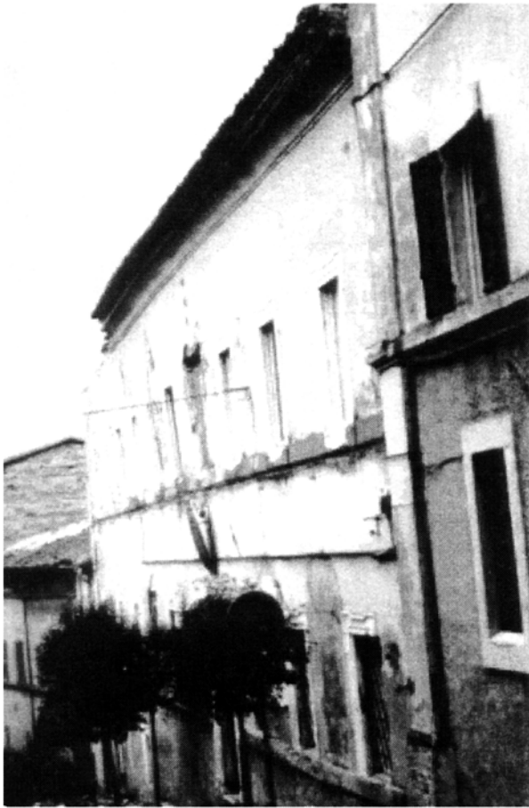
Plate 3.35: Nocera Umbra: out-of-plane overturning of the Civic Archive façade
