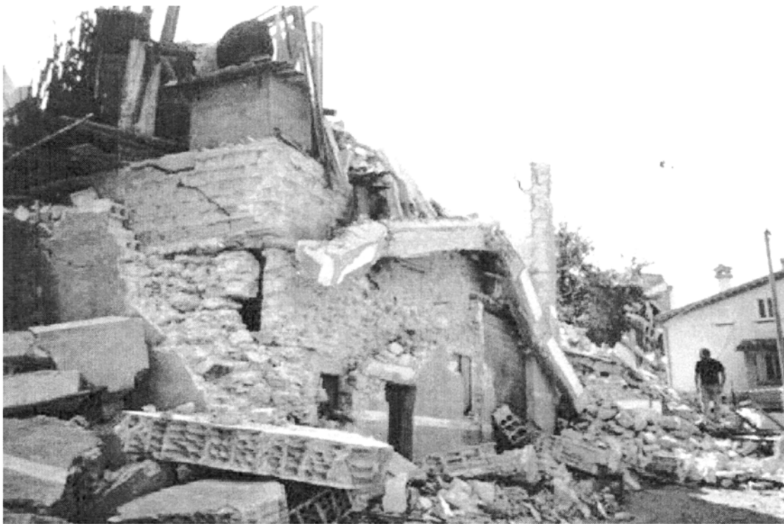
Plate 2.8: Extensions to traditional house using modern materials: Collecorti
