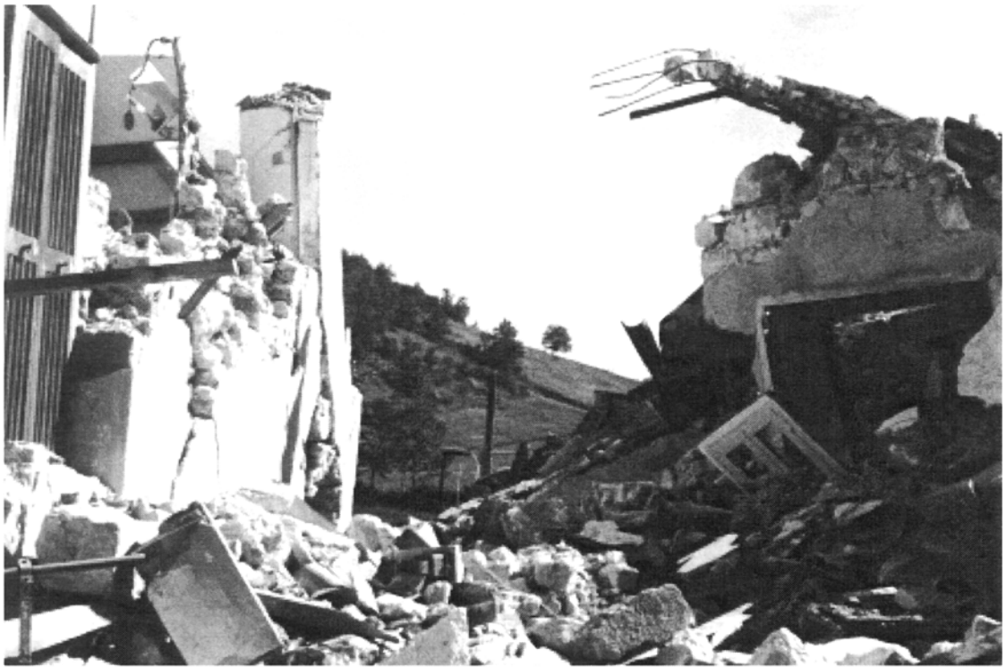
Plate 2.9: Collapsed house with inserted reinforced concrete beam: Collecorti
