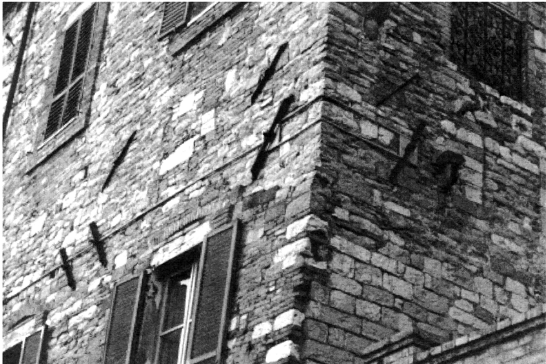
Plate 2.5: Traditional form of wall tie: Assisi
