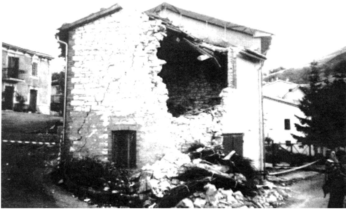
Plate 2.23: Rubble masonry building with corner damage: Annifo
