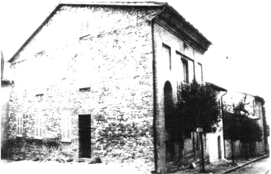
Plate 3.36: Nocera Umbra: a recently restored and improved building opposite the Civic Archive has no apparent sign of damage
