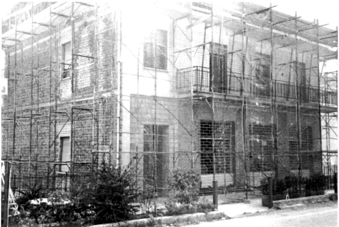
Plate 2.22: Undamaged masonry building undergoing strengthening: Nocera Scalo
