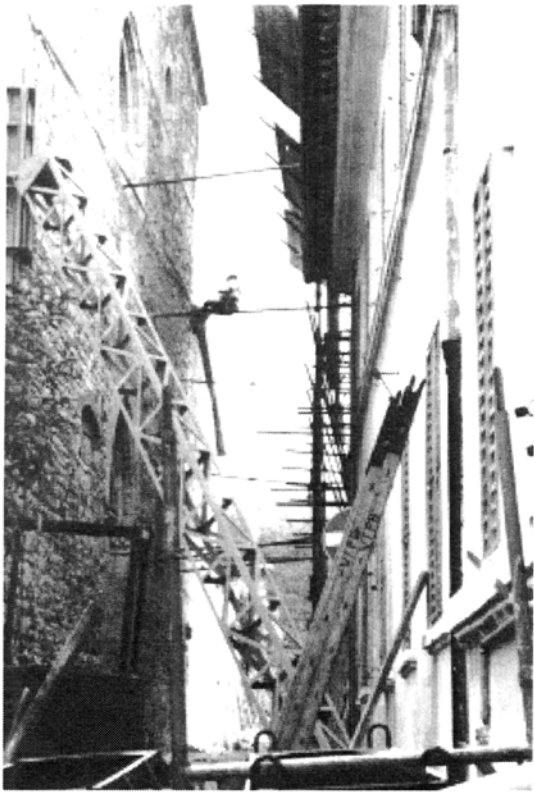
Plate 4.10: Emergency activities 10 and 11 October: strapping dangerous masonry: Nocera Umbra
