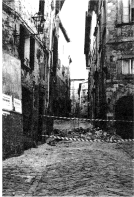
Plate 4.8: Emergency activities 10-11 October: securing dangerous areas: Nocera Umbra
