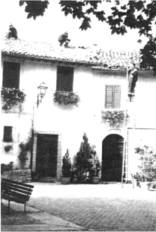
Plate 4.7: Emergency activities 10-11 October: removing loose roof materials: Nocera Umbra
