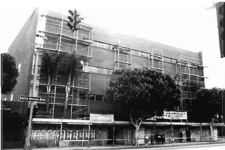
Plate 6.212: A masonry clad framed building with continuous fenestration except one end
