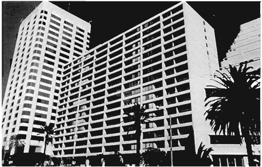
Plate 6.124: Building designed to pre-1971 edition of UBC between two buildings designed to post -1971 editions
