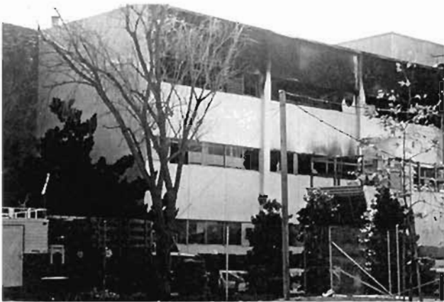
Plate 6.90: Fire damaged chemistry block
