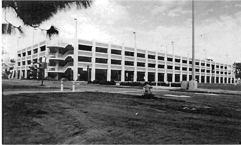
Plate 6.12: CSU Northridge : Zelzah Avenue Car Park
