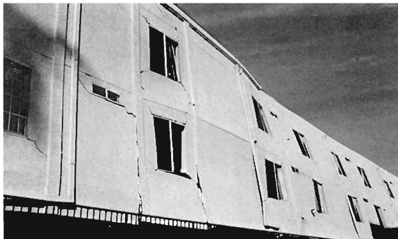
Plate 6.143: Close-up of East wall
