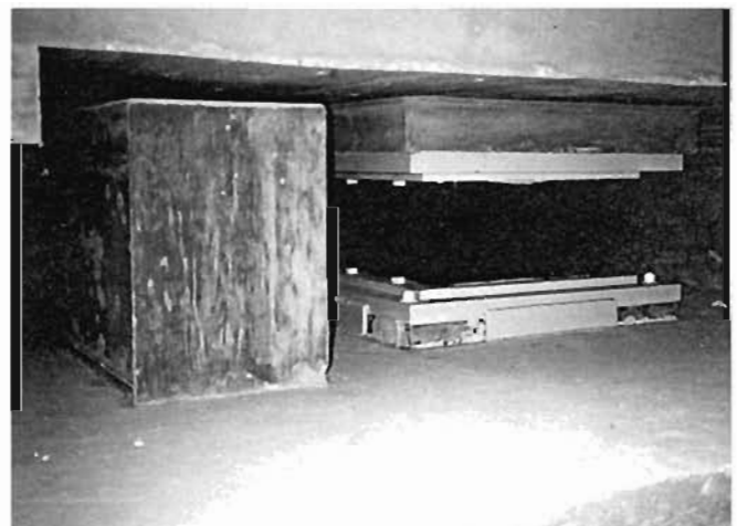
Plate 6.4: USCUTH : Bearing Location and measuring position
