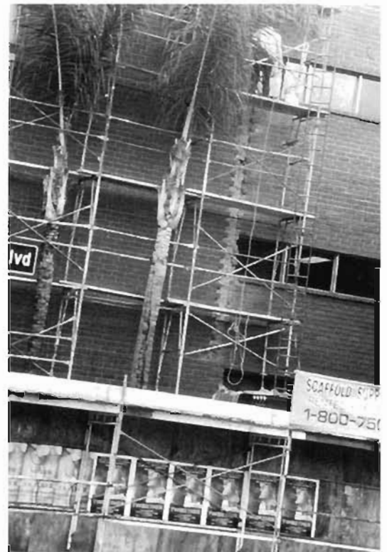
Plate 6.213: Structural damage at end of fenestration
