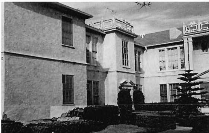
Plate 6.225: Stucco damage in old decorative U-shaped building in Santa Monica
