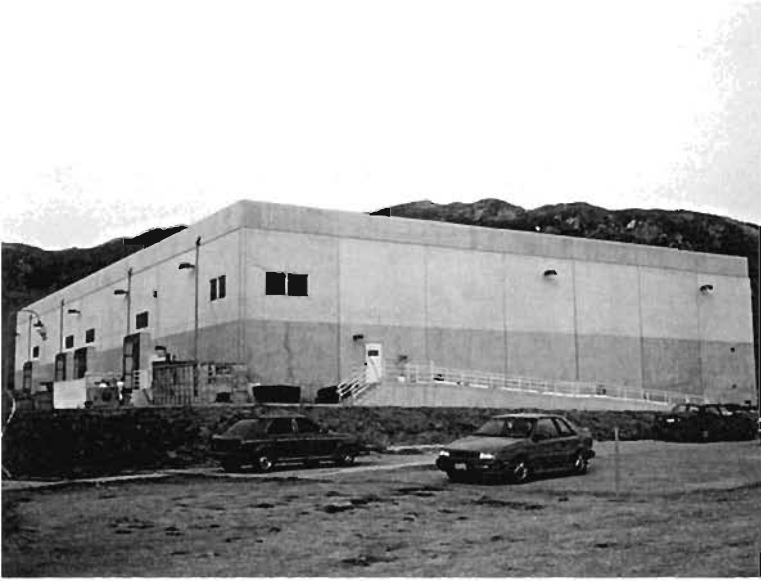
Plate 6.74: Old tilt-up in hospital grounds
