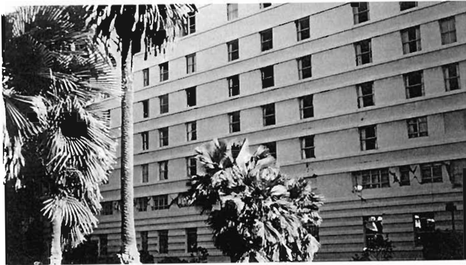
Plate 6.54: St John's Hospital, Santa Monica
