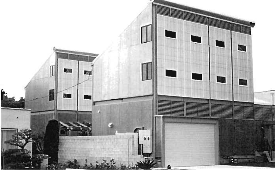
Plate 6.9: Two identical base isolated houses with braced steel frames
