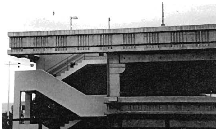
Plate 6.53: Vulnerable multi-storey car park in South LA
