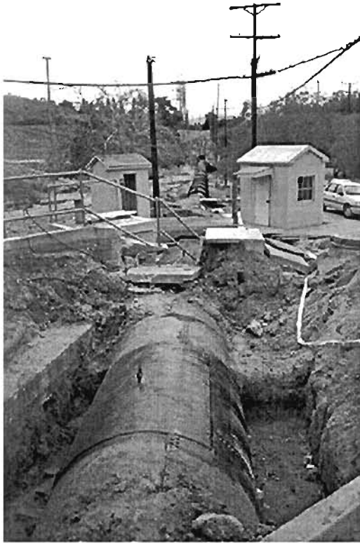
Plate 4.5: Los Angeles Reservoir Repaired outlet pipe
