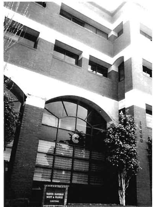
Plate 6.215: Undamaged masonry clad building with vertical irregularity
