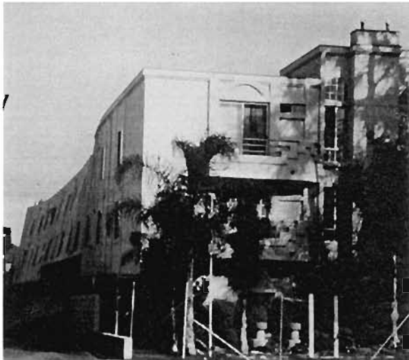
Plates 6.141/142: Triad Apartments: Inwards list of East and West walls after internal collapse
