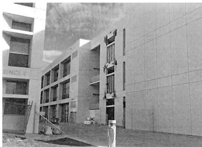
Plate 6.88: Science block showing bridge supports
