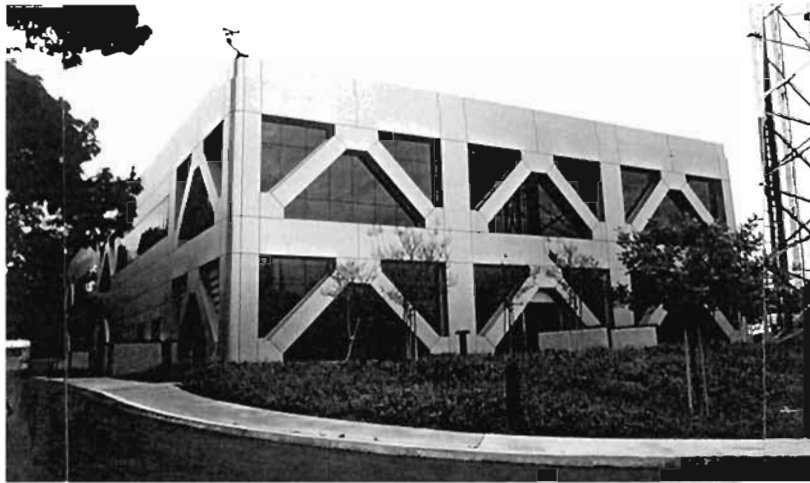
Plate 6.1: Los Angeles Fire Command and Control Facility
