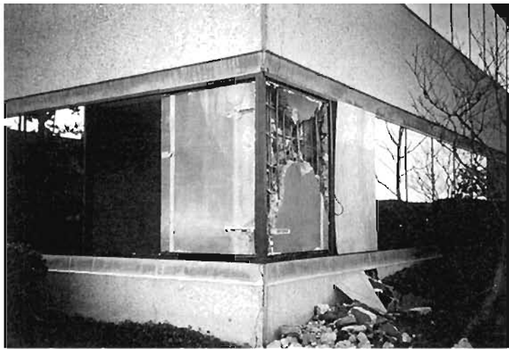
Plate 6.144: Collapsed wall of 2-storey tilt-up
