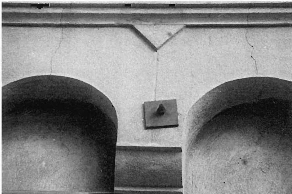
Plate 6.191: Anchor plate of tie
