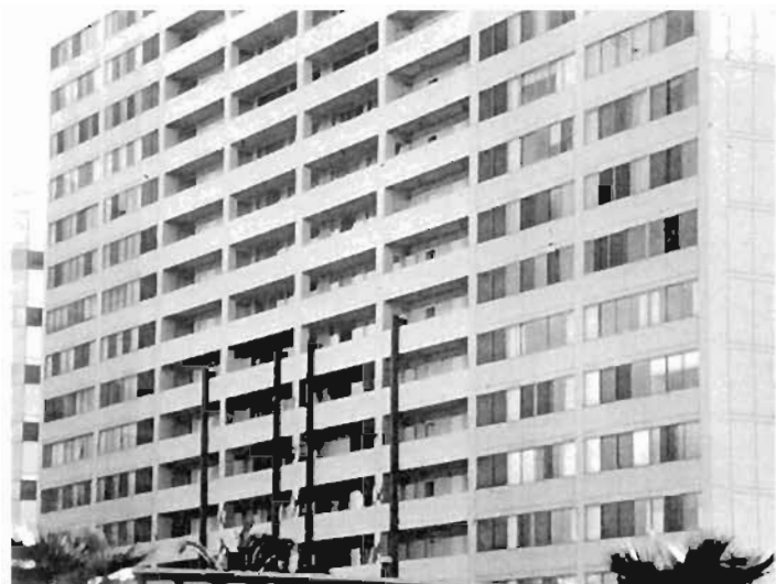
Plate 6.129: East face of Champagne Towers, Santa Monica
