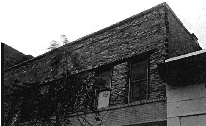
Plate 6.207: 9" wall retrofitted with flats above windows
