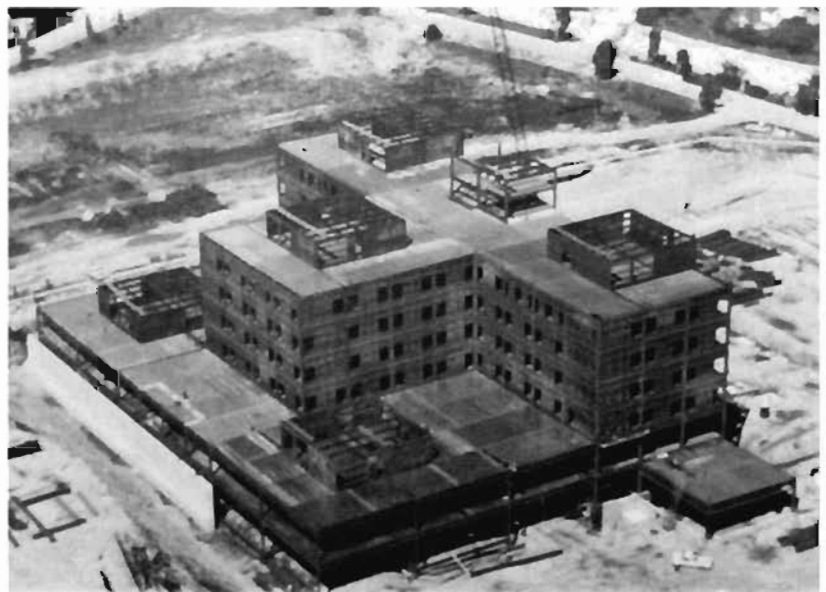
Plate 6.73: The steel plate walls during construction
