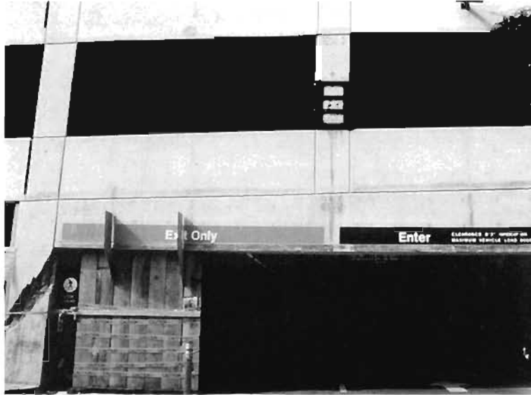
Plate 6.27: Extreme vertical irregularity at entrance
