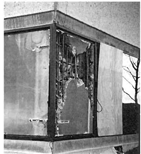
Plates 6.146/148: Failed shear panels over height of ground floor fenestration
