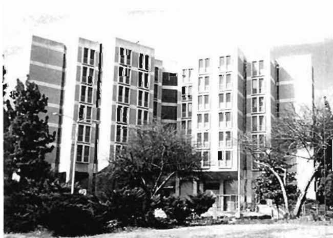
Plate 6.94: Abandoned accommodation block
