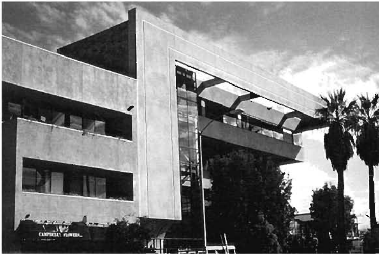
Plate 6.219: Undamaged building irregular in both plan and elevation
