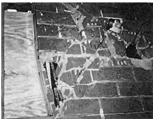
Plates 6.186/187: Buckling of unrestrained vertical bars between windows
