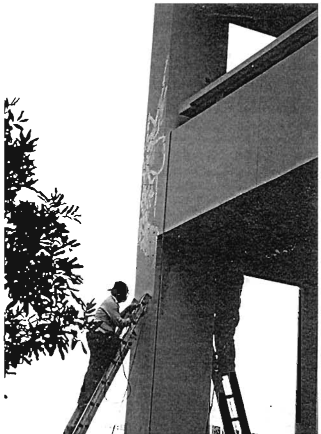
Plate 6.114: Repairing the cracks
