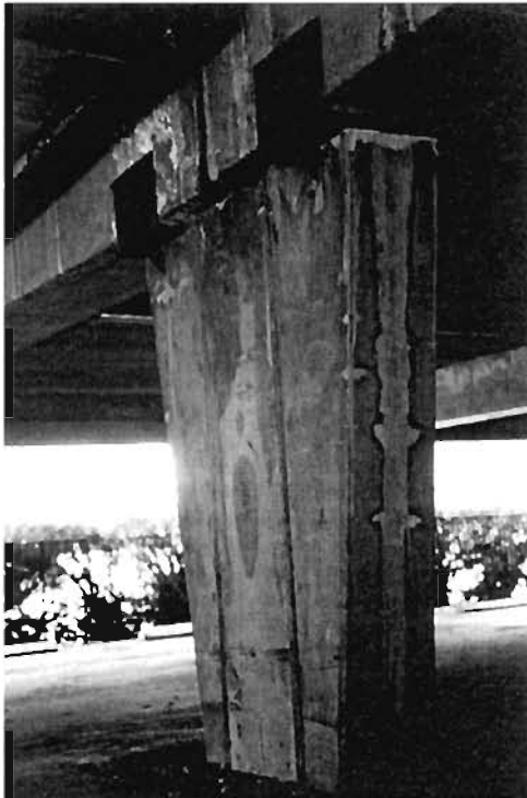
Plate 6.33: Internal columns sandwiched between replacements
