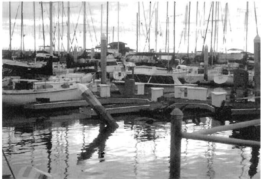
Plate 3.11: Bent concrete anchor pillars indicate direction of soil flow following liquefaction
