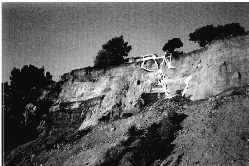
Plate 3.3: Northern end of land slide on Pacific front; plate shows wetting of soil, possibly due to a broken water main
