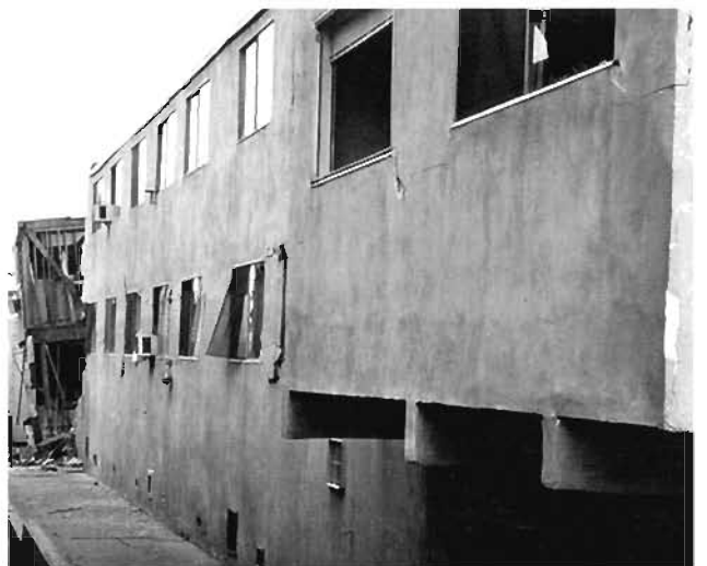
Plate 6 160: Streetwise movement of building in plate 6.158
