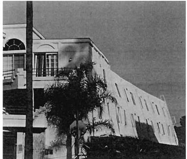
Plates 6.141/142: Triad Apartments: Inwards list of East and West walls after internal collapse
