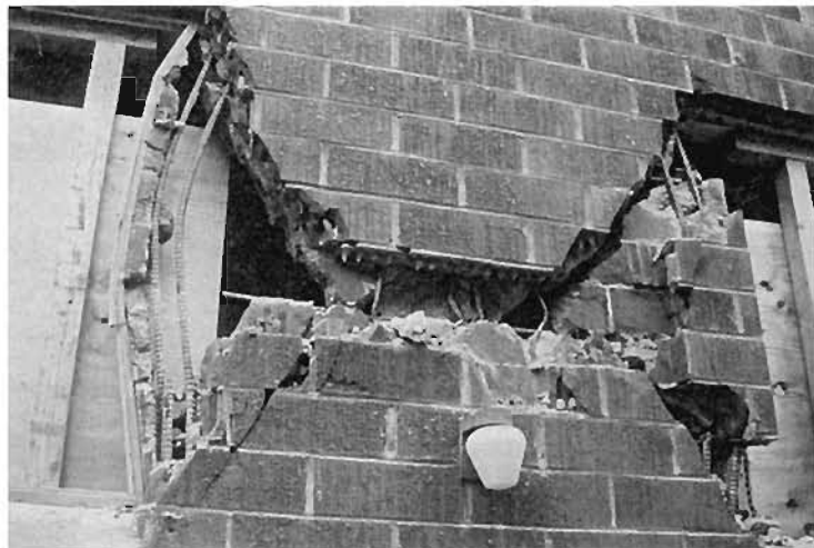
Plate 6.188: Comparable buckling at wall ends
