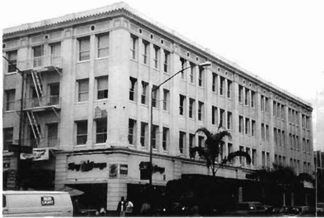
Plate 6.208: A discretely retrofitted masonry clad building with shop fronts
