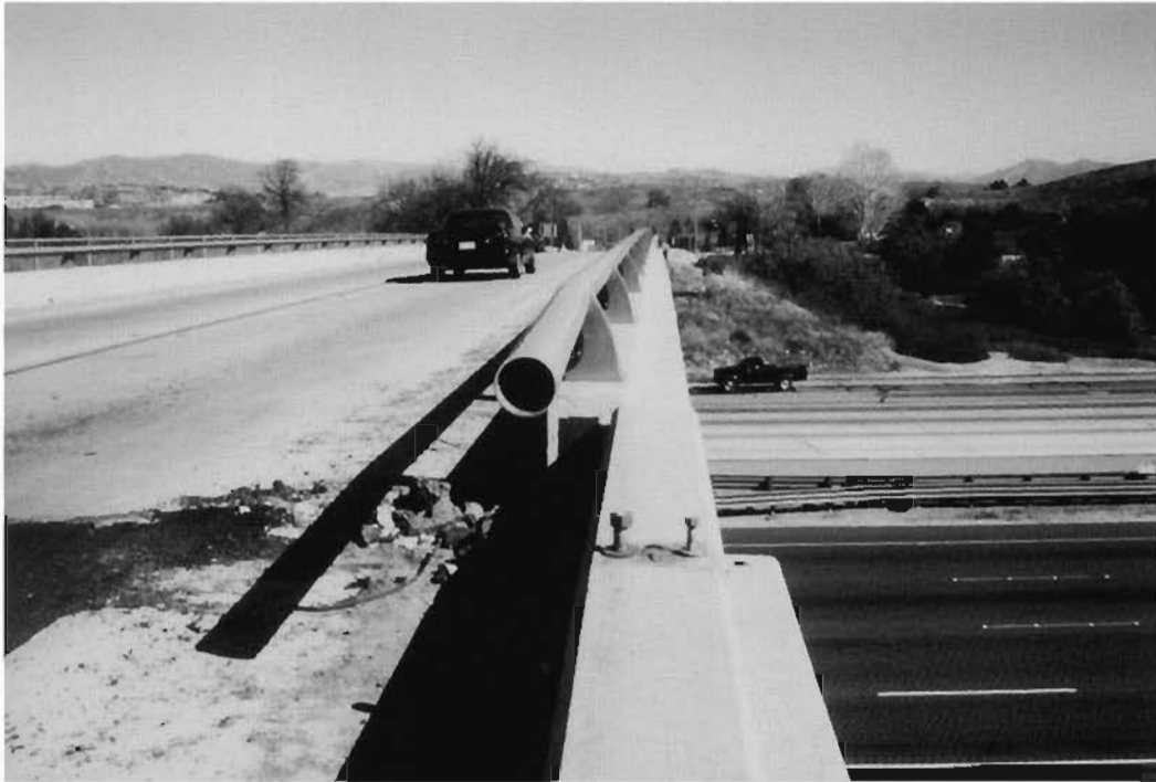
Plate 5.14: Lateral movement of composite bridge over Interstate 5
