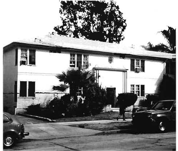
Plate 6.156: Stucco fallen from plywood sheet
