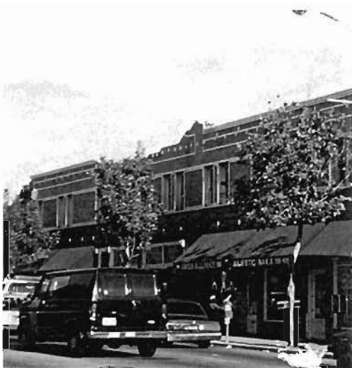
Plate 6.196: Partial collapse of retrofitted parapet
