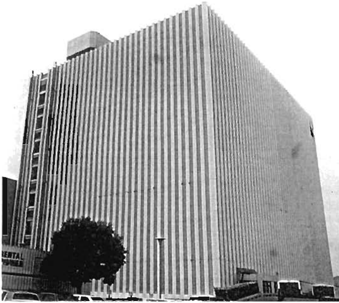
Plate 6.111: Extensive wall cracking in AT&T building
