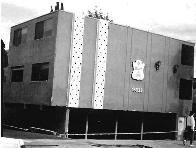
Plate 6 159: Ground floor weak storey accommodating car ports
