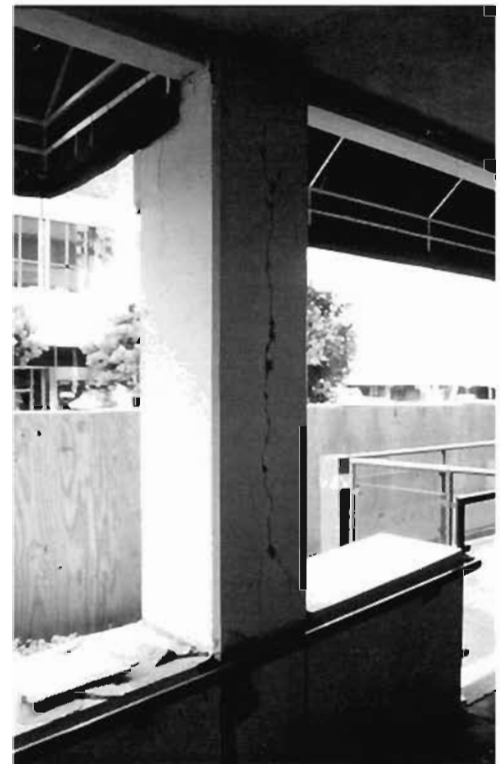
Plate 6.122: Vertical splitting of column
