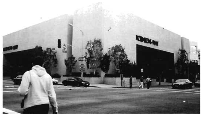
Plate 6.218: Undamaged building with extreme vertical irregularity
