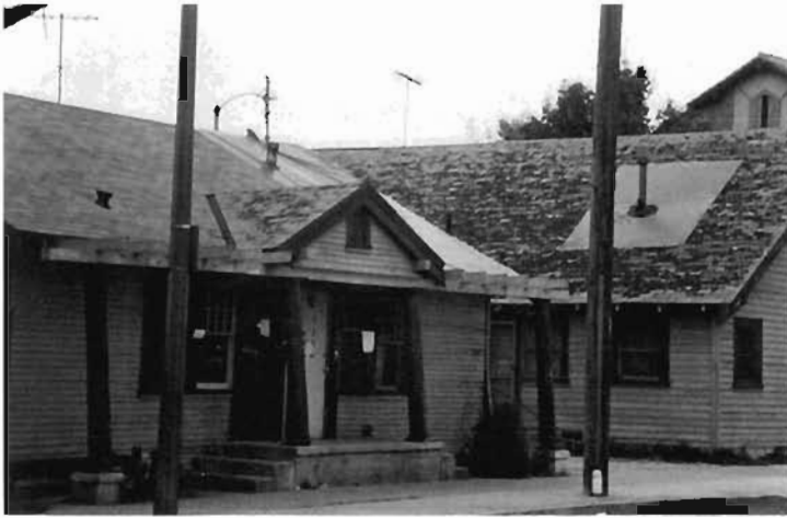
Plate 6.149: Collapsed chimneys
