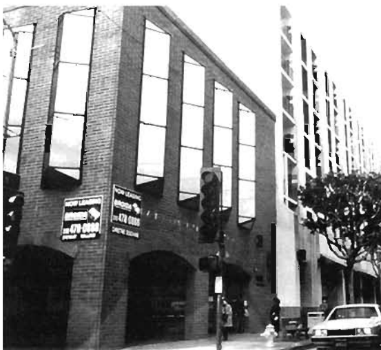
Plate 6.214: Undamaged building with extreme vertical irregularity
