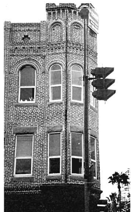
Plate 6.202: Retrofitting and separation at corner
