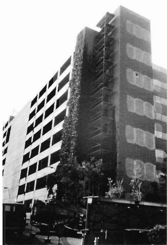
Plate 6.29: Separated stair well
