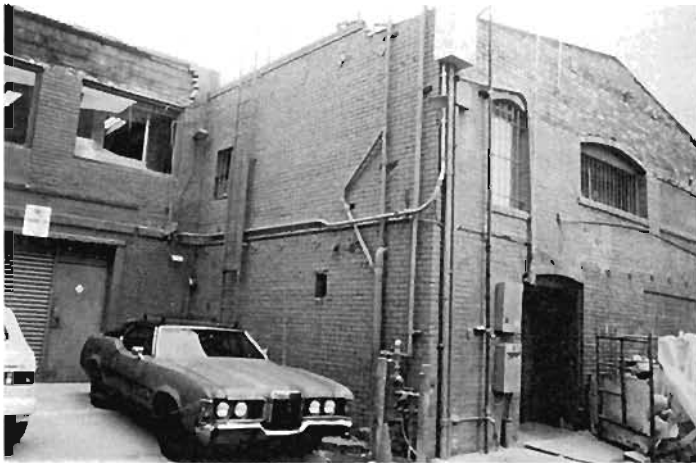
Plate 6.206: 9" wall retrofitted with ties
