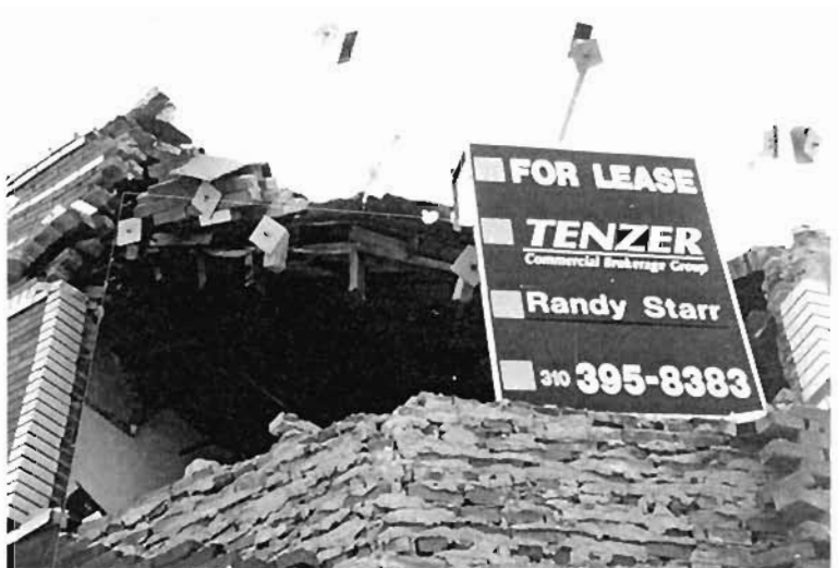
Plate 6.197: Parapet/upper wall failure at rounded corner
