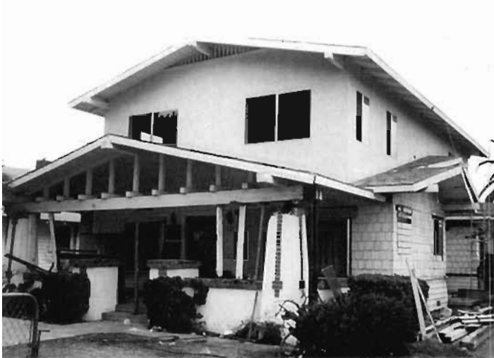
Plate 6.151: Collapsing porch
