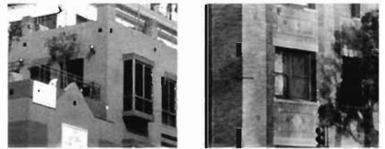
Plate 6.210: Close-ups of retrofitting
