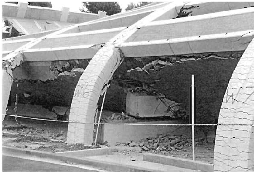
Plate 6.20: Distributed out-of-plane inelasticity in columns
