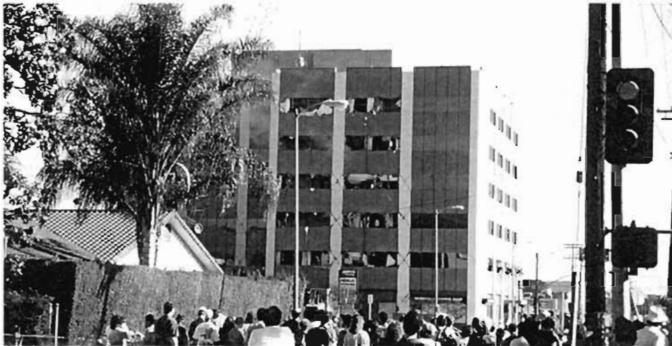
Plate 6.58: Barrington Medical Centre, Santa Monica
