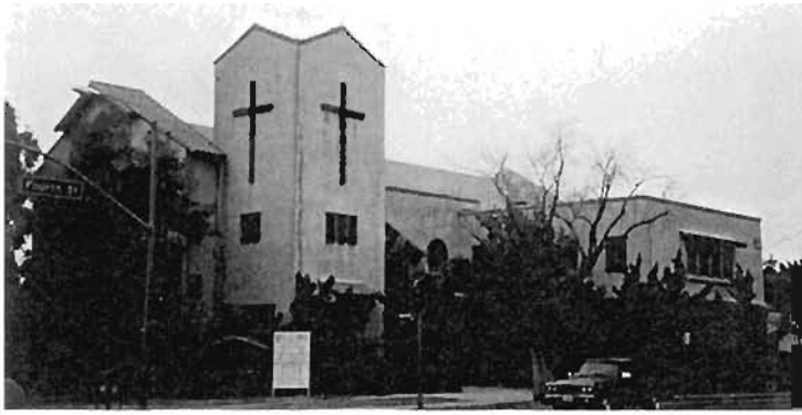
Plate 6.220: Church of light construction in San Fernando
