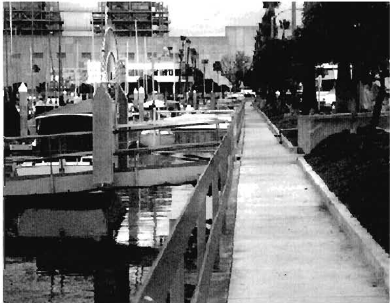
Plate 3.8: Quay wall at the King Harbour before the earthquake
