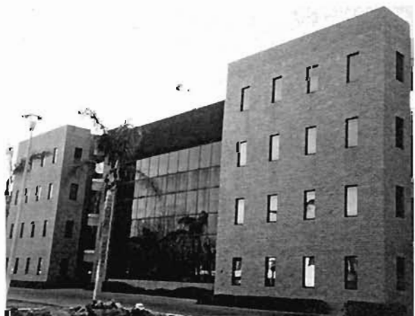
Plate 6.95: Undamaged faculty office
