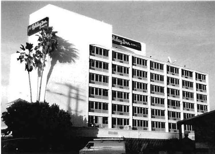
Plate 6.97: South side (rear)
