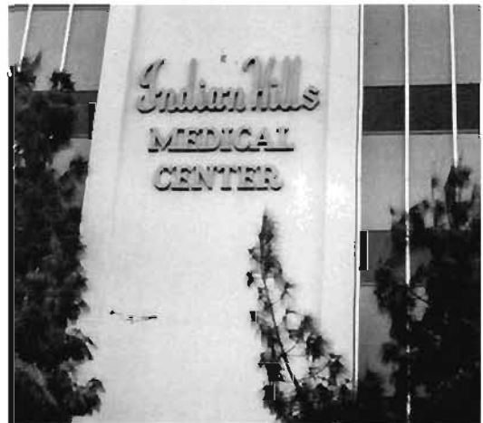
Plate 6.68: Side wall damage on opposite face
