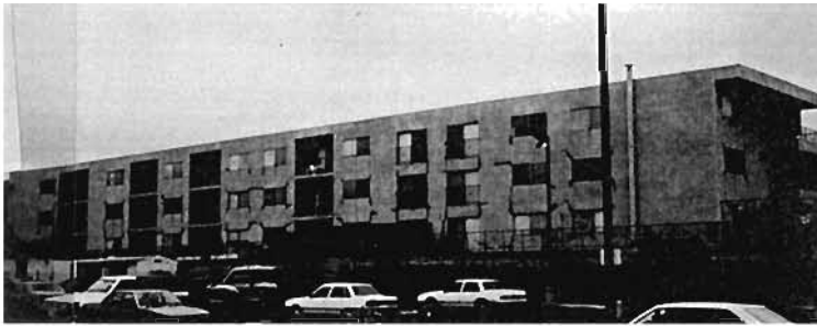
Plate 6.222: Long low apartments with rigid walls bolt end in Santa Monica
