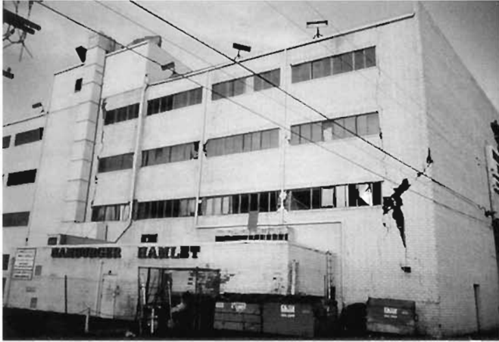
Plate 6.179: Reinforced masonry building
