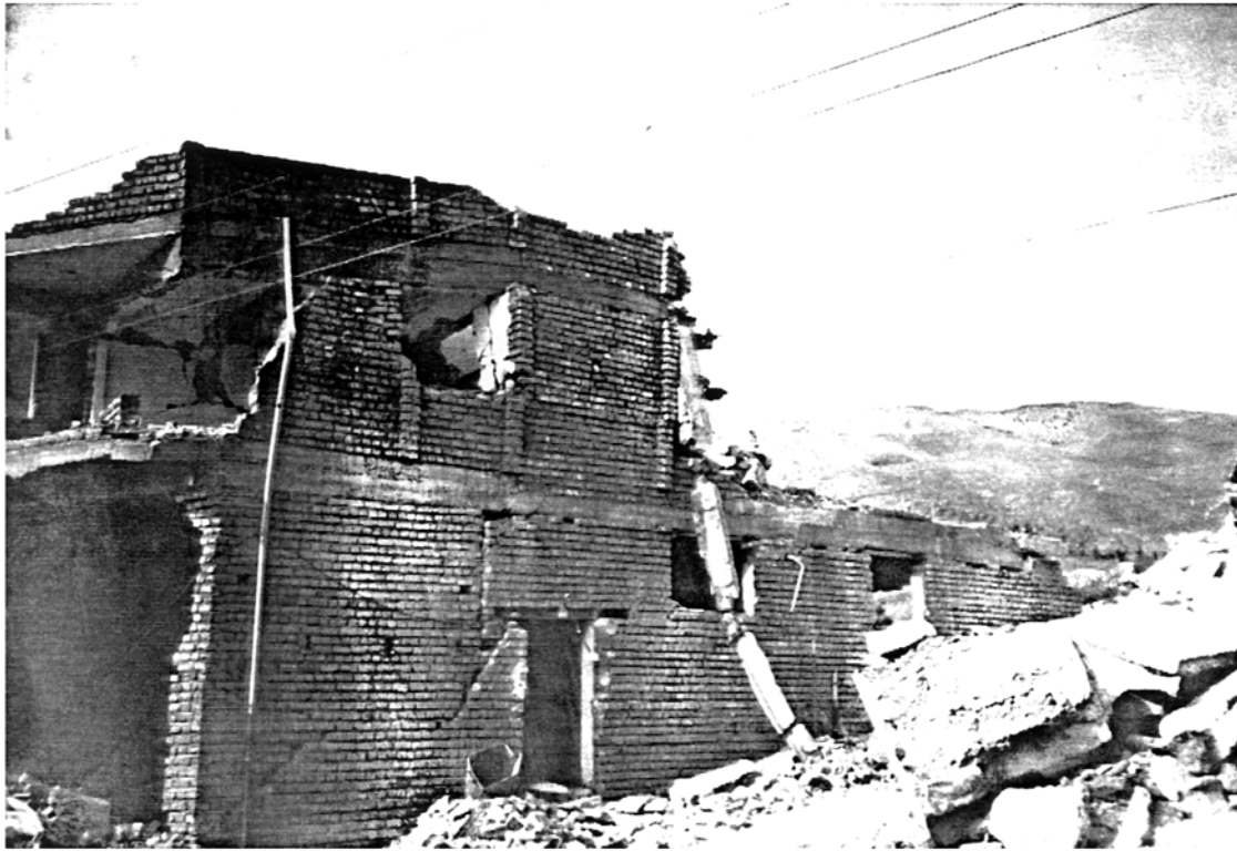
Picture 3.11 Two-storey Brick Building, Manjil Collapse of the ring beam and roof of the east side due to the complete loss of vertical support
