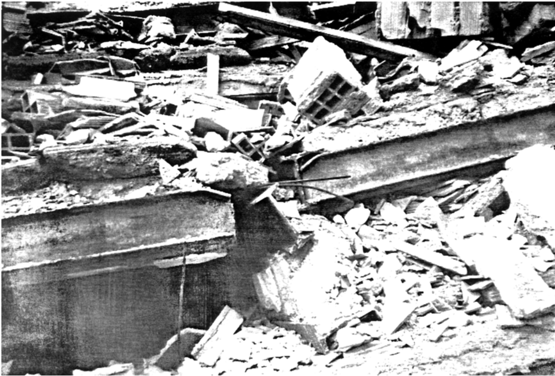
Picture 4.25 Six-storey Steel Frame Building, Rasht Weak welded joints simply snapped under small stresses
