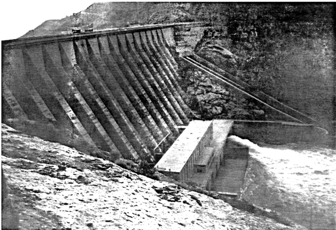
Picture 5.2 Sefid-rud Dam, Manjil, general view of downstream
