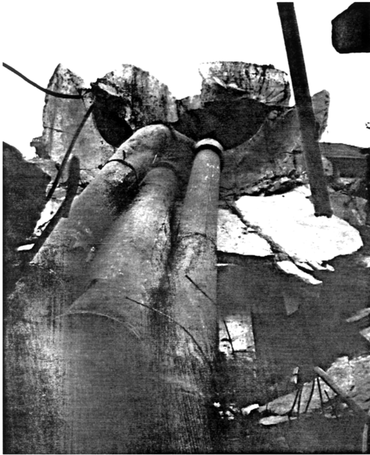
Picture 5.29 Concrete Water Tower No. 1, Rasht Destruction of the shaft on impact
