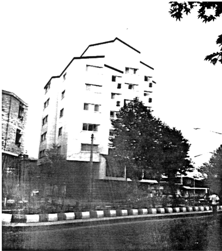
Picture 4.33 Nine-storey Apartment Block, Rasht The concrete frame behaved well
