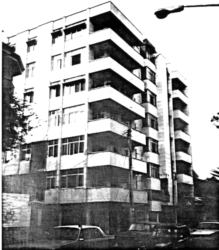
Picture 4.27 Seven-storey White Stone Clad Building, Rasht A steel frame building with better design and workmanship
