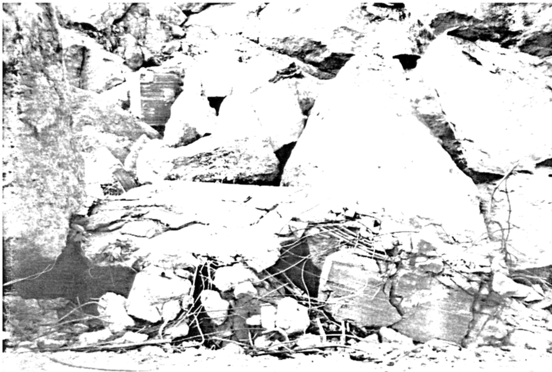
Picture 5.10 Sefid-rud Dam, Manjil Destruction of the reinforced concrete guard house under the secondary action of the rock fall
