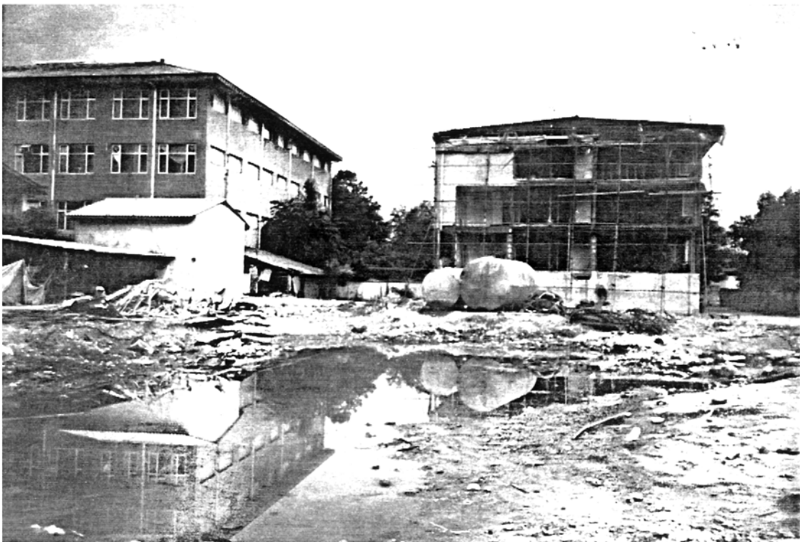
Picture 4.26 Site of a collapsed eight-storey steel frame building. Poor welded joints and weak steel columns the main causes of failure, Rasht
