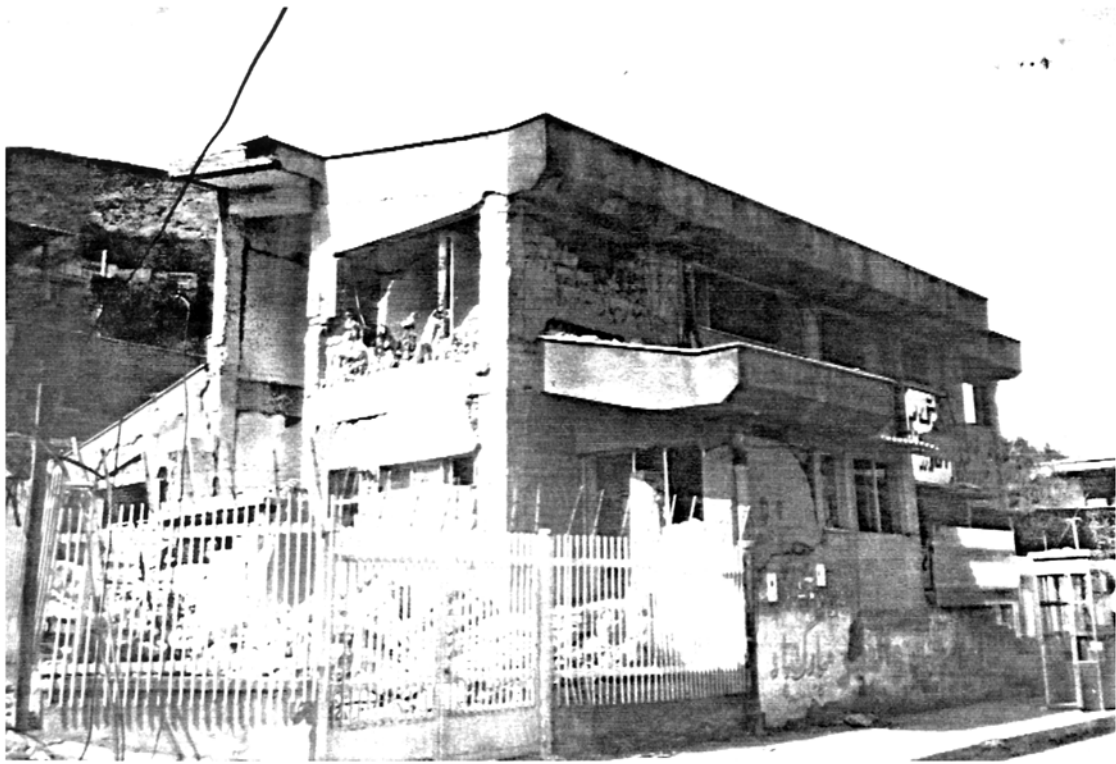
Picture 4.13 Telecom Building, Rudbar Collapse of the infill masonry walls
