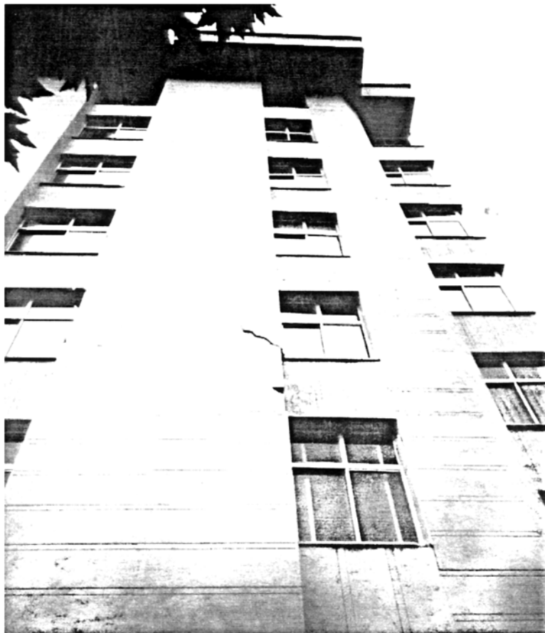
Picture 4.36 Eight-storey White Stone Clad Building, Rasht Minor crack in the stone cladding the only damage in this building
