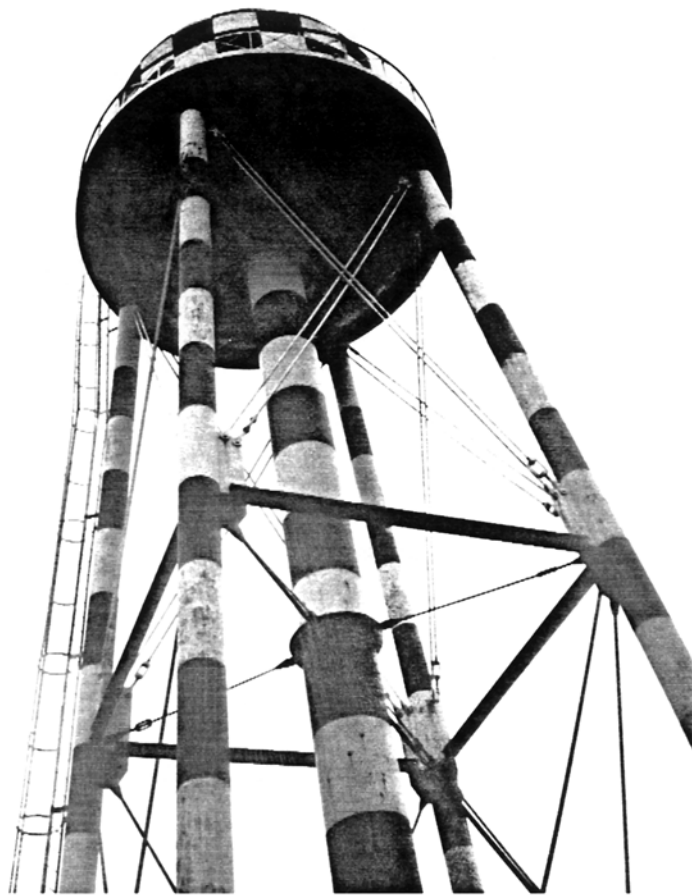
Picture 5.35 Elevated Steel Water Tank, Rasht No damage to this well supported elevated water tank
