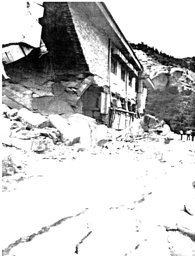
Picture 3.10 Vali-asr Hospital, Rudbar Failure of built ground and the pavement concrete slabs
