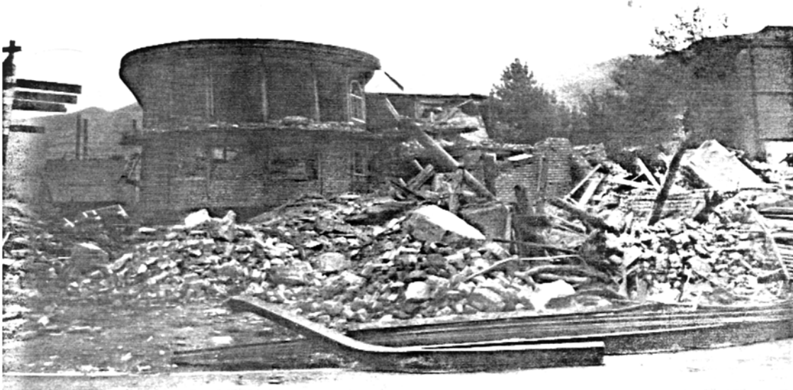
Picture 3.24 Two-storey Steel Frame Building, Rudbar Bending failure in upper floor due to lack of shear elements
