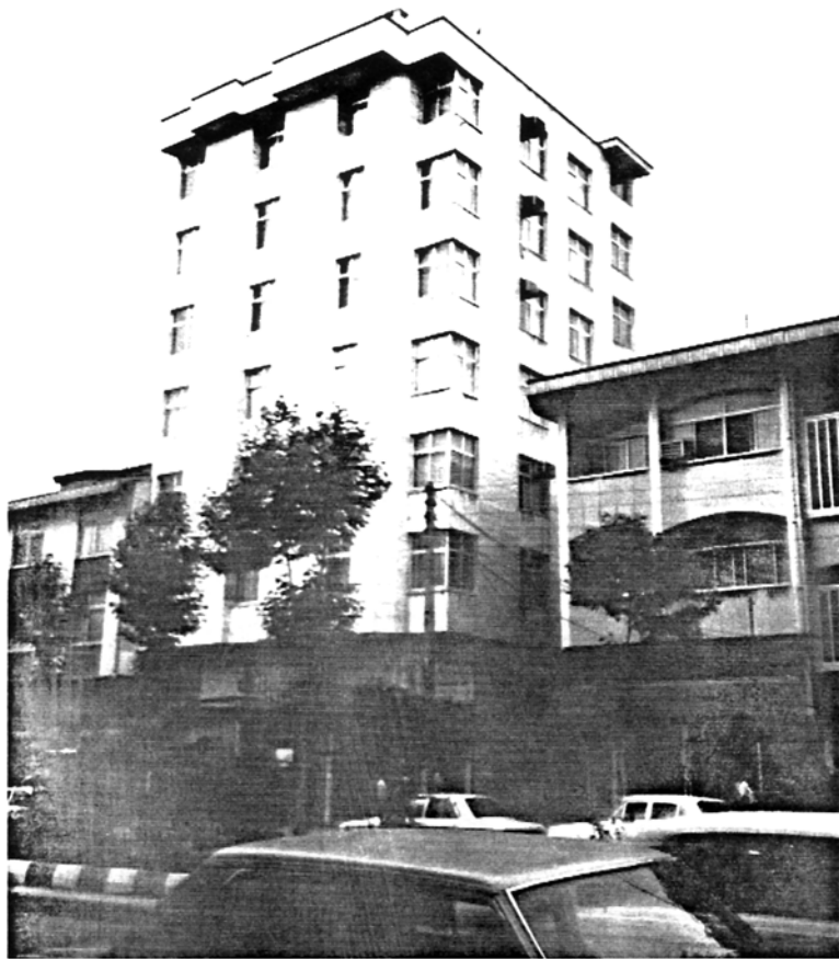
Picture 4.35 Eight-storey White Stone Clad Building, Rasht This well designed and constructed reinforced concrete frame building survived the quake undamaged
