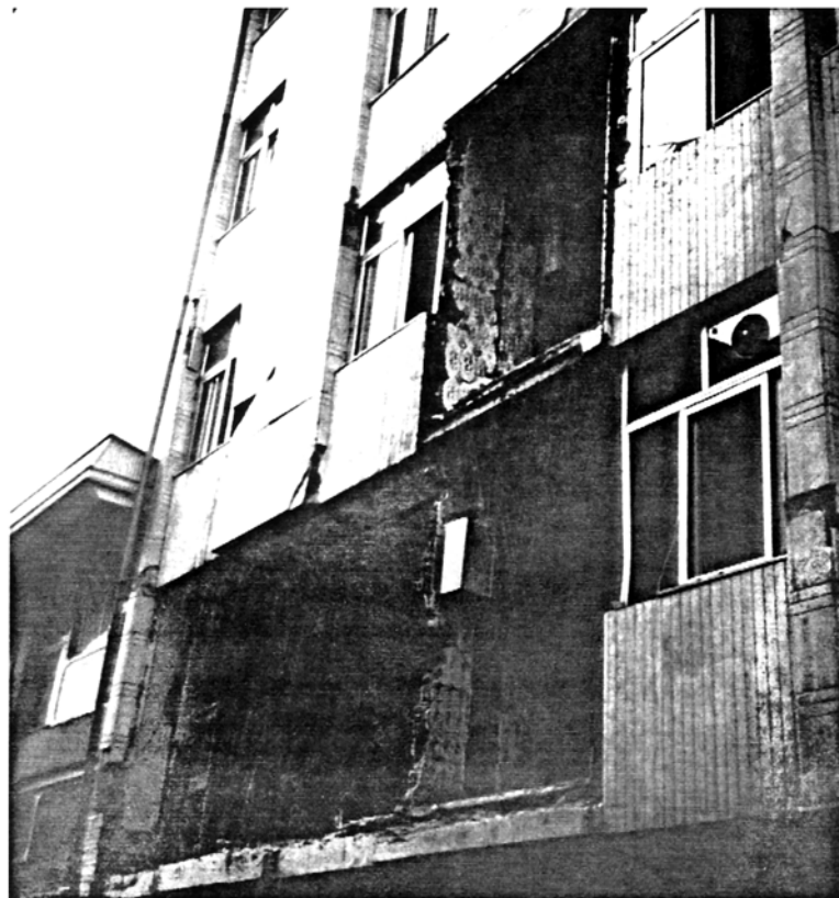
Picture 4.28 Seven-storey White Stone Clad Building, Rasht Collapse of a number of the unsupported infill walls
