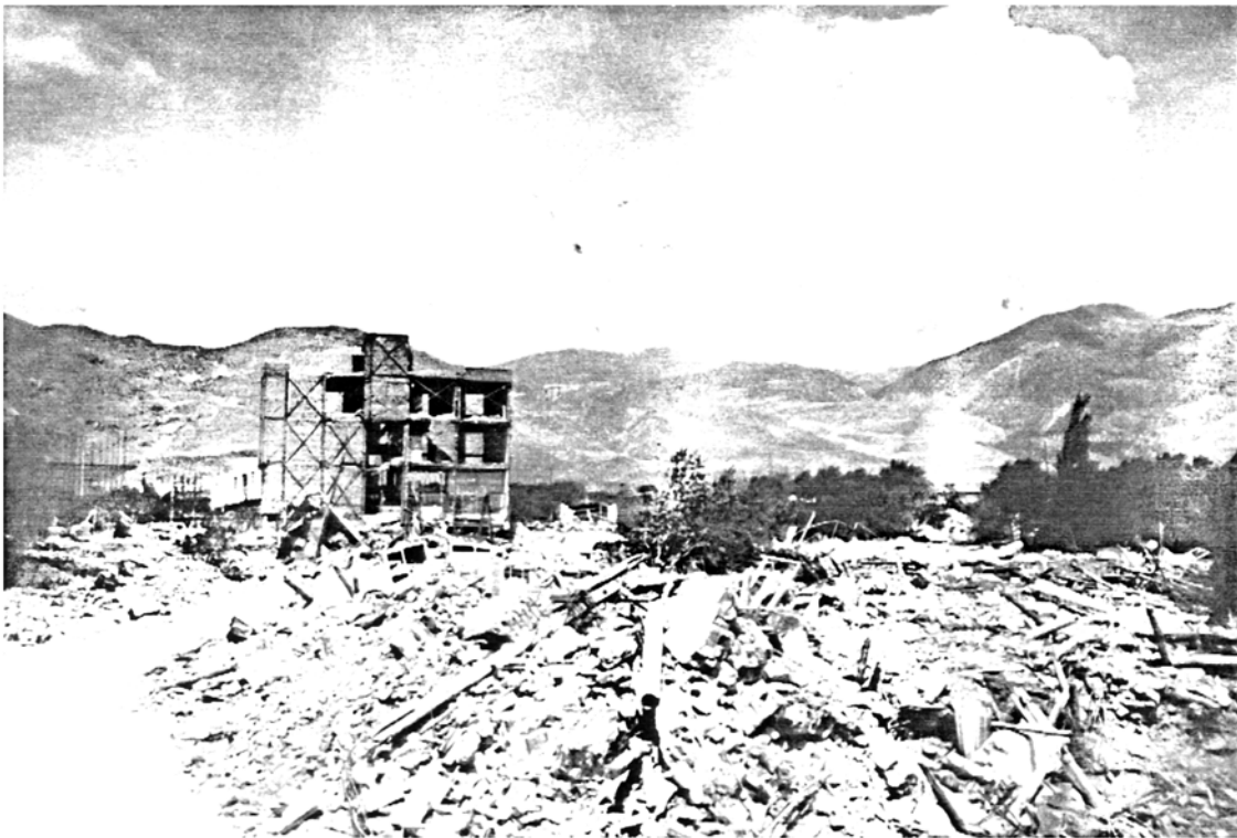
Picture 4.10 Better behaviour of this flexible steel frame building was as much due to its lower natural frequency of vibration as its relatively better construction, Manjil
