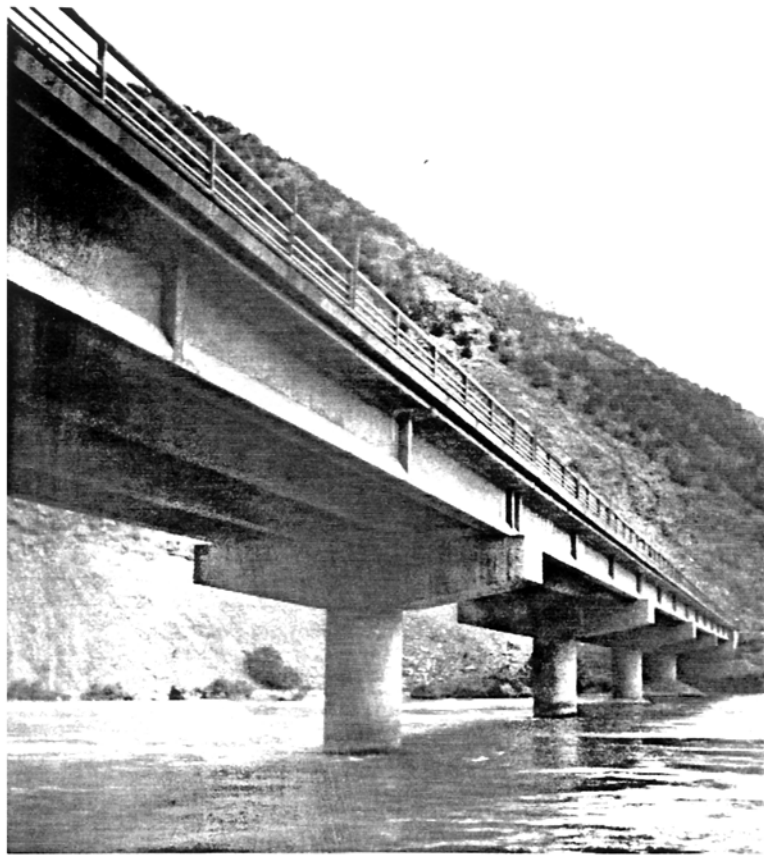
Picture 5.15 Concrete Bridge, Rudbar, West view
