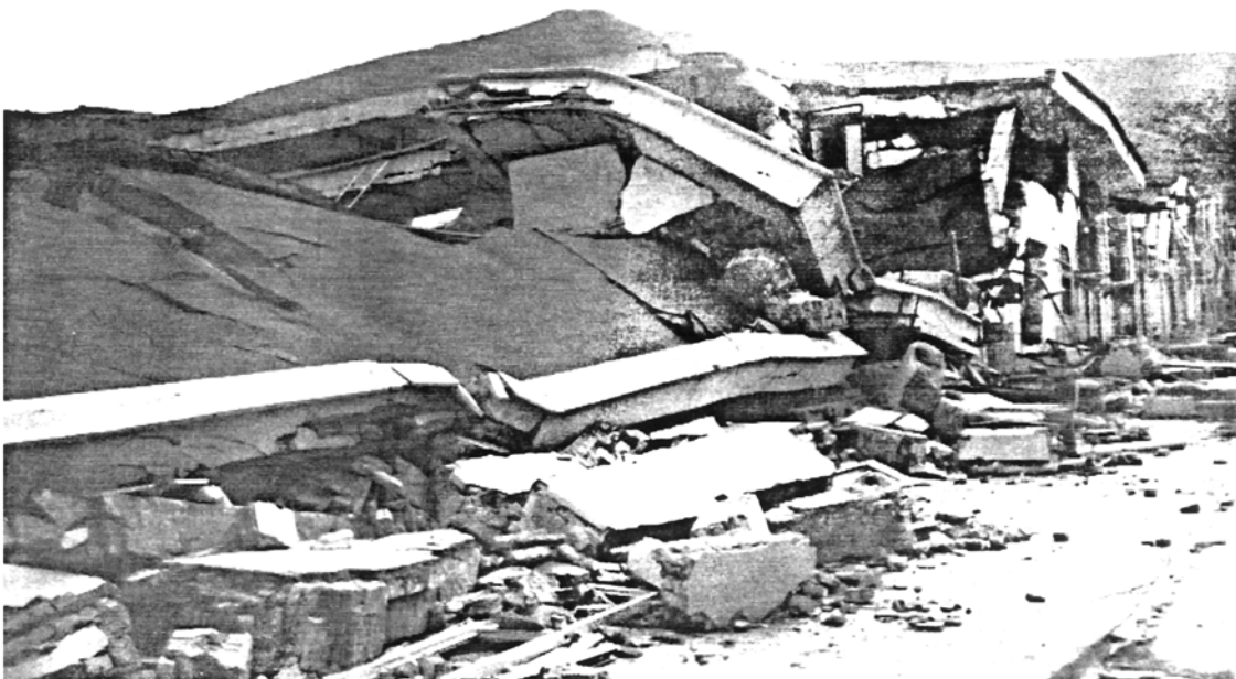
Picture 3.8 Vali-asr Hospital, Rudbar Destruction of casualty department due to weak vertical supports
