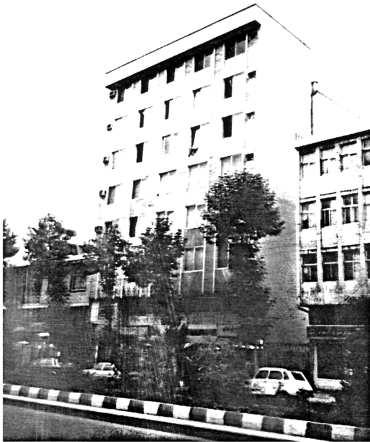
Picture 4.37 Eight-storey Grey Stone Clad Building, Rasht Another well constructed reinforced concrete building surviving the quake with minor damages
