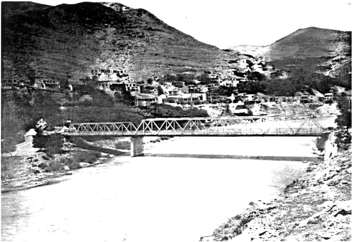
Picture 5.21 Steel Bridge, Rudbar. It behaved well during the earthquake
