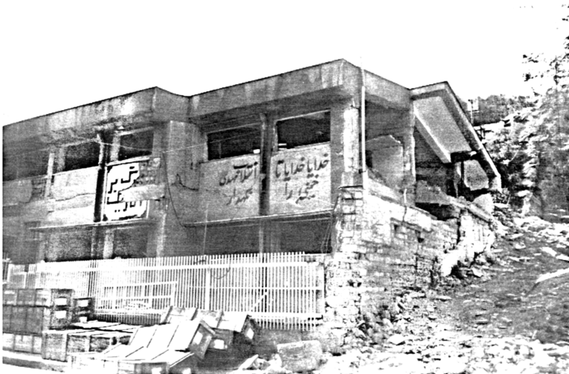
Picture 4.14 Telecom Building, Rudbar
