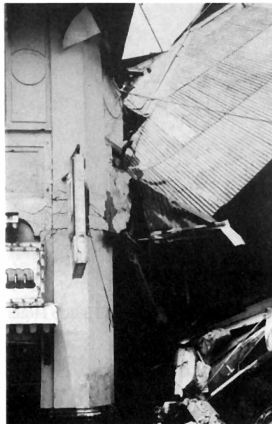
Impact damage caused by collapse of Baguio Park Hotel
