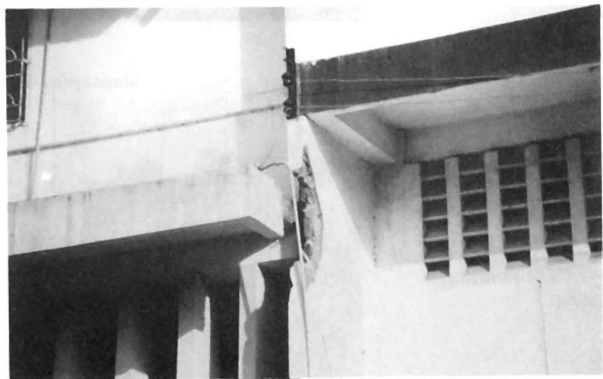
Figure 6.8 Buffeting damage in Dagupan
