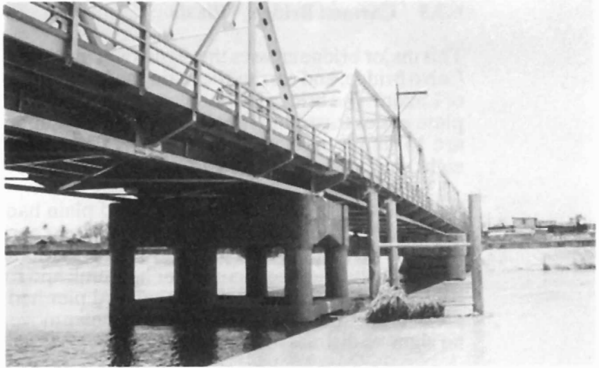
General view of Calvo Bridge, Bayambang
