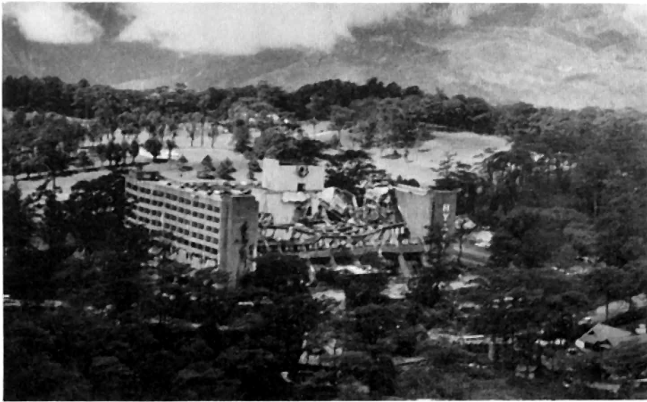
Figure 5.6 Hyatt Terraces Hotel from the air, looking south
