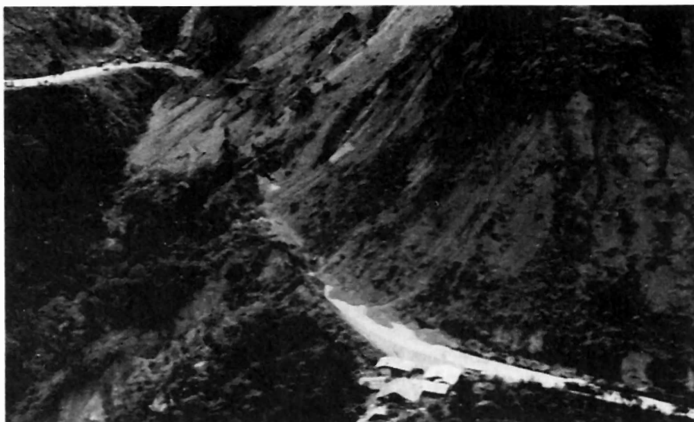
Figure 7.3 Slope failure in Dalton Pass
