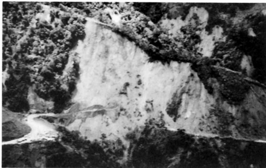
Figure 7.1 Landslide on Kennon Road below Baguio
