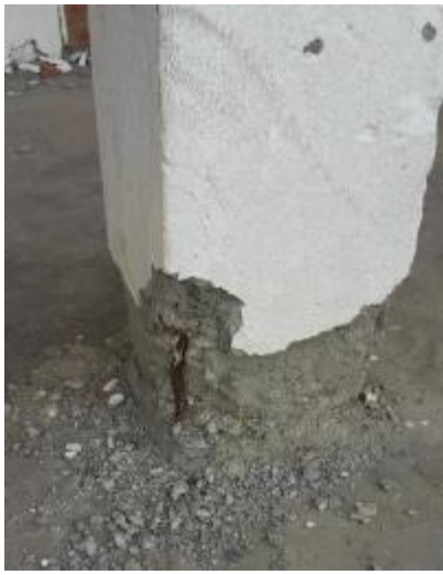
Figure 6-6 Damages in storey columns and walls in a RC-framed building.
