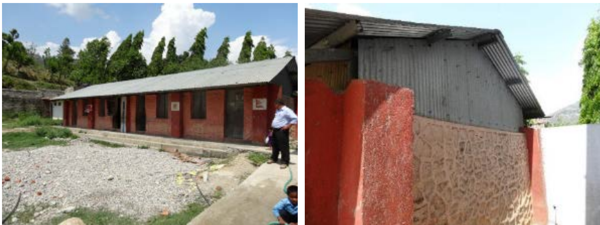
Figure 6-9 Stone rubble with mud mortar school.
