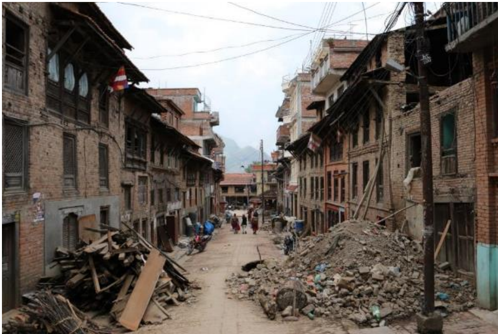
Figure 3-10 A street lined with traditional Newari housing. Sorted materials and propping are visible on masonry facades.
