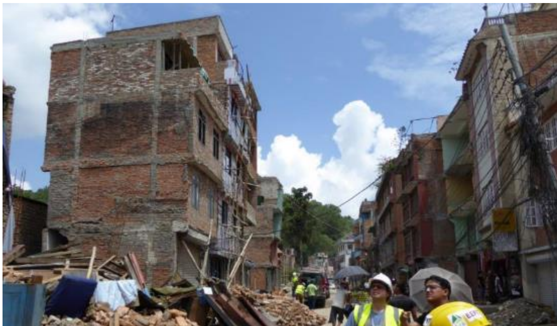
Figure 4-14 Examples of top-heavy concrete structures. Examples of top-heavy concrete structures, where upper floors cantilever out and the concrete frames do not extend to the corners of the building.
