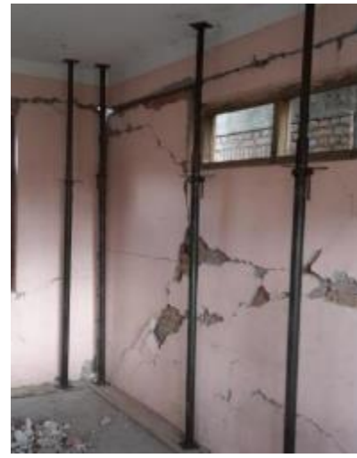
Figure 6-6 Damages in storey columns and walls in a RC-framed building.
