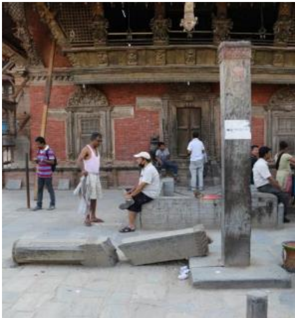
Figure 4-11 Evidence of rocking and overturning to monuments.
