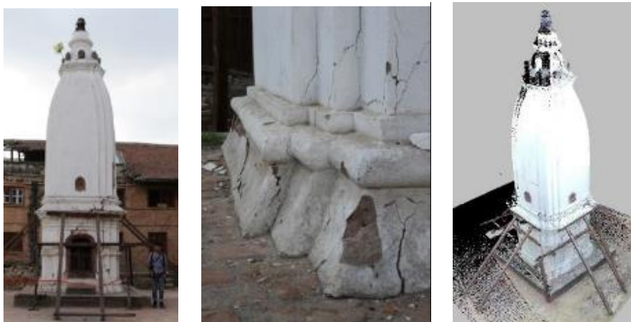
Figure 4-10 Evidence of rocking damage to a temple in Bachtapur Durbar.
