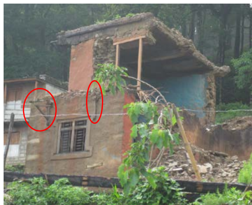
Figure 4-3 Out of plane failure.
