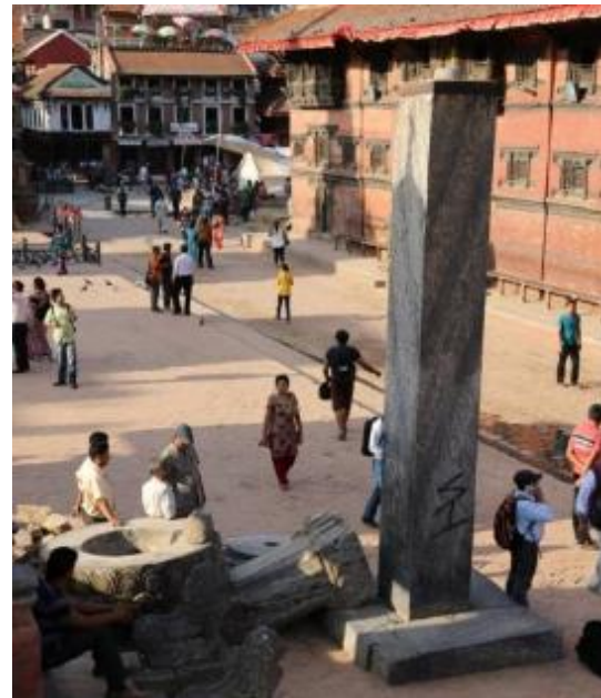
Figure 4-11 Evidence of rocking and overturning to monuments.
