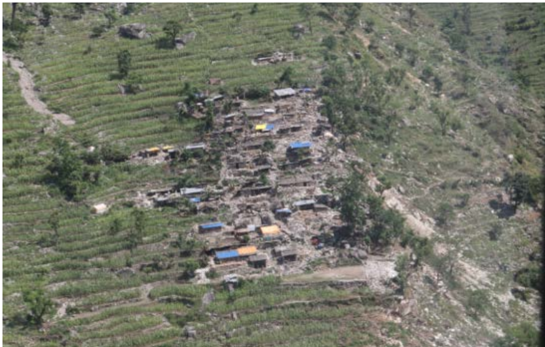
b) Very badly affected village. It is not known if this village was abandoned long before the earthquake and left to decay or whether it was caused by the earthquake, but the coloured roofs suggest the damage may have been recent.
