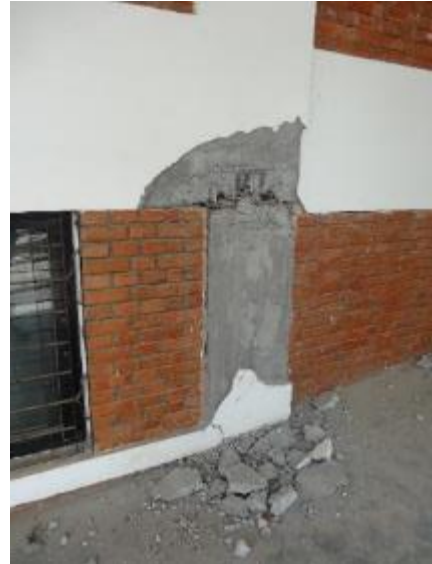
Figure 6-17 Damages in a two storey RC framed district hospital.
