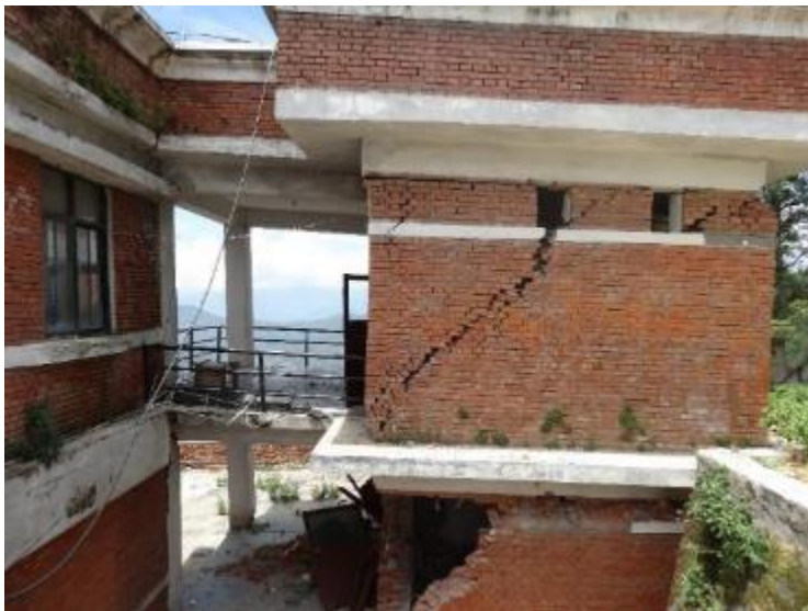
Figure 6-18 Damages in unreinforced masonry.
