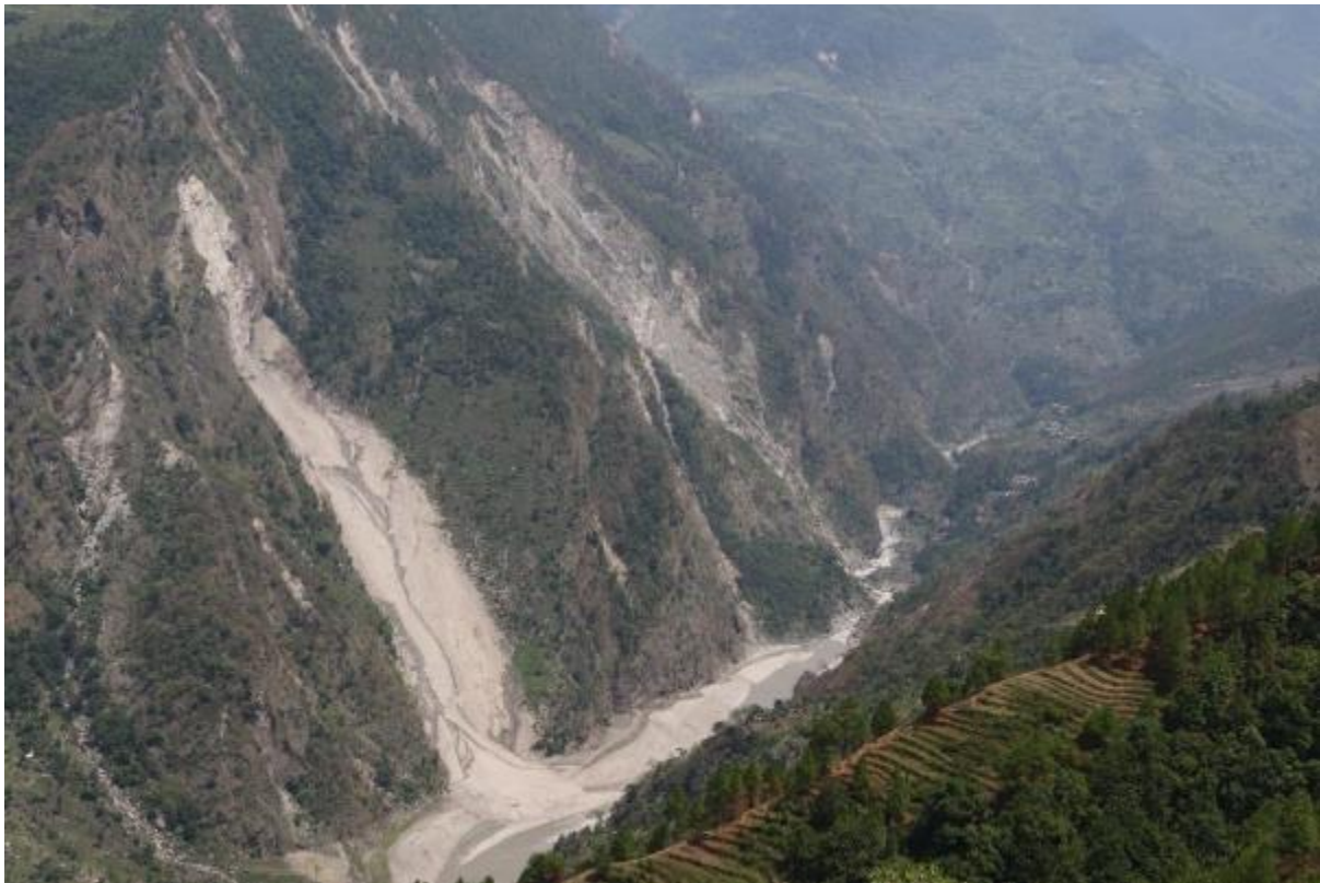
L) Deep landslide estimated to be over 200m in length.
