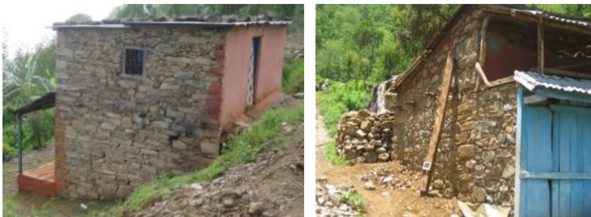
Figure 3-8 Stone structures built with traditional techniques.
