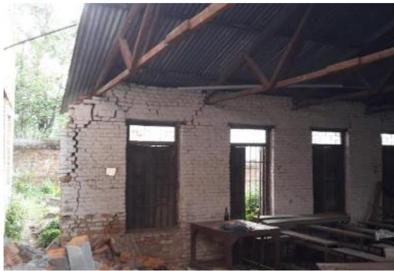
Figure 6-7 A fired clay brick school building with gable wall failure.
