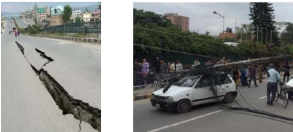
Figure 5-5 Infrastructure settled during the earthquake. Settlement damage to Araniko Highway (Goda et al. 2015) (Left). Foundational Collapse of a utility pole (Aydan and Ulusay 2015) (Right).
