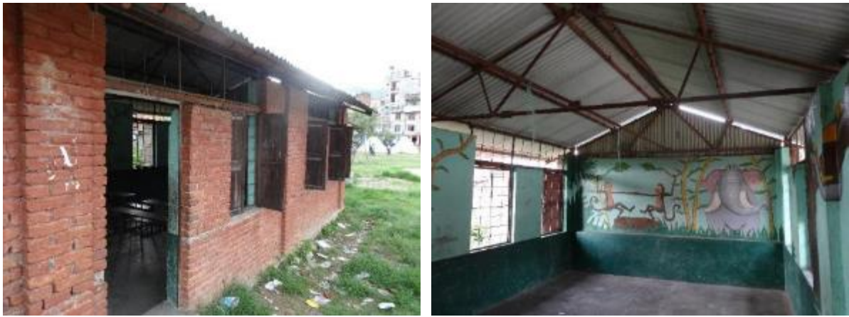
Figure 6-8 A fired clay brick school building with gable walls.
