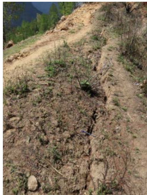
Figure 7-10 Tension Crack on the survey route.
