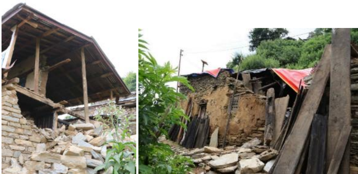
Figure 7-4 Examples of building and typical damage.
