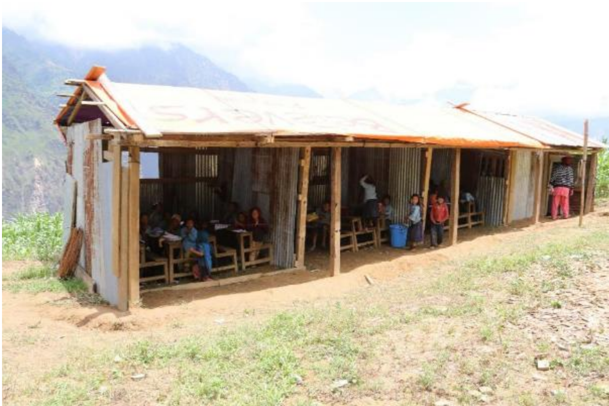
Figure 7-6 Temporary school building.
