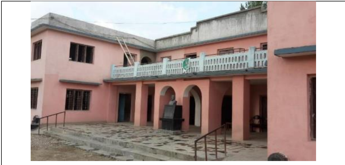
Figure 6-3 Adobe building with 2014 retrofit solution designed by NSET.
