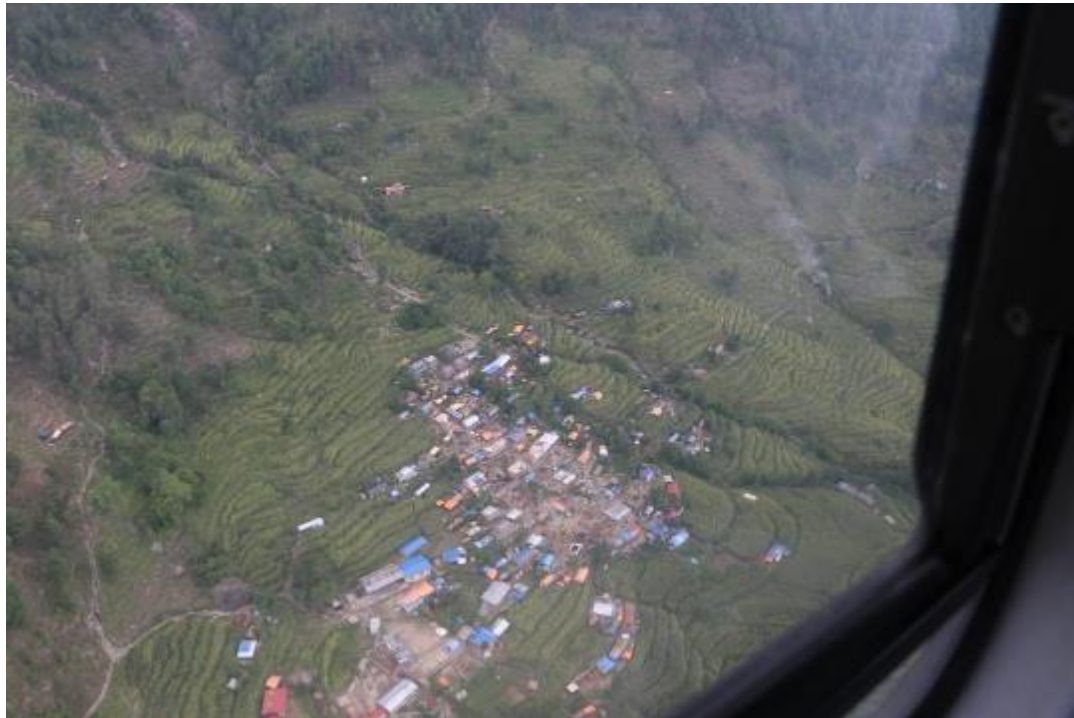
a) Badly affected village. This village sustained heavy levels of damage but this was not unusual in the villages that were overflown. The coloured roofs are usual (but not always) tarpaulins. These were necessary due to roofs collapsing when rubble masonry walls collapsed or sustained heavy damage.
