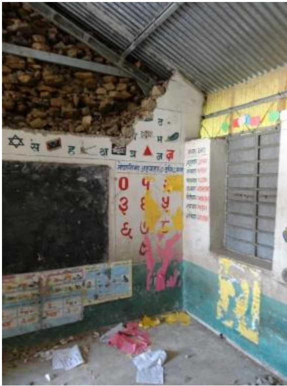
Figure 6-10 Interior view of stone rubble with mud mortar school.
