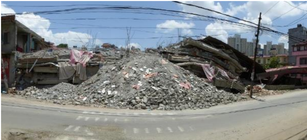
Figure 4-17 Pancake collapse of Morgan College -7-storey school in Tokha, Kathmandu.
