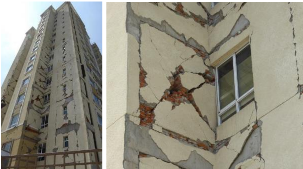
Figure 4-15 the Park View Horizon Apartments in Dhapasi.
