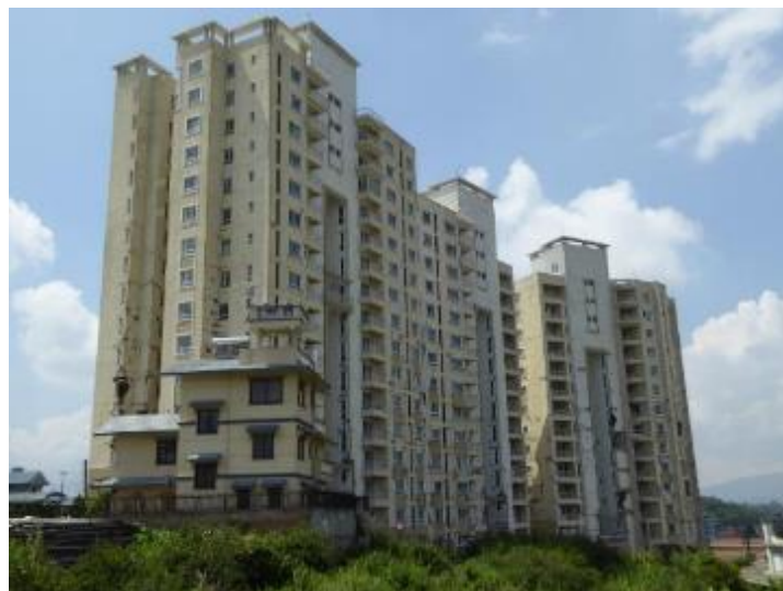
Figure 3-15 Park View Horizon Apartments in Dhapasi Kathmandu
