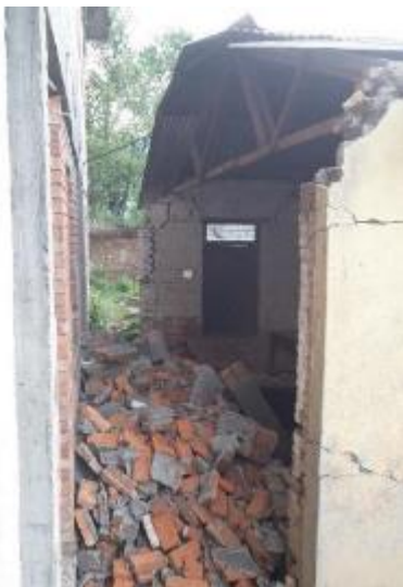
Figure 6-7 A fired clay brick school building with gable wall failure.
