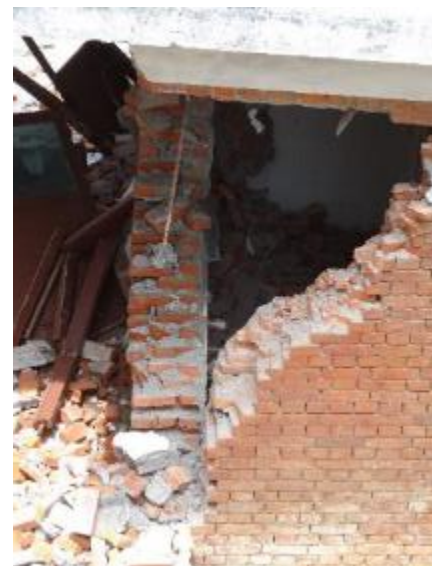
Figure 6-17 Damages in a two storey RC framed district hospital.
