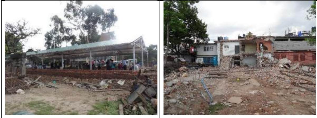
Figure 6-14 New prefabricated steel framed school vs. collapsed school.
