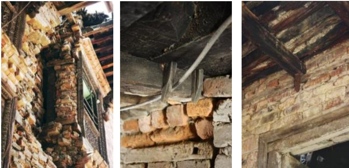
Figure 3-12 Examples of timber detailing in vernacular structures.
