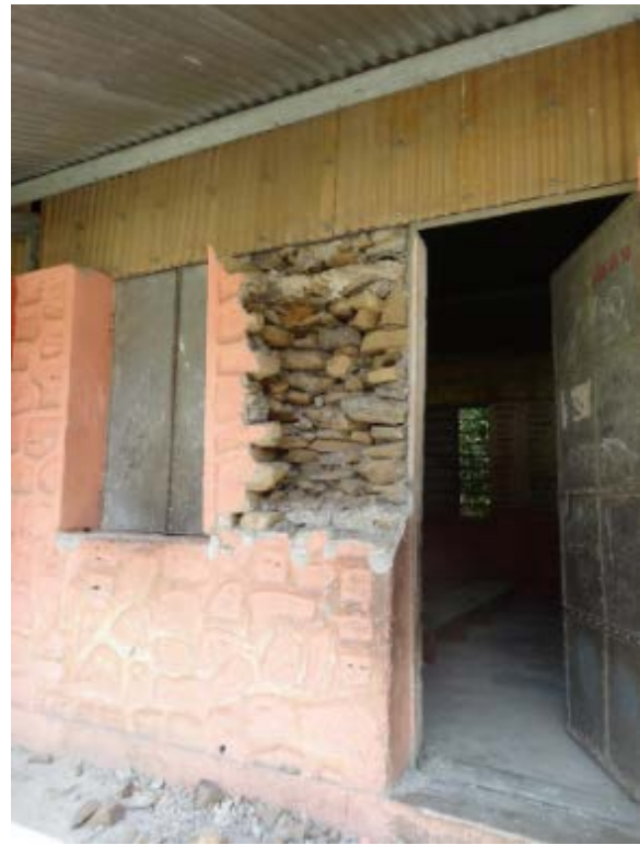
Figure 6-10 Interior view of stone rubble with mud mortar school.
