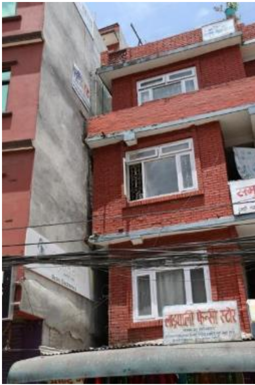
Figure 4-13 Evidence of pounding damage between adjacent concrete buildings.
