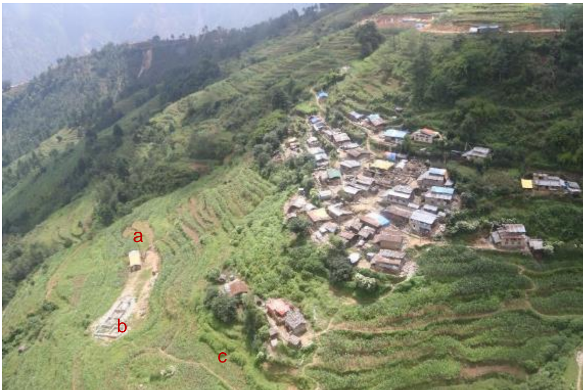
d) The village of Yamagaum. The buildings of this village were surveyed and are displayed in later figures. The locations of the various buildings mentioned in the report are indicated on this figure as a) new school building, b) temporary school building c) path to devastated school building (just out of shot).
