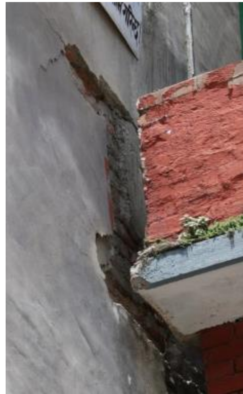
Figure 4-13 Evidence of pounding damage between adjacent concrete buildings.
