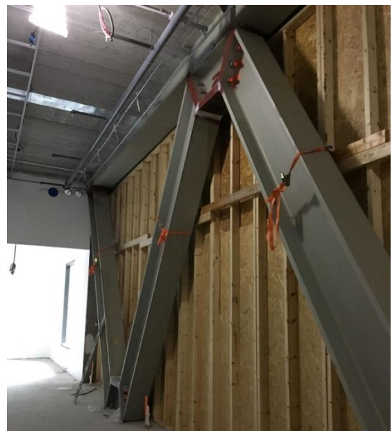
Figure 13- Large Steel Truss at Ground Floor
