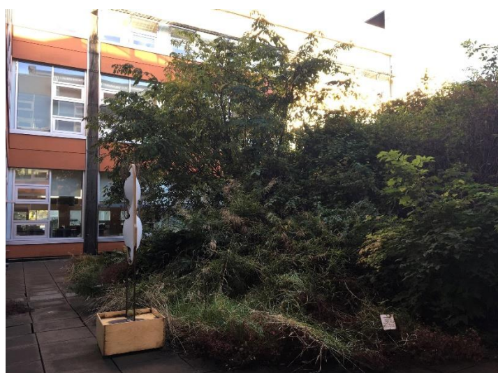
Figure 23 – Biodiverse green roof
