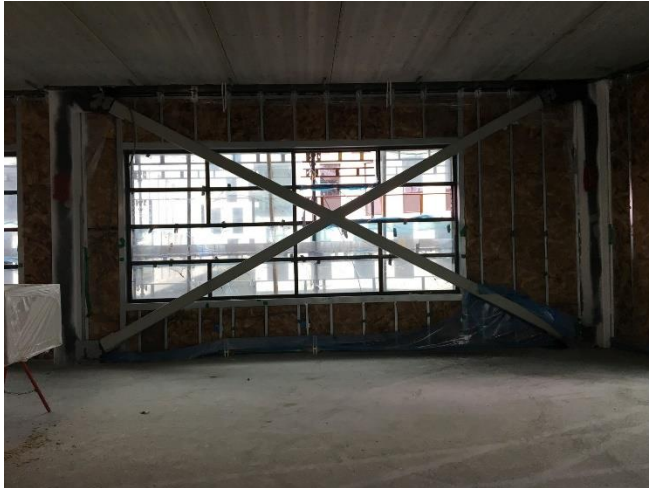
Figure 14 – Bracing needed for lateral stability, made into a feature
