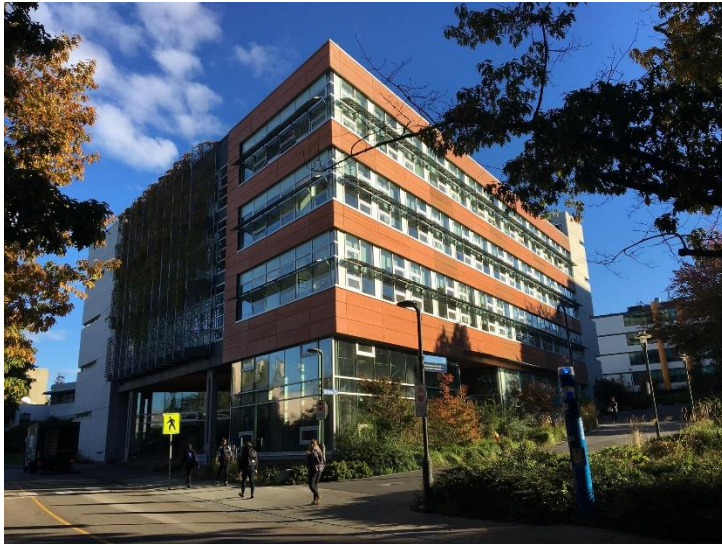
Figure 19 – CIRS Building, UBC
