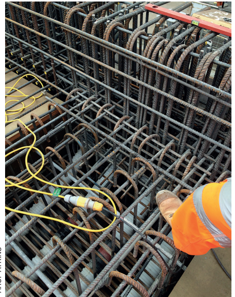
Figure 9 View of end block to post-tensioned spine beam
