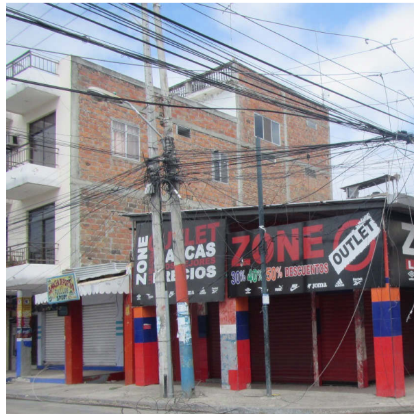
Figure 12 - Set back additional floors in Manta, Ecuador © EEFIT
