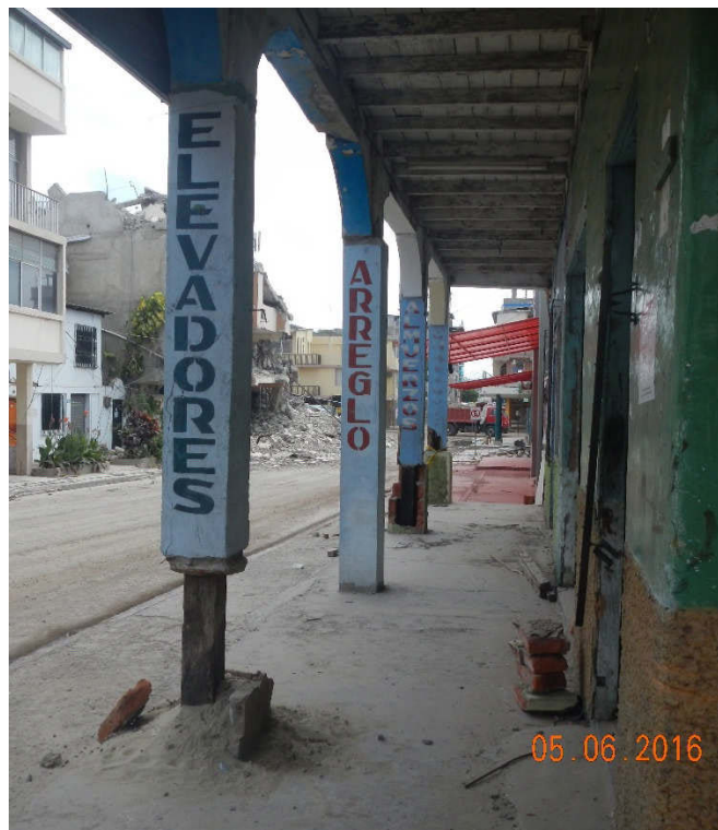
Figure 9 - Hidden timber structure, Manta, Ecuador © EEFIT
