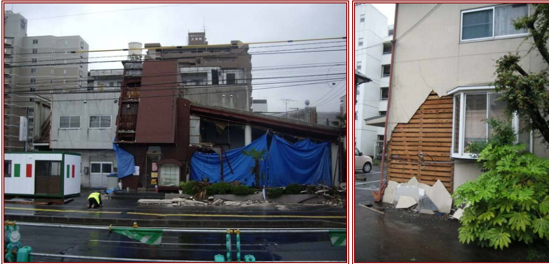
Figure 8.6 Earthquake-induced damage on low-rise wooden structures
