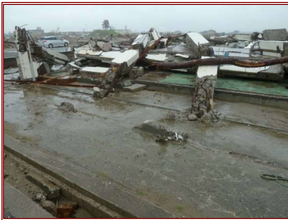
Figure 7.61 (left) Failure of RC columns showing flow direction adjacent to Yuriage port.
