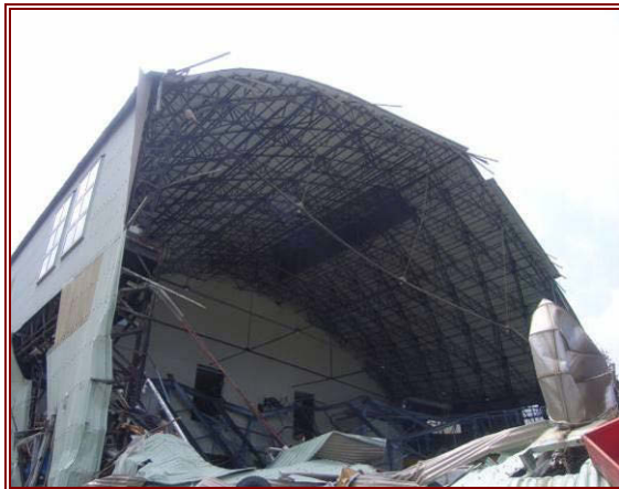
Figure 7.8 (left) Large trussed portal frame structure of the Nippon Steel Factory, at the eastern end of remaining structure.
