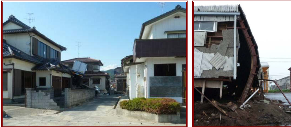
Figure 7.49 (left) Lorry trailer deposited on the first floor roof of house (centre of photo) but otherwise minor damage to the adjacent timber frame structures. Collapsed timber frame structures were also recorded at this observation point.
