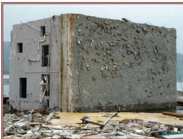
Figure 7.38 (left) Scour may have contributed to the overturning failures of several RC buildings.
