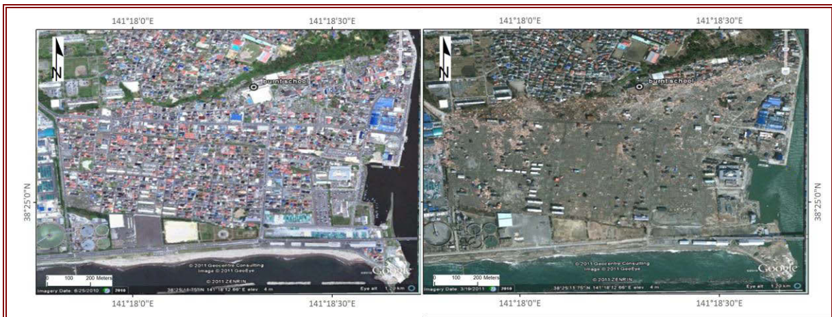
Figure 7.48 Area of destruction west of the Kitakami River mouth in Ishinomaki (left image is dated 25 th June 2010; right image is dated 19 th March 2011). The burnt school, indicated, is discussed further in section 10.1.5. Land increases in elevation abruptly, initially to around 10 m at the line of trees in the north of this image.
