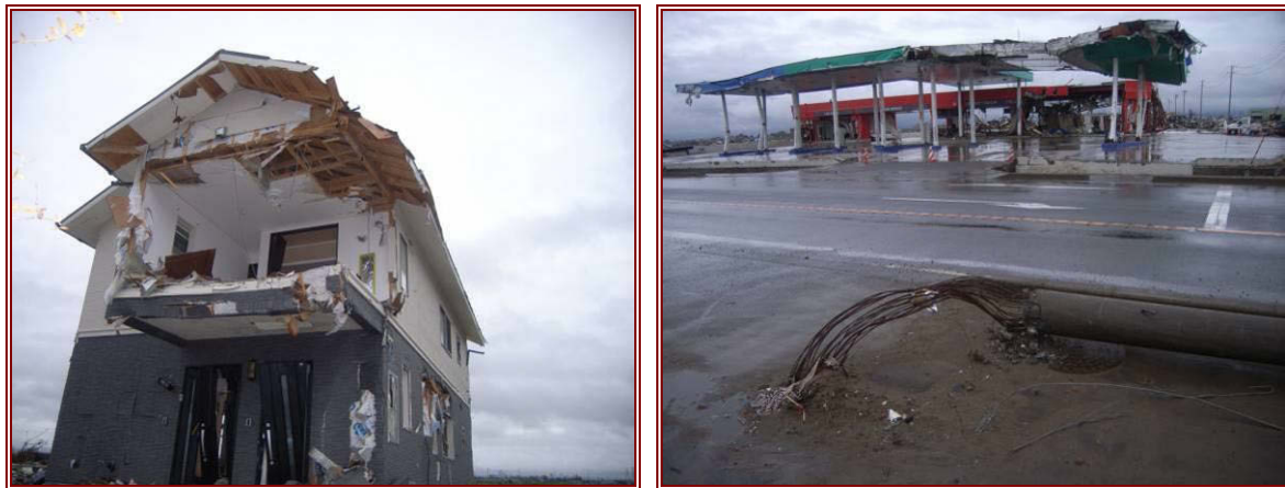
Figure 7.51 (left) Many timber houses sustained heavy damage or partial / complete collapse (D4).
