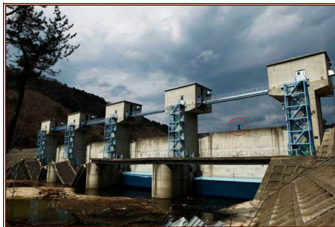
Figure 6.21 Tsunami sluice gates at Fudai. Notice the man walking along the top of the wall for scale (Komo News, 2011).
