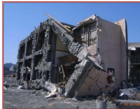
Figure 7.44 (left) View of building E showing out-of-plane failure of an infill wall.
