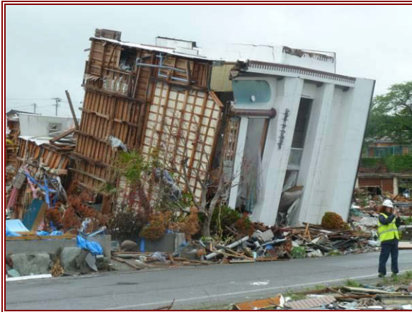
Figure 7.16 (left) An overturned timber building in Ōfunato.
