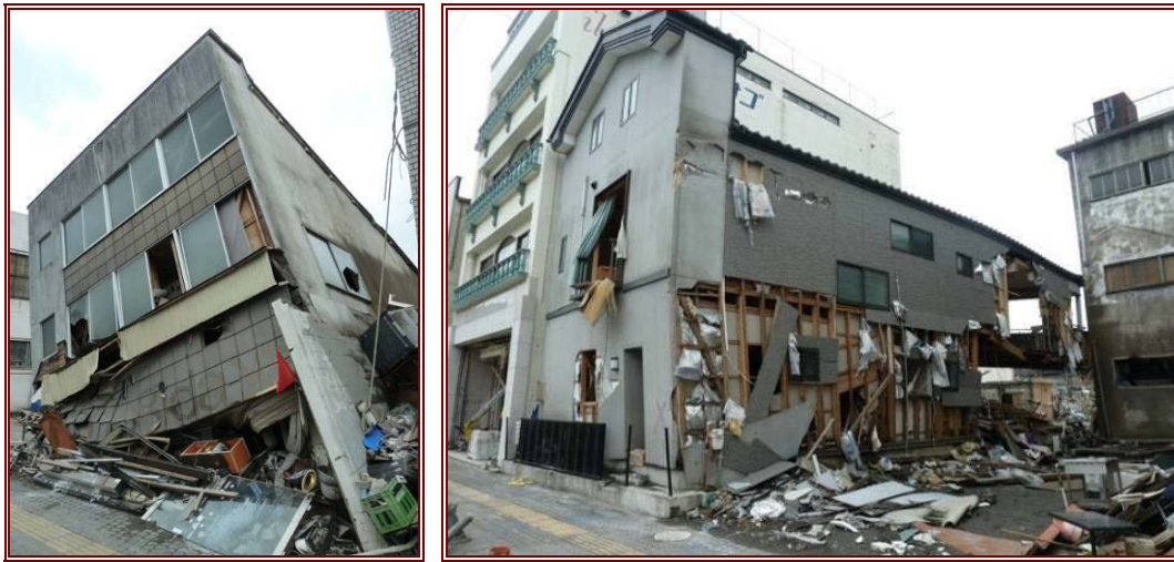
(g) Timber frame, D4, 7 m inundation.
