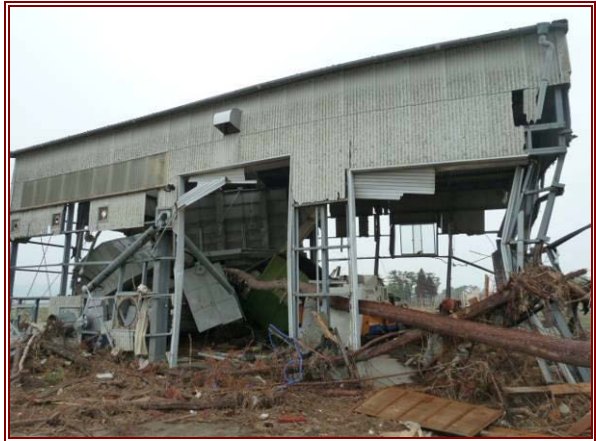
Figure 7.68 (left) View of the front of steel building, struck by tree trunk on left structural column. Tsunami flow inland was towards this face of the building.
