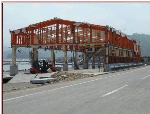
Figure 7.2 (right) Steel-frame hotel in Tarō Town showing heavy damage to the third floor and minor damage at the 4 th floor.
