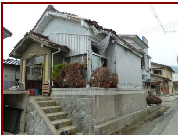
Figure 7.28 (left) Raised concrete foundation; structure built 2 m from ground level, 660 m inland and 100 m from Shikaori River. Inundation depth was approximately 6 m in the area around this building.
