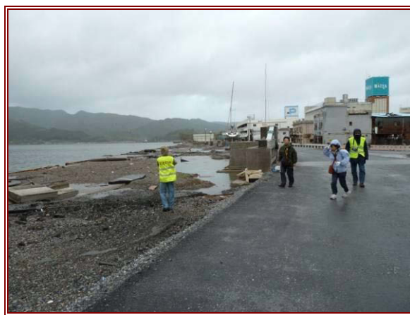
Figure 6.3 Quayside at Ōfunato City, showing limited freeboard of the quay walls
