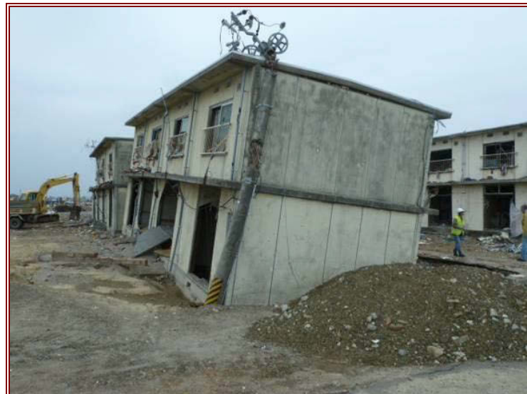
Figure 7.64 (left) View along the north side of one apartment block, illustrating scour of the full length of building.
