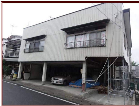
(d) Damaged house at the ground floor level
