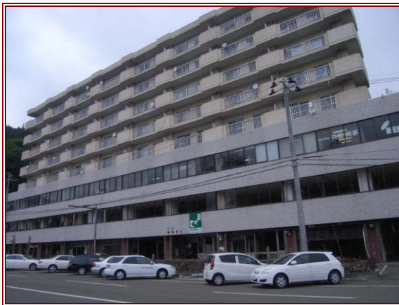
Figure 10.12 (left) Eight-storey RC frame evacuation structure with steel frame structure on the seaward face. Two external staircases for the fourth floor exist on the other side of the building.
