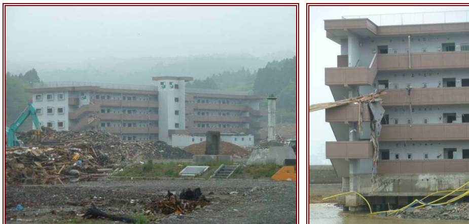
Figure 10.14 (left) Harbour-front designated evacuation structure. Vertical Evacuation signage (green) is visible on the landward (rear) side and at external staircases.
