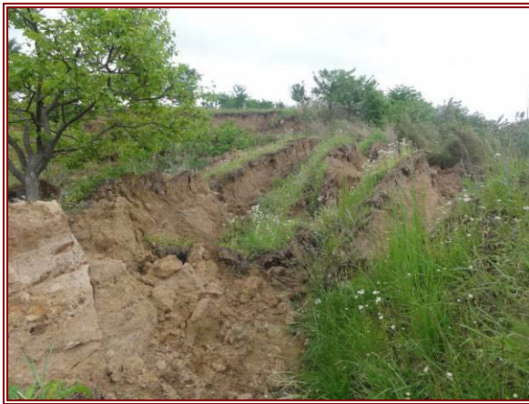
(c) Loose sections of displaced soil
