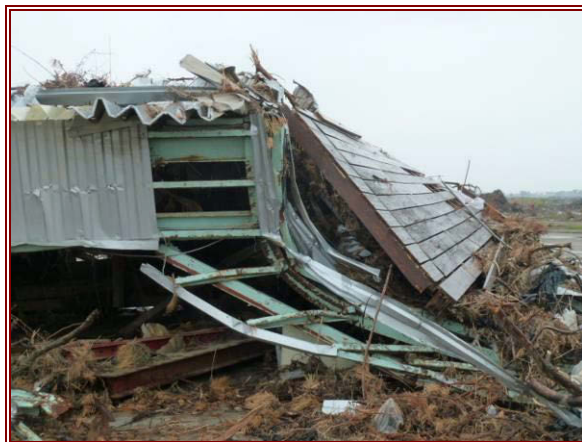
Figure 7.70 (left) View of the front left corner of the building, which appears to have been the column struck by debris.
