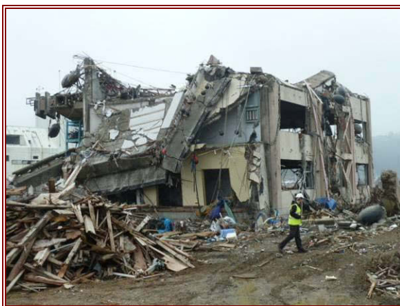
Figure 7.31 (left) Collapse of third storey of a RC building in Shiomi-cho, 100 m from the sea (38° 40' 29.10" N, 141° 26' 44.96" E).
