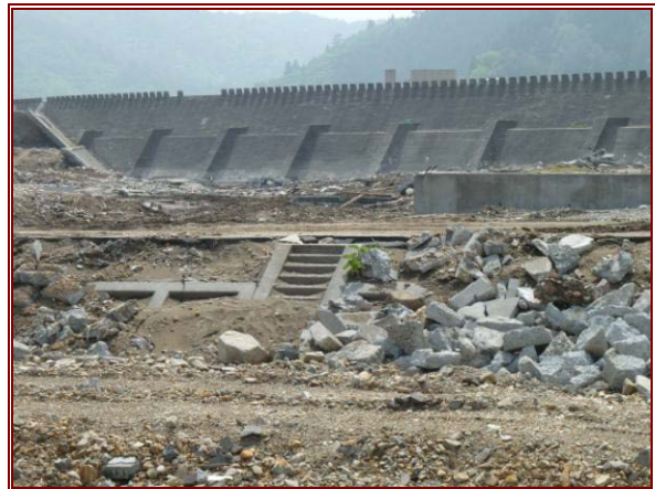
Figure 6.7 (left) A surviving gate structure and buttresses in Tarō. The seawall has been destroyed either side of this gate.
