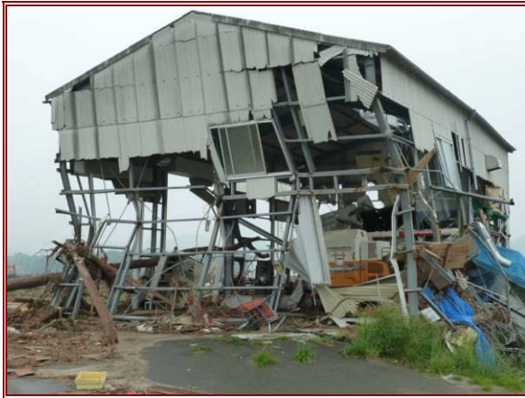
Figure 7.68 (left) View of the front of steel building, struck by tree trunk on left structural column. Tsunami flow inland was towards this face of the building.
