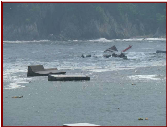
Figure 6.7 (left) A surviving gate structure and buttresses in Tarō. The seawall has been destroyed either side of this gate.
