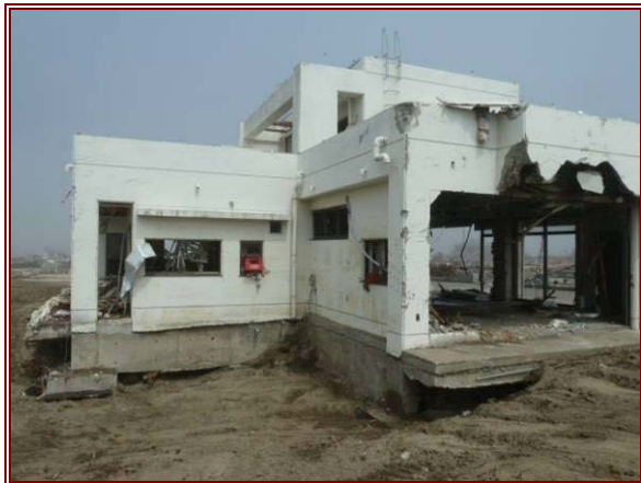
Figure 7.53 (left) Tilting due to scour on the seaward side of a residential building in Wakabayashi-ku.
