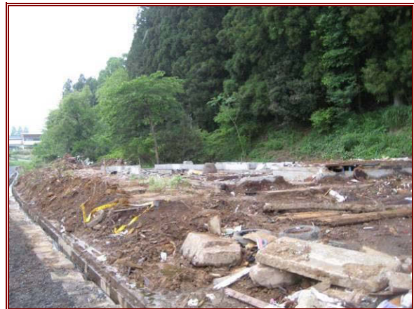
(d) Foundations of destroyed houses
