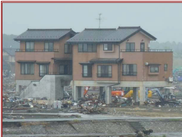
Figure 7.59 (left) Residential buildings in Yuriage constructed with an open ground floor.
