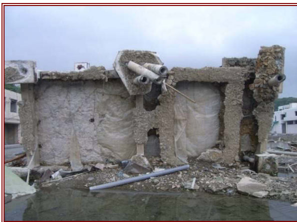
Figure 7.36 (left) Foundations of building A showing some piles remain connected to the pile cap.
