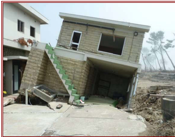
Figure 7.53 (left) Tilting due to scour on the seaward side of a residential building in Wakabayashi-ku.
