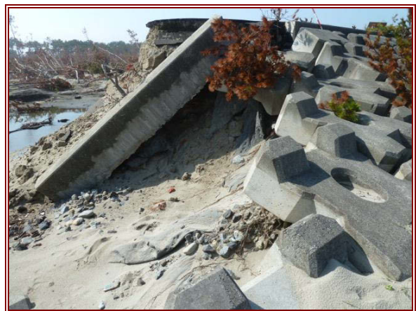
Figure 6.18 (left) Seaward side of concrete block revetment at Arahama Beach.
