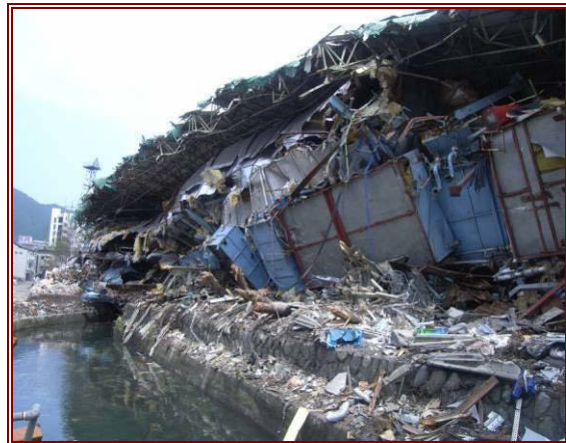
Figure 7.8 (left) Large trussed portal frame structure of the Nippon Steel Factory, at the eastern end of remaining structure.
