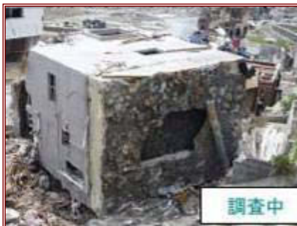
Figure 7.40 (left) Building C (a hotel) transported 30 m landward from its original location (image from Shuto, 2011).
