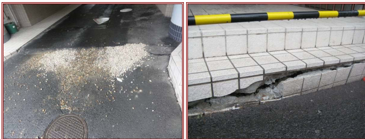
Figure 8.4 Lower building settlement relative to surrounding ground, in Yamato-machi, Sendai City.
