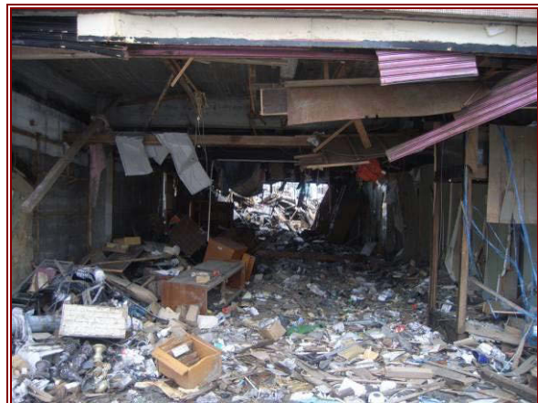
Figure 7.10 (left) Water and some debris were able to pass through the structure limiting the amount of shelter this building was able to provide to the buildings behind.
