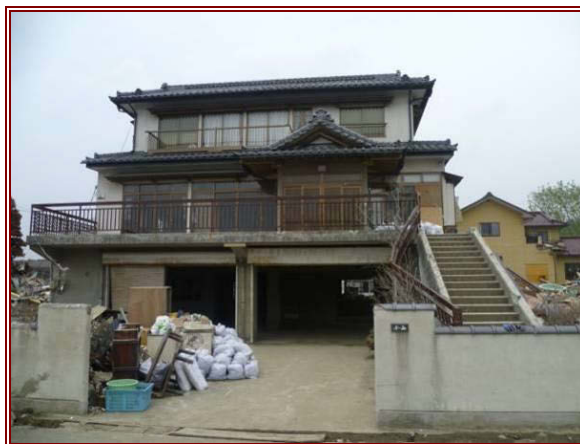
Figure 7.28 (left) Raised concrete foundation; structure built 2 m from ground level, 660 m inland and 100 m from Shikaori River. Inundation depth was approximately 6 m in the area around this building.
