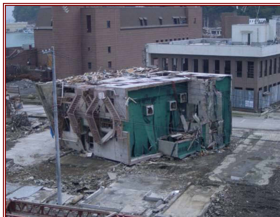
Figure 7.40 (left) Building C (a hotel) transported 30 m landward from its original location (image from Shuto, 2011).
