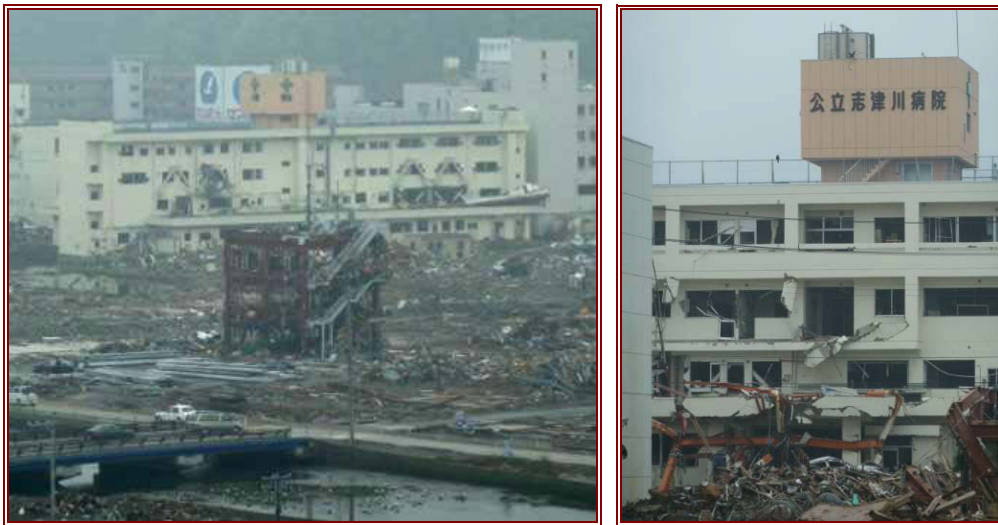
Figure 10.16 (left) View of the hospital (landward side) with steel bracing and damage to third storey visible.
