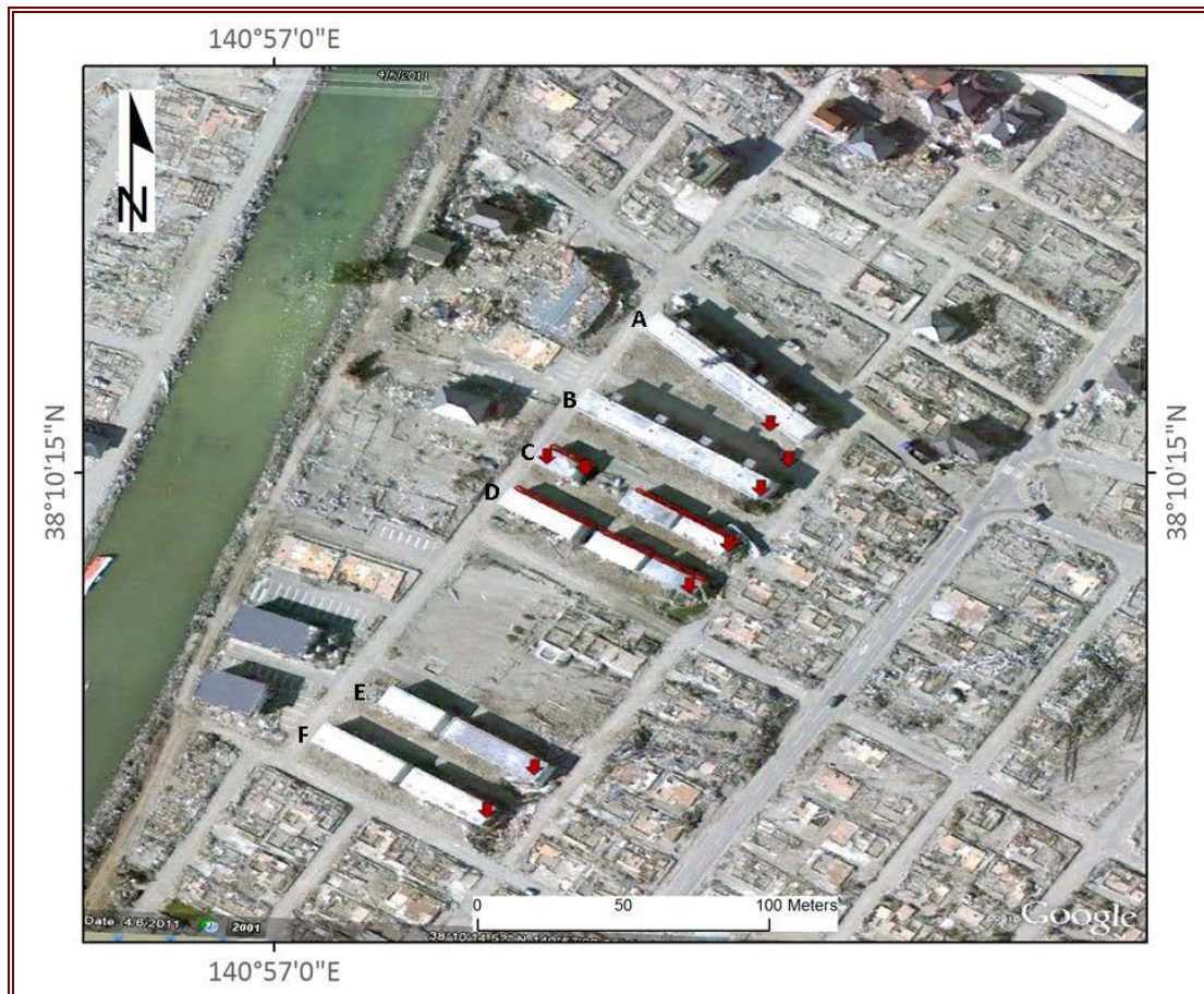
Figure 7.63 Aerial photograph of apartments in Natori with significant scour at the seaward end and northern side of each building. Scour is indicated by red polygons along the northern side of buildings, and red arrows (primarily at the south-eastern ends).
