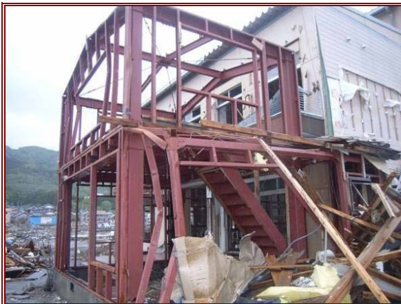
Figure 7.18 (left) Cladding had been washed away (or subsequently removed) and steel frame appears to have suffered impact damage but the structural steel frame seemed intact.
