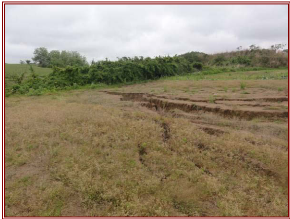
(d) Tension cracks near summit of slope
