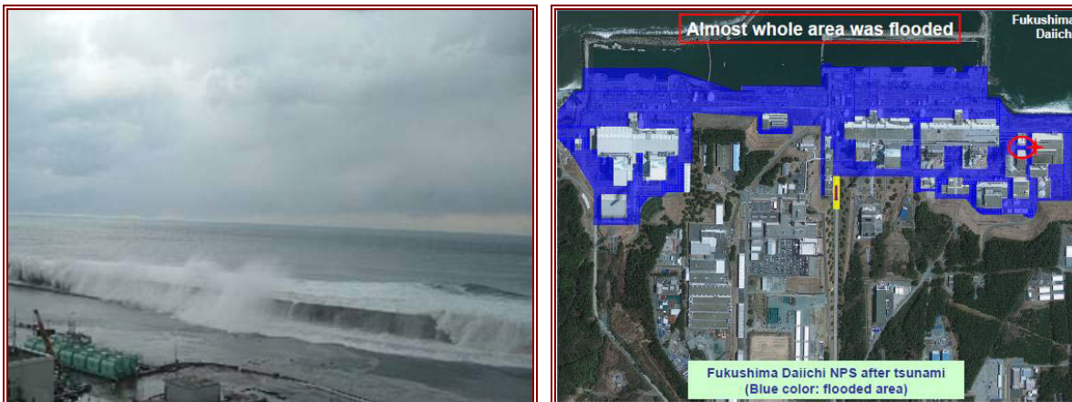
Figure 9.3 (left) Tsunami overtopping sea defences at Fukushima Daiichi (TEPCO, 2011b).
