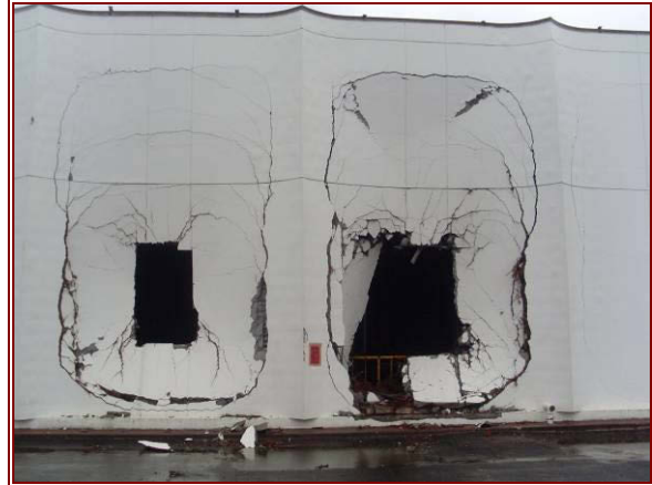
Figure 9.9 (left) Tsunami at Minami Gamou Sewage Treatment Plant (Sendai City, 2011a).
