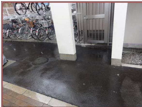
Figure 8.4 Lower building settlement relative to surrounding ground, in Yamato-machi, Sendai City.
