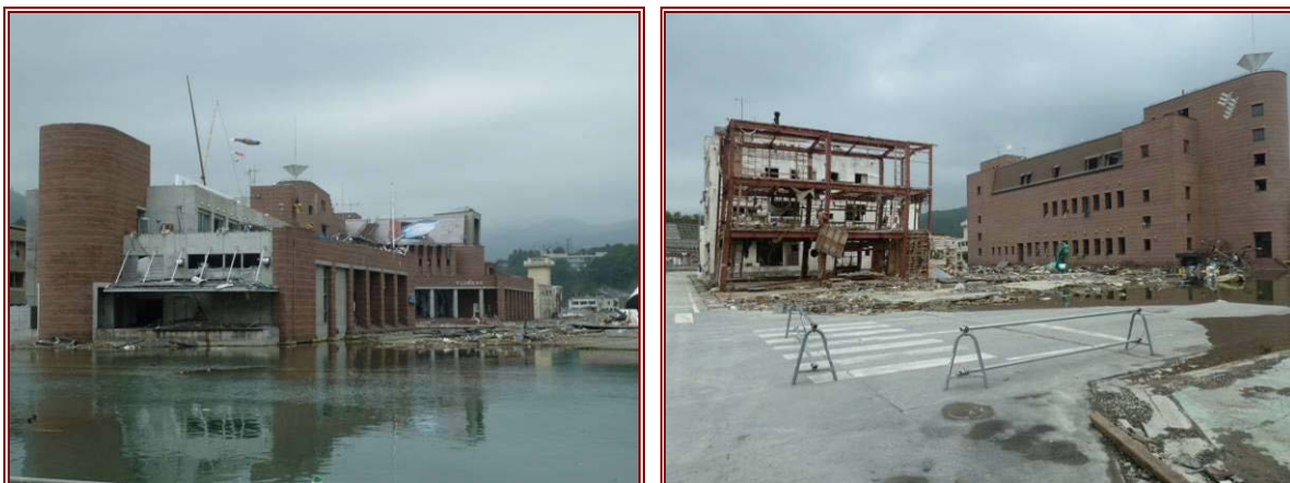
Figure 7.46 (left) Seaward side of the harbour-front buildings.
