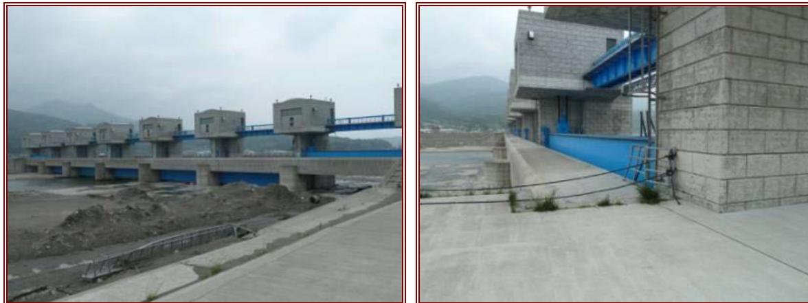
Figure 6.22 Tsunami gates on the Tsugaruishi River in Miyako Bay.
