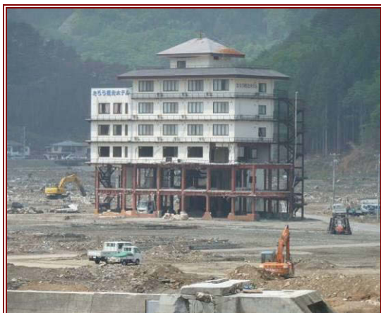
Figure 7.2 (right) Steel-frame hotel in Tarō Town showing heavy damage to the third floor and minor damage at the 4 th floor.
