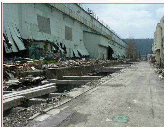
Figure 7.10 (left) Water and some debris were able to pass through the structure limiting the amount of shelter this building was able to provide to the buildings behind.
