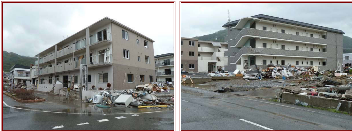
Figure 7.20 (left) RC shear wall building with separate front and rear entrances in the seaward and inland side. Seaward view is shown. The building flooded all the way to the top but its structure remained almost intact.
