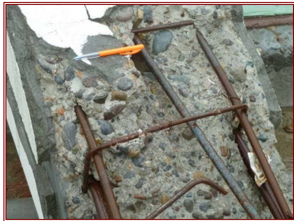
Figure 7.61 (left) Failure of RC columns showing flow direction adjacent to Yuriage port.
