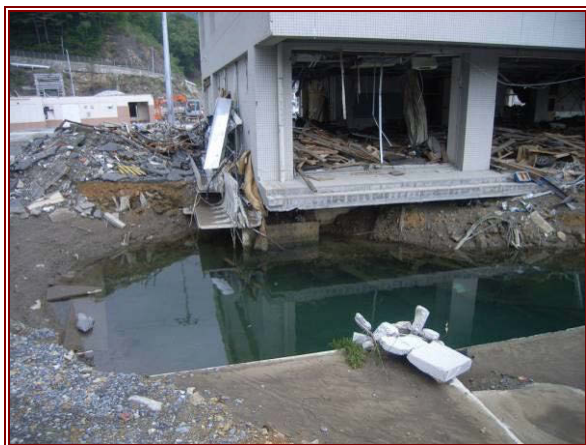
Figure 7.38 (left) Scour may have contributed to the overturning failures of several RC buildings.
