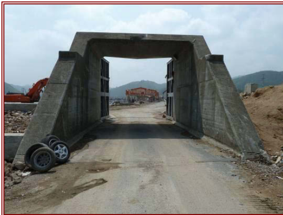
Figure 6.7 (left) A surviving gate structure and buttresses in Tarō. The seawall has been destroyed either side of this gate.
