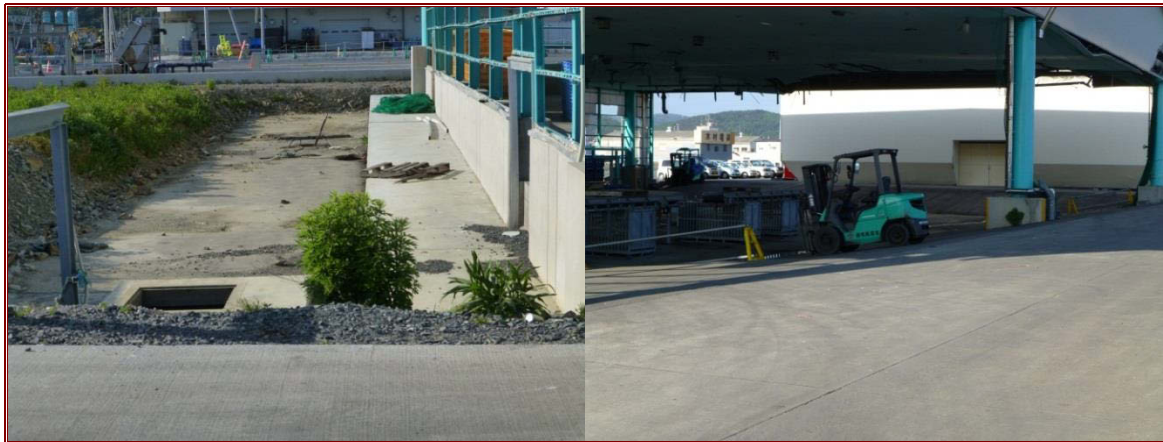
Figure 3.13 (left) Old and new ground levels at Ishinomaki fishing port.
