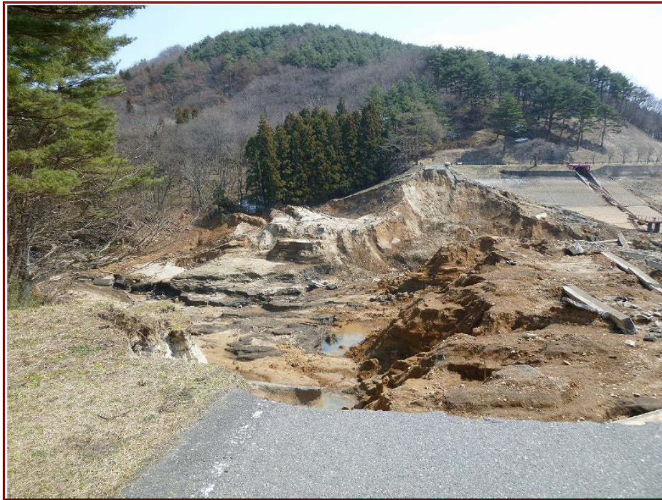
Figure 4.21 Fujinuma main dam after the earthquake (Matsumoto, 2011).
