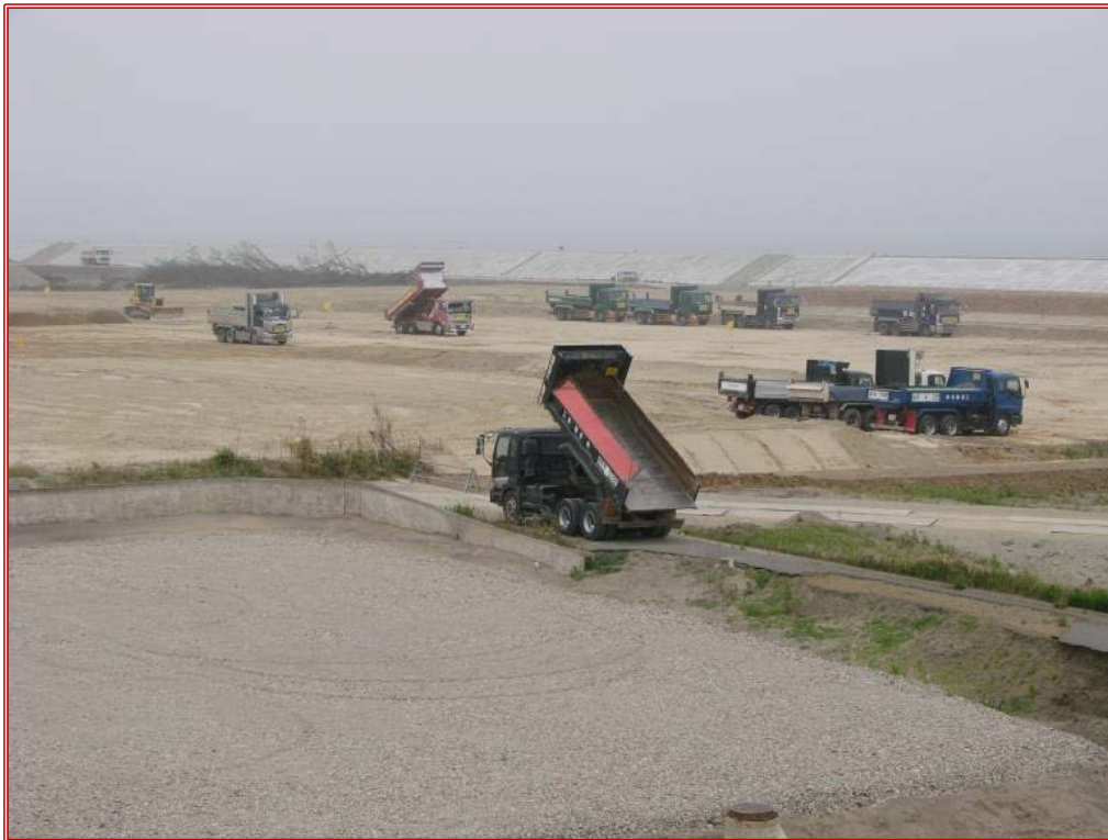
Figure 7.1 Elevated plinth for housing under construction at Iwanuma.
