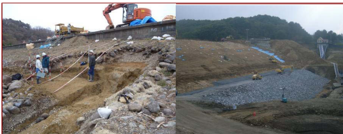
Figure 4.19 Repair works on the upstream surface of the Nishigo Dam (Matsumoto, 2013).
