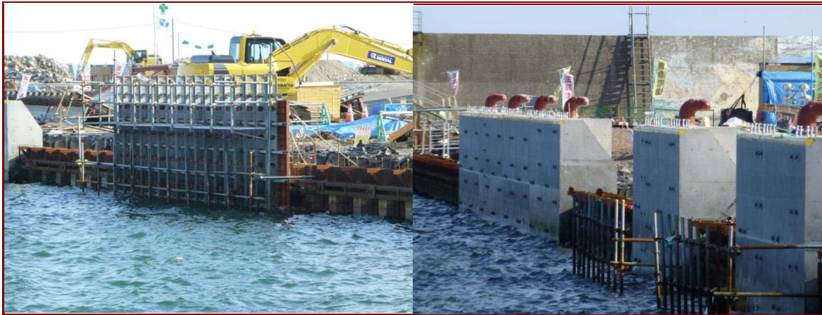
Figure 3.18 (left) Formwork at Ishinomaki.
