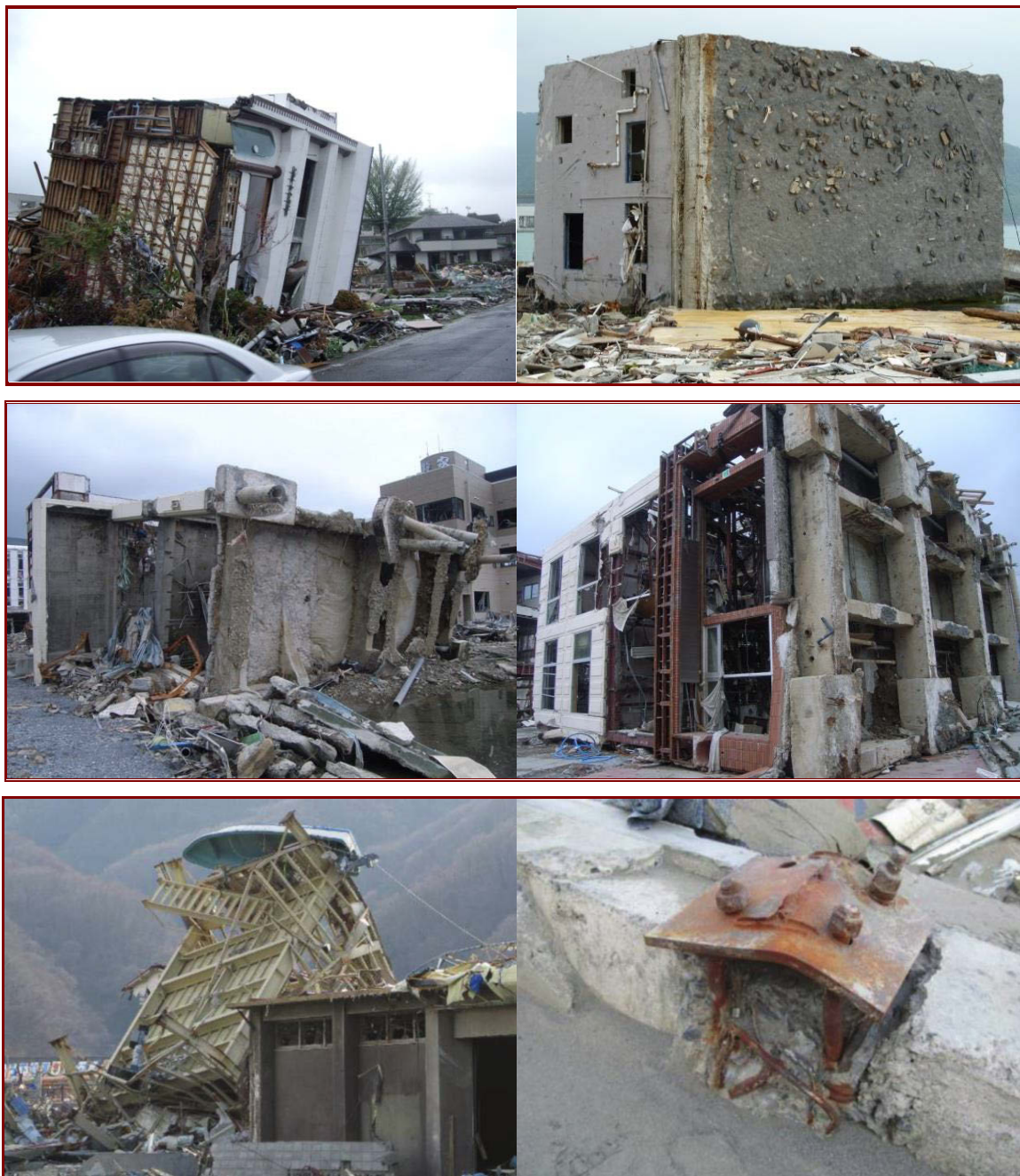
Figure 2.10 Overturning of structures due to a combination of tsunami effects (lateral fluid forces, buoyancy, debris impact and foundation failure).
