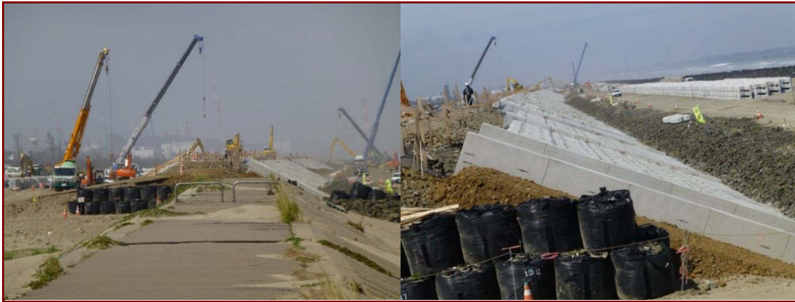
Figure 3.7 (left) Construction of revetments at Arahama.
