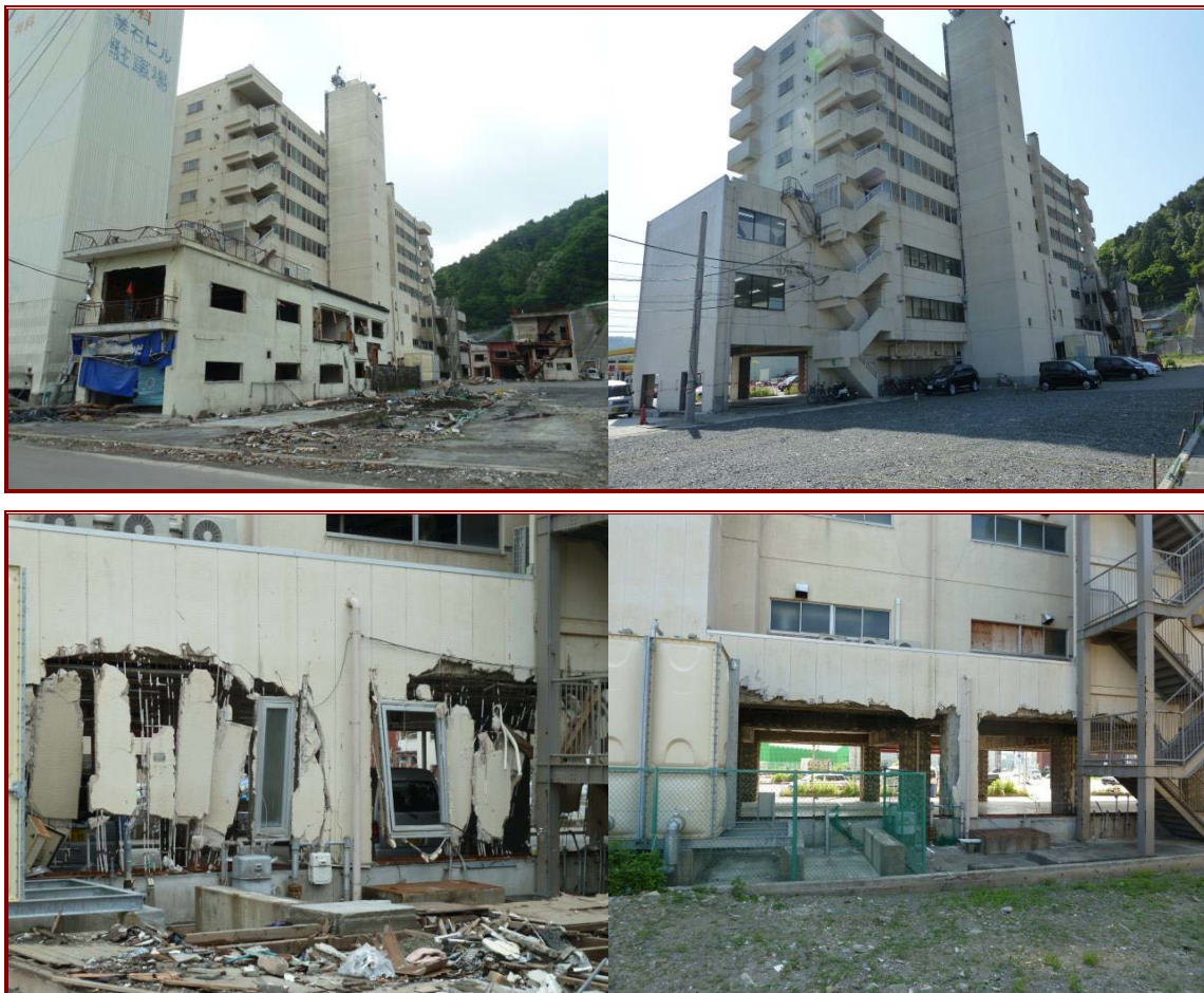
Figure 2.16 8-storey mixed-use RC vertical evacuation structure in 2011 (left) and 2013 (right).
