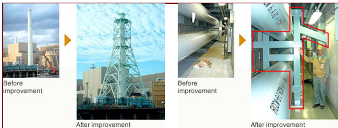
Figure 4.10 Seismic strengthening work undertaken in Hamaoka NPP (reproduced from Hamaoka NPP, 2013).
