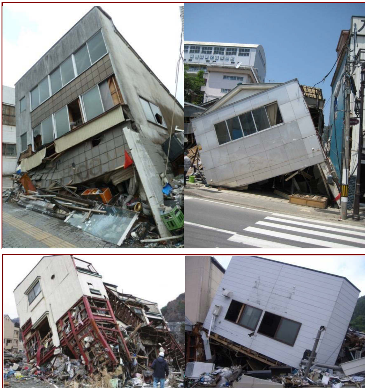
Figure 2.7 Soft-storey and disproportionate collapse.
