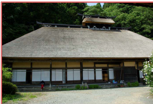
Figure 6.10 (Left) Ogata House before the tsunami.
