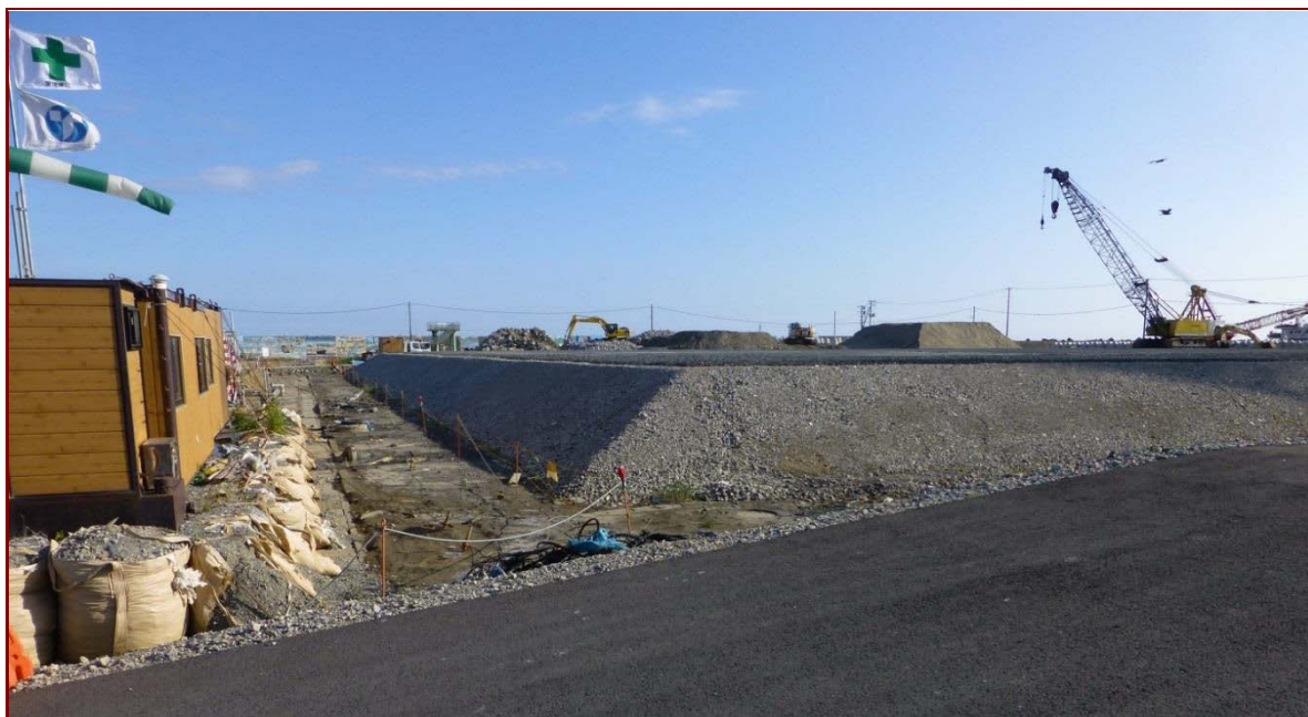
Figure 3.15 Elevated ground level at Ishinomaki fishing port.
