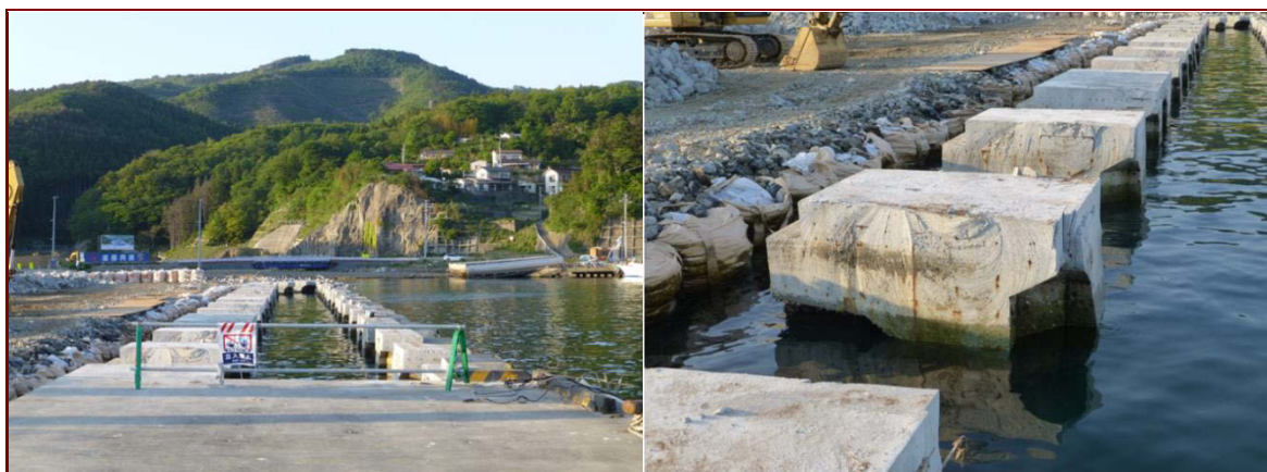
Figure 3.24 Bridge piers for new quay in Onagawa.
