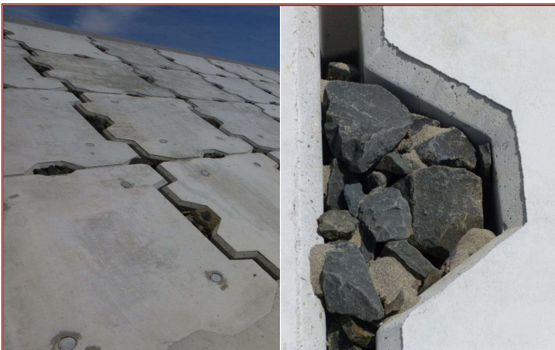
Figure 3.3 (top left) Seaward slope of newly built concrete revetment at Arahama.
