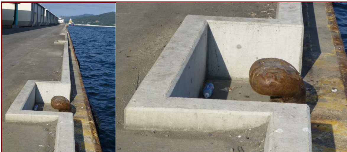
Figure 3.20 (left) Renovated quay wall at Ishinomaki fishing port.
