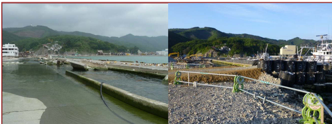
Figure 3.23 Pair of photographs taken in the 2011 (left) and 2013 (right) EEFIT missions, towards the southern end of Onagawa port.
