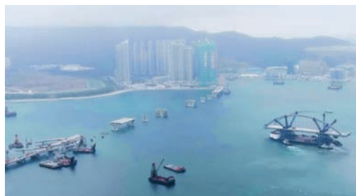
FIGURE 8: Fabrication and delivery of double-arch steel bridge of Cross Bay Link
