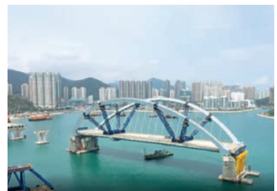
FIGURE 8: Fabrication and delivery of double-arch steel bridge of Cross Bay Link
