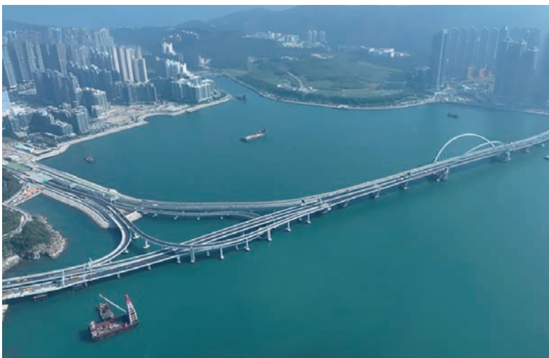
FIGURE 9: Completed Cross Bay Link
