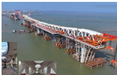
➤ FIGURE 11: Fabrication and installation of mega trusses of Macau Bridge
