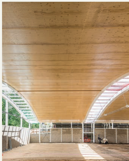
FIGURE 1: LVL was used for roof of Hurlingham Club, London
