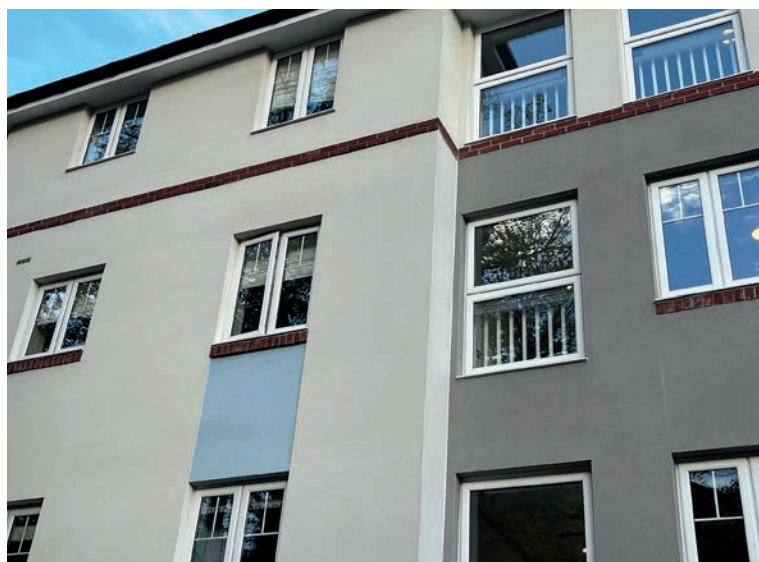
FIGURE 2: Elevation of residential building with AOVs – the AOVs are indistinguishable from standard windows
