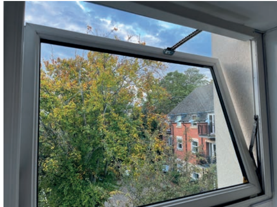
FIGURE 1: AOV in open position
