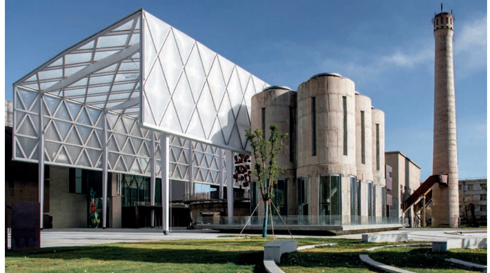
↘ Art bookstore within Tibetan Art Museum was transformed from former cylindrical cement slurry storage tanks
