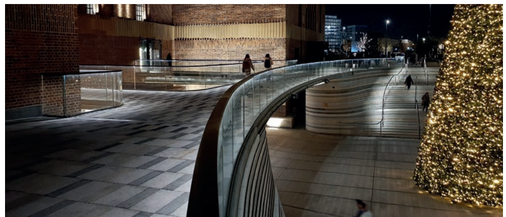
↓ FIGURE 2: Malaysia Square Pedestrian Bridge after completion
