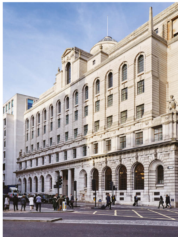
▼FIGURE 1: Redevelopment of 27 Poultry – The Ned – was key project for Gowler
