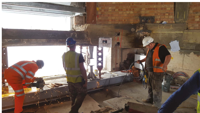
FIGURE 3: Exposed structure during jacking of dome
