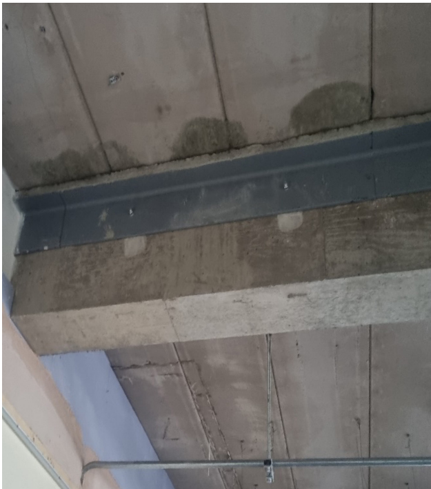
End bearing strengthening
