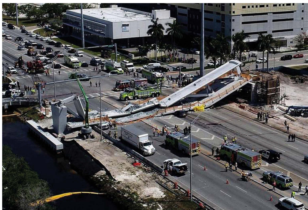
FIGURE 1: The Florida bridge collapse in 2018 was attributed to failings by both the design team and the site engineer 1
