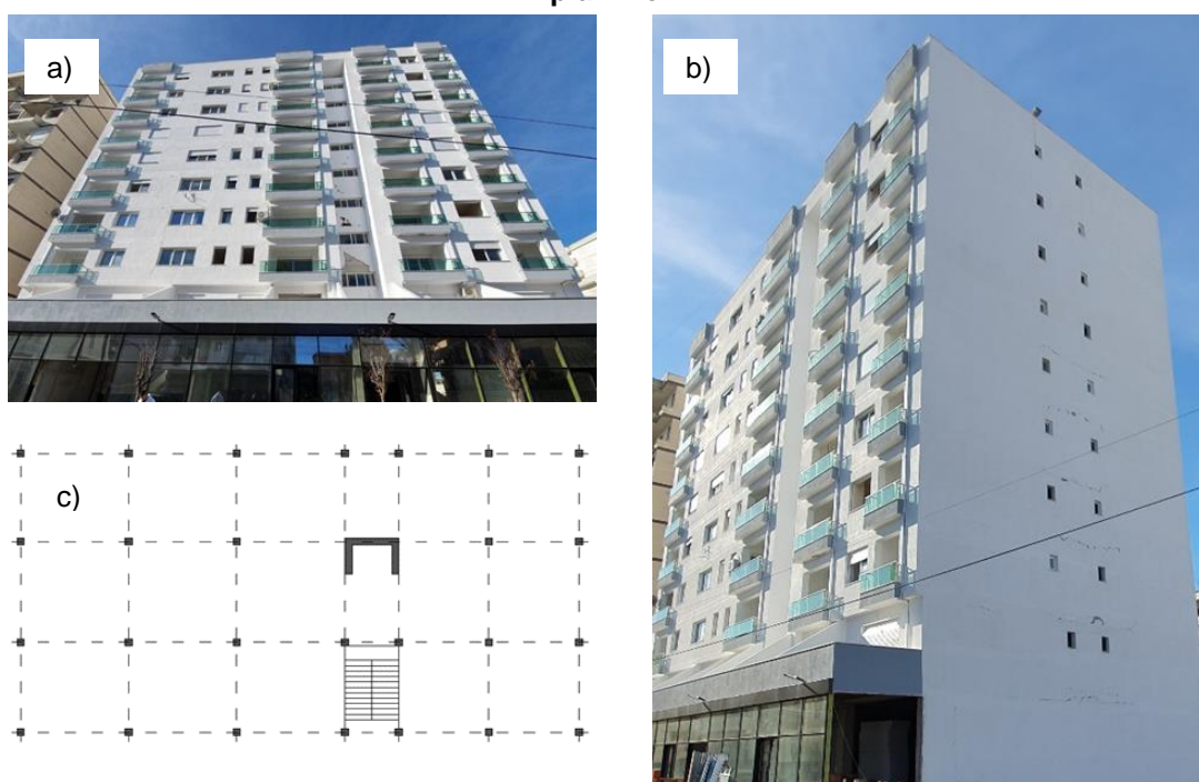
Figure 7.24: Typical post-2010 multi-storey RC building compliant with KTP-N.2-89 with integrated aspects of Eurocode 8: a) north-east facade; b) south-east side; c) indicative plan view
