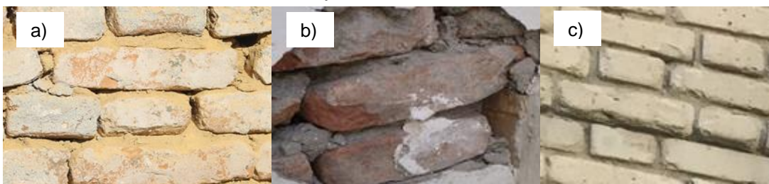
Figure 7.3: Typical bricks for URM buildings. Solid clay bricks with a) silicate mortar; b) cement mortar; c) silicate bricks with silicate mortar
