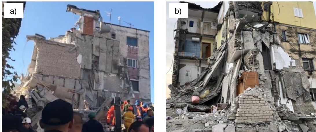
Figure 5.19: Two five-storey calcium-silicate masonry buildings in Kodër-Thumanë that caused 24 fatalities
