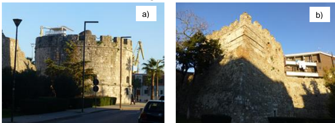
Figure 7.34: Visible repairs of the walls and towers of Durrës (a) Venetian tower and (b) gate tower
