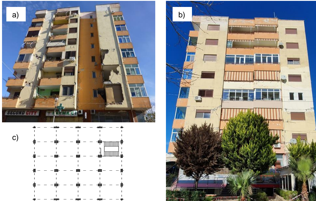
Figure 7.19: Typical 2000s multi-storey RC building compliant with KTP-N.2-89: a) east façade; b) south façade; c) indicative plan view
