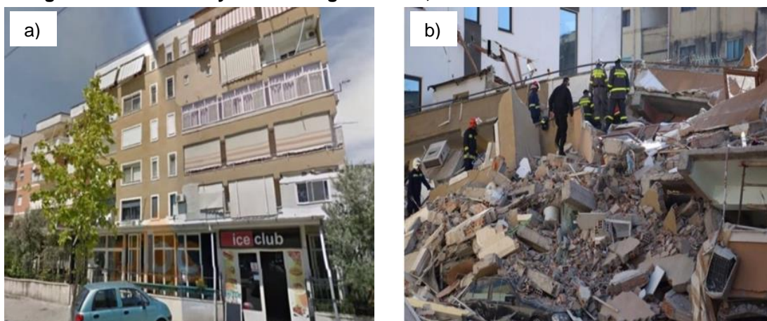
Figure 5.13: Six-storey RC building in Durrës, built in 1996 that caused 7 fatalities
