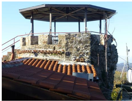
b) new construction adjacent to the tower
