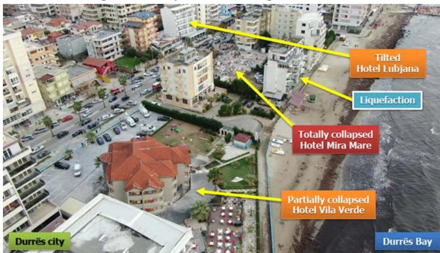
Figure 2.7: Liquefaction along Durrës beach
