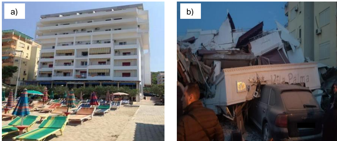
Figure 5.17: Eight-storey RC hotel in Durrës that caused 1 fatality
