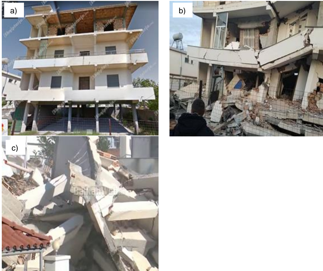
Figure 5.12: Four-storey RC building in Durrës that caused 8 fatalities
