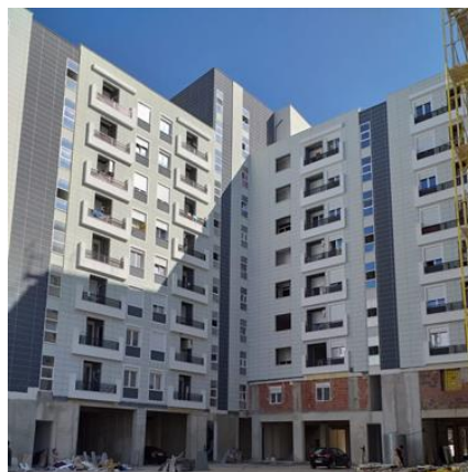
d) New RC building (under construction)
