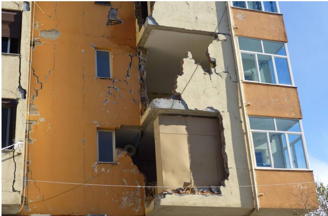
Figure 7.23: Typical 2000s multi-storey RC building compliant with KTP-N.2-89: damage layout on the eastern façade of the building, closeup
