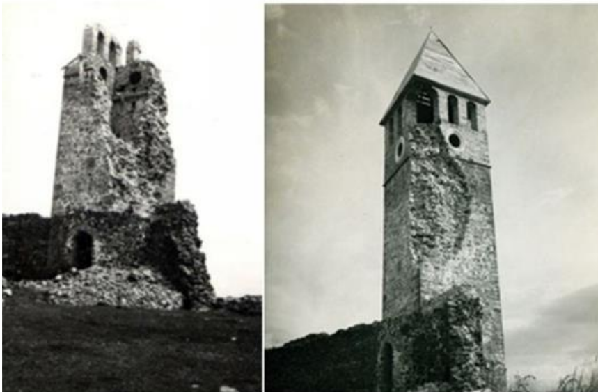
Figure 7.46: Damage suffered by the Prezë castle clock tower at different times [7.18]
