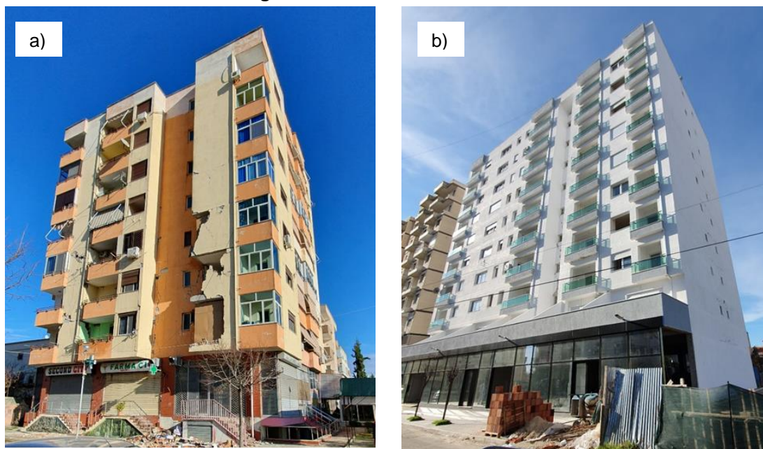
Figure 7.17: Example of typical RC multi-storey buildings. a) Typical 2000s building compliant with KTP-N.2-89; b) Typical post-2010 building compliant with KTP-N.2-89 with integration based on the Eurocode 8
