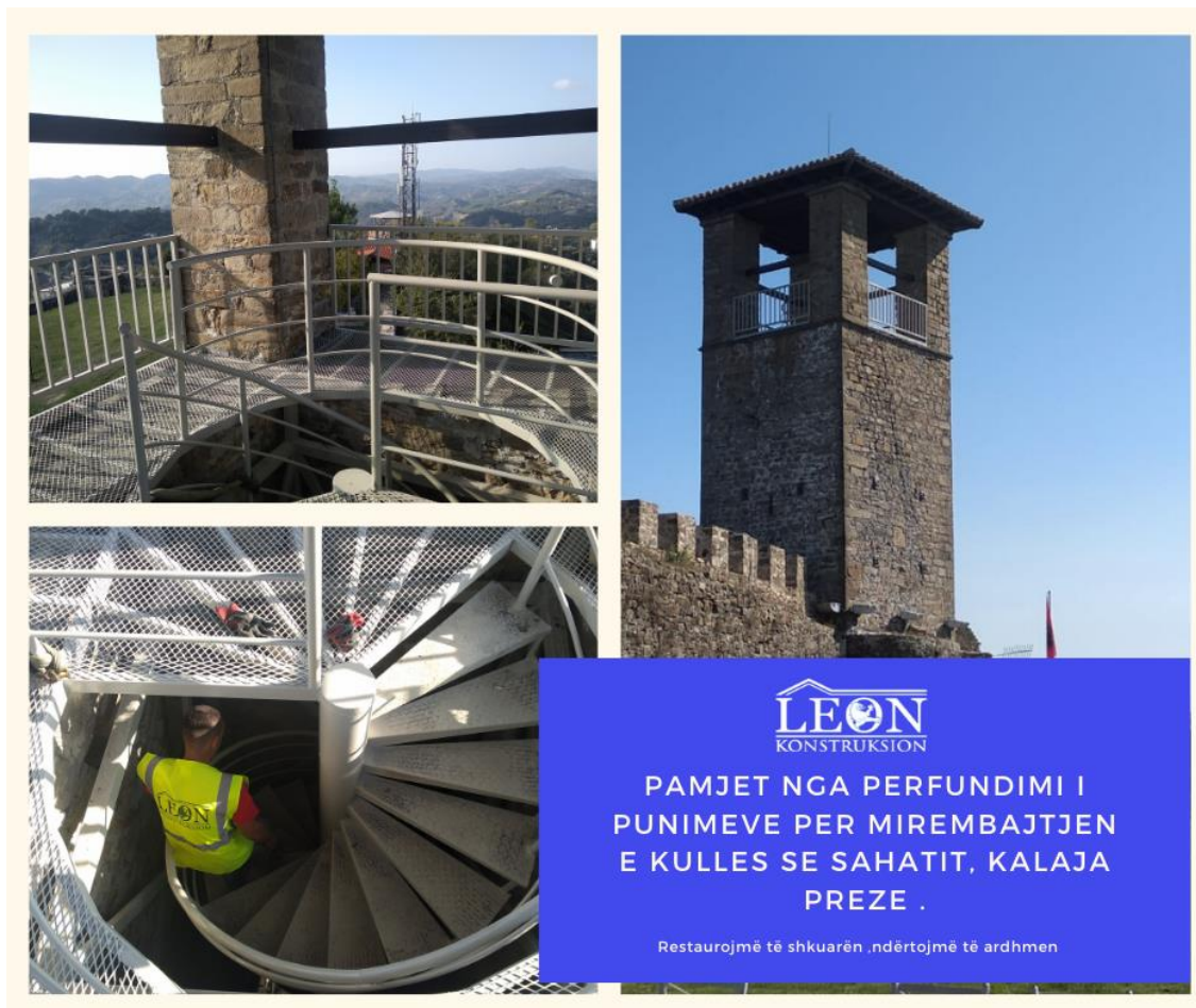
Figure 7.47: Photos showing the intervention on Prezë clock tower in summer 2019
