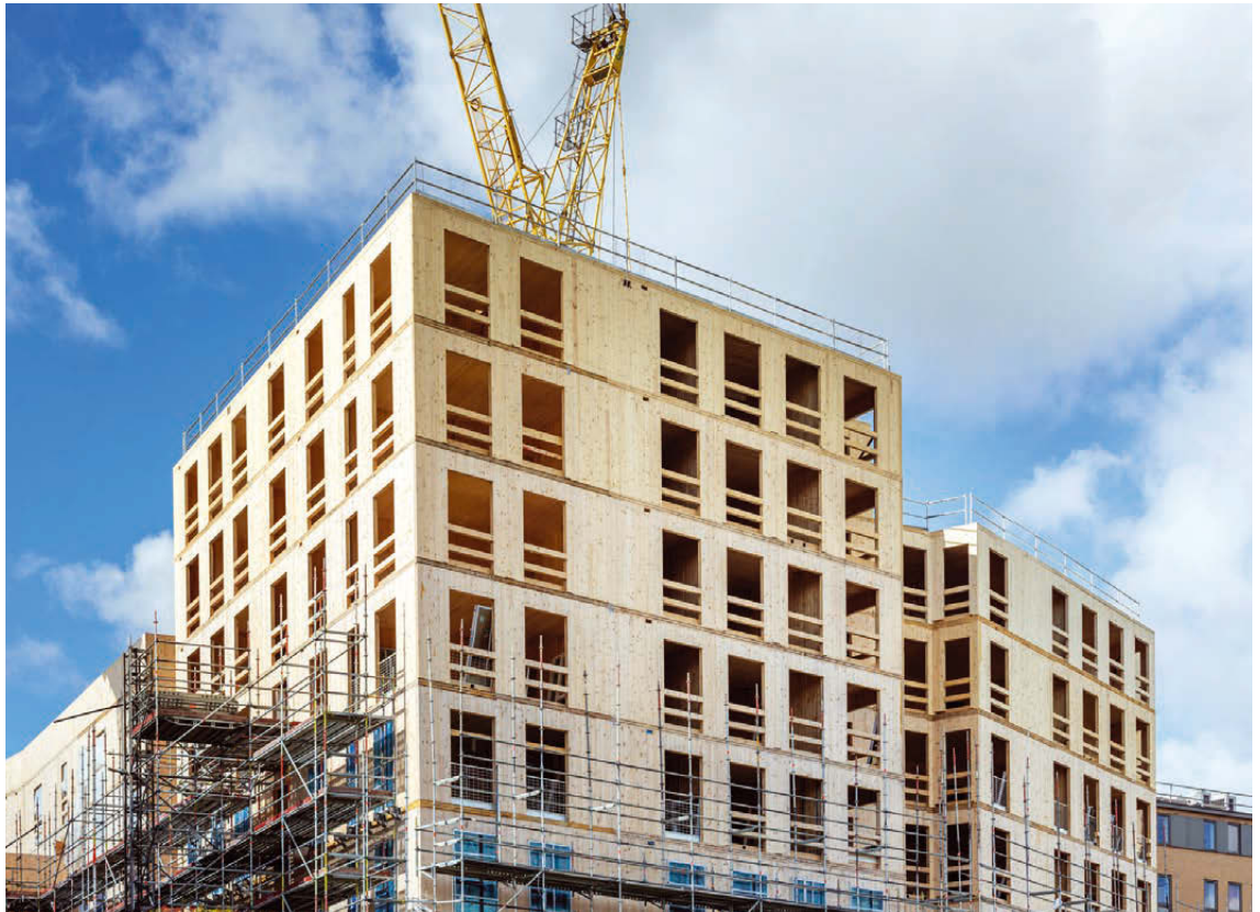
FIGURE 9: Dalston Works under construction, London
