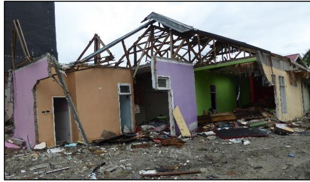
Figure 7.10 – Heavily damaged CM houses in Palu bay area along the Jl. Rajamoili road, about 100m from coastline. The walls of this house were directly hit by the tsunami inundation.
