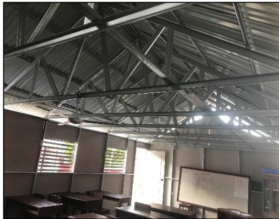
(a) Light steel framed structure
