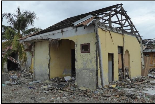
Figure 7.10 – Heavily damaged CM houses in Palu bay area along the Jl. Rajamoili road, about 100m from coastline. The walls of this house were directly hit by the tsunami inundation.
