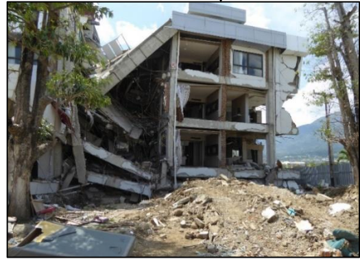
Figure 7.45 – Mercure Hotel, which suffered soft-storey failure of ground floor. Top – Image of the hotel before the earthquake, Source: Tripadvisor.com. Bottom – Pictures of the Hotel after the earthquake, showing the soft-storey failure of the ground storey of the structure.
