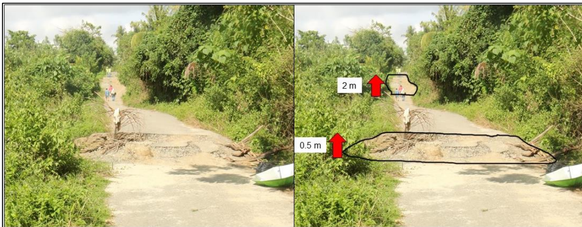
Figure 3.7 – Normal faulting observed North of Labua on the East side of Palu Bay. Photo taken facing North East
