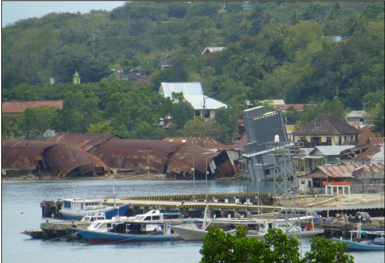
Figure 7.59 - Damage to old port of Donggala
