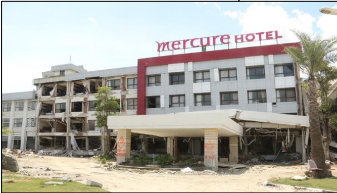
Figure 7.45 – Mercure Hotel, which suffered soft-storey failure of ground floor. Top – Image of the hotel before the earthquake, Source: Tripadvisor.com. Bottom – Pictures of the Hotel after the earthquake, showing the soft-storey failure of the ground storey of the structure.
