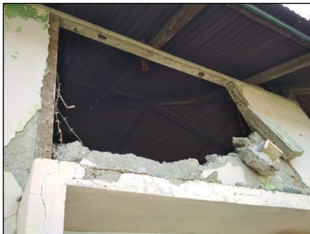
Figure 7.8 - Typical earthquake damage observed in infilled timber frame construction. Left - Out-of-plane failure of infill panels. Right - Separation of infill from frame due to differential settlement of foundations.
