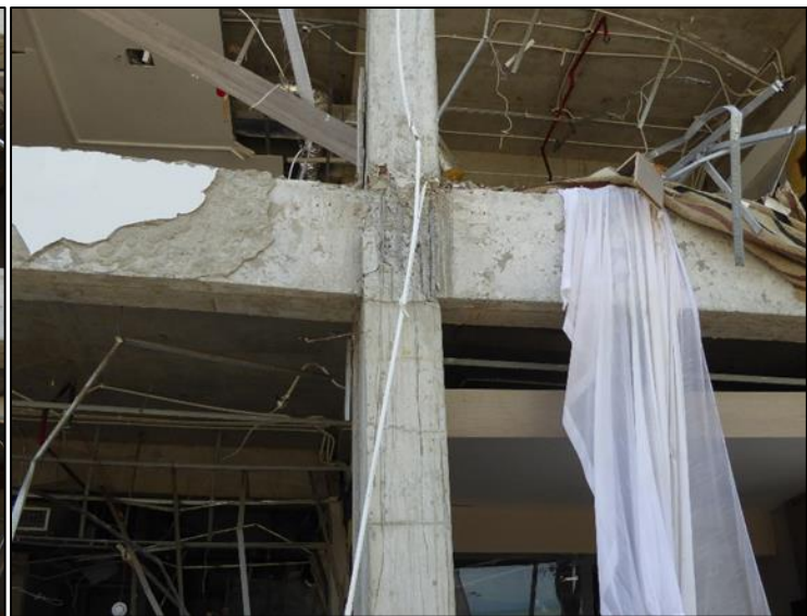
Figure 7.46 – Mercure Hotel – Images of cover spalling in RC frame joints in the second storey of the structure
