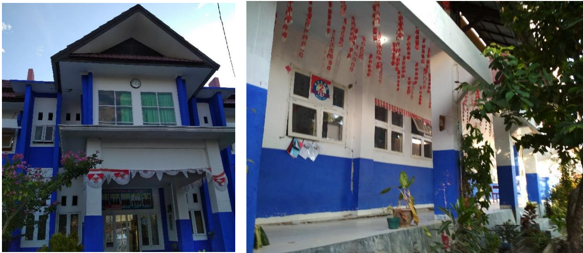
Figure 7.34 - SMP Negeri 1 Biromaru School, Building A in Fig. 7.24a. Left – front entrance to the building. Right – the rear of the building showing columns that support the balcony sited on a 1m high “slab” of made ground covered in concrete screed.
