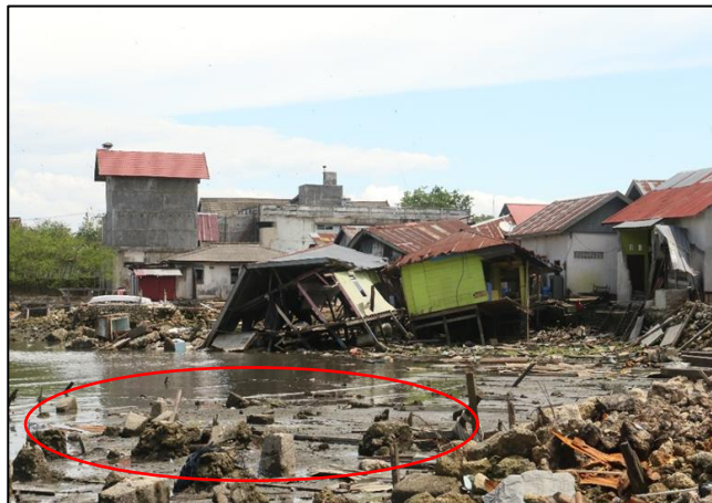
Figure 7.4 - Performance of timber stilt houses in Palu and Donggala, Central Sulawesi: Left – The palace of the Princes of Palu. This structure was affected by ground shaking but not tsunami inundation and was undamaged. Right - The remaining concrete foundations of the timber stilt houses in the Labuan Bajo Fisherman Village, shown in red circle. Collapsed stilt houses can be seen in the background.
