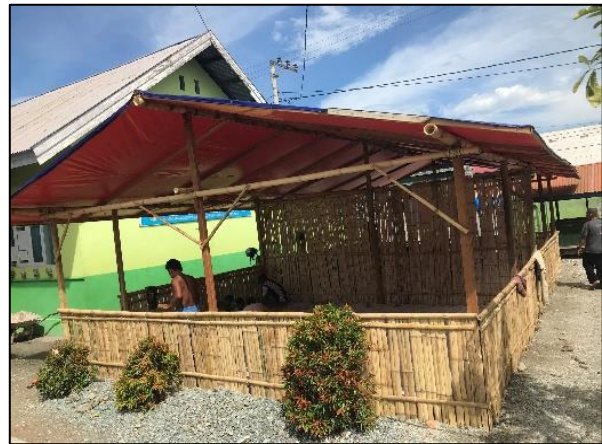
(b) Light bamboo framed structure
