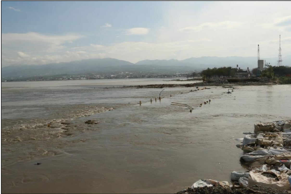
Figure 6.21 - Submerged bridge deck of the Palu Bridge IV which may have acted as a submerged breakwater to the tsunami waves, preventing them travelling up the river
