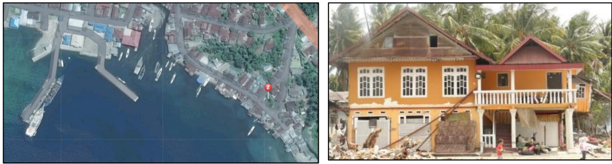
Figure 6.12 - Location (left) and photograph (right) of the house where the man in the car ended up at around 50 m inland from the sea
