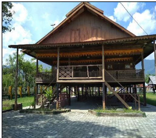
Figure 7.4 - Performance of timber stilt houses in Palu and Donggala, Central Sulawesi: Left – The palace of the Princes of Palu. This structure was affected by ground shaking but not tsunami inundation and was undamaged. Right - The remaining concrete foundations of the timber stilt houses in the Labuan Bajo Fisherman Village, shown in red circle. Collapsed stilt houses can be seen in the background.
