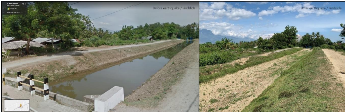
Figure 4.10 – Far northern end of the Bendung Irigasi Gumbasa irrigation channel above the head of the Petobo Landslide before (left) and after (right) the earthquake.
