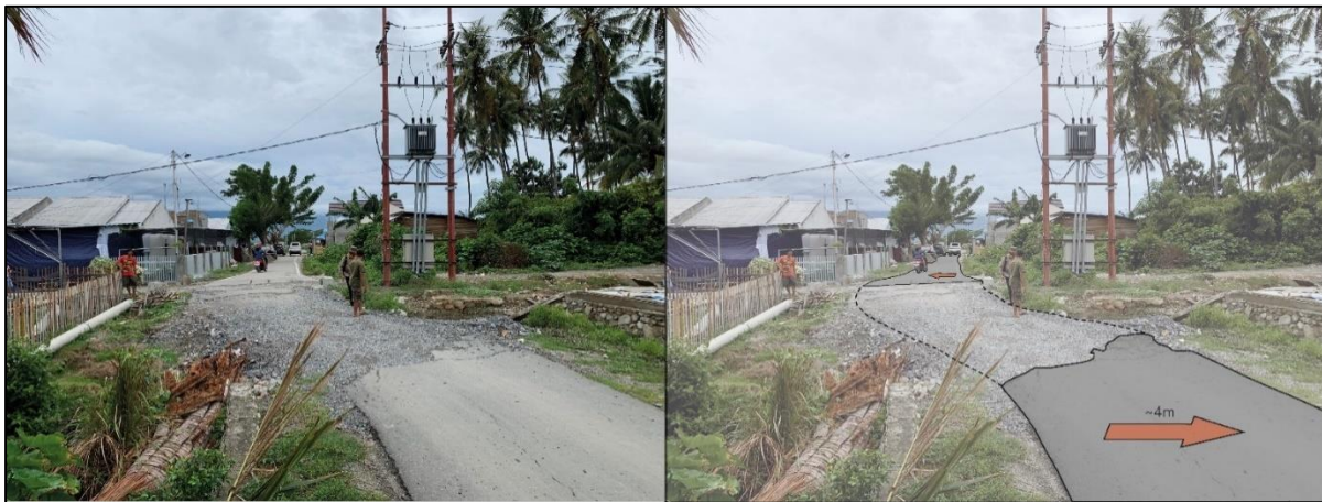
Figure 3.4 – Offset road due to strike-slip fault displacement.
