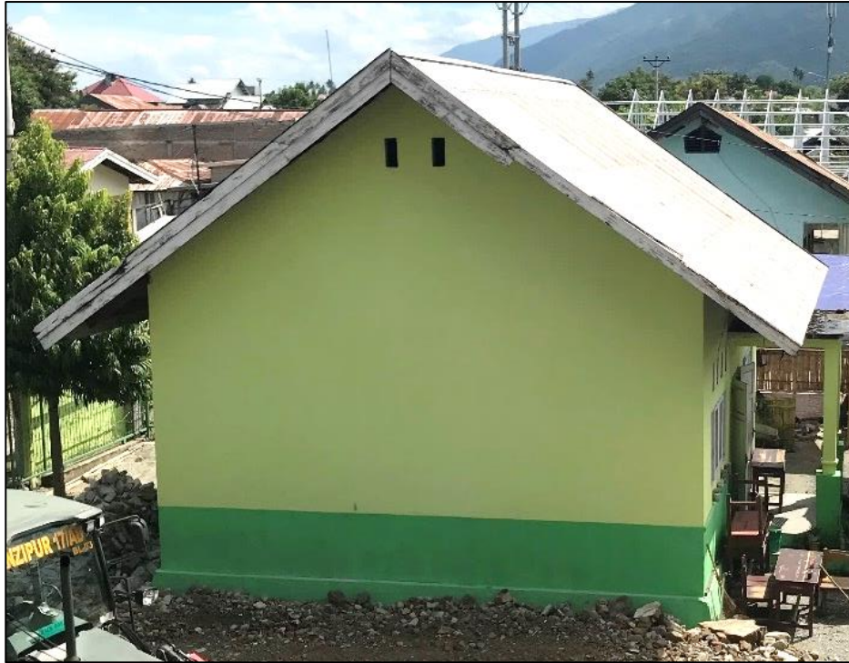
Figure 7.30 - A small plan box-type CM school building that suffered no damage (building B in Fig. 7.24c) in SD Negeri Pengawu school.
