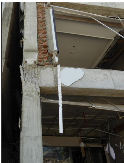
Figure 7.46 – Mercure Hotel – Images of cover spalling in RC frame joints in the second storey of the structure
