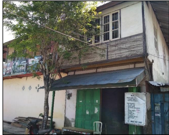
Figure 7.6 - Examples of infilled timber frame construction in Labuan Bajo. Left - Timber framed house with wire-reinforced mortar. Right - Two storey timber framed house with mortar infill.
