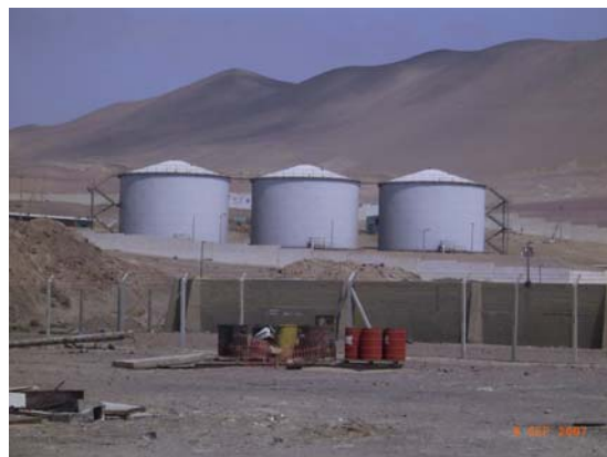
Figure 7.10 Port of San Martín: adjacent steel tanks showing no damage
