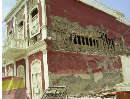
Figure 5.2 Pisco historic waterfront: adobe building with quincha exposed at second storey
