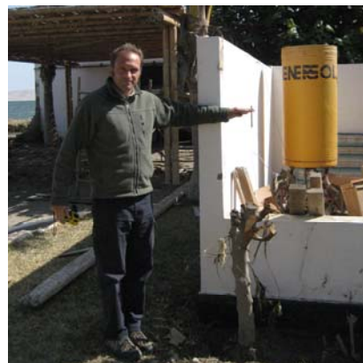
Figure 4.2 Tsunami water height in holiday villas at Paracas
