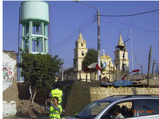
Figure 8.6 Water tower near Guadalupe.
