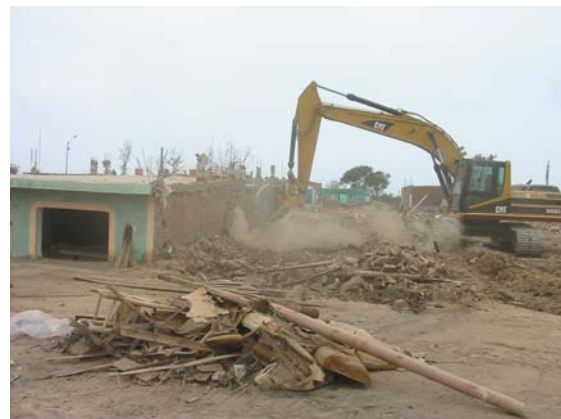
Figure 3.6 Liquefaction affected houses being demolished by the government
