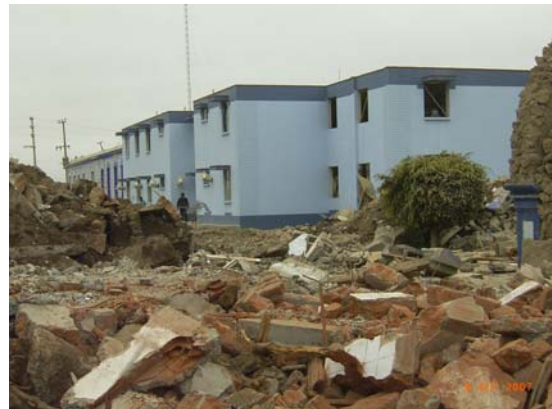
Figure 10.2 New hospital, built prior to the earthquake, next to a previously existing one that was severely damaged and demolished in Pisco
