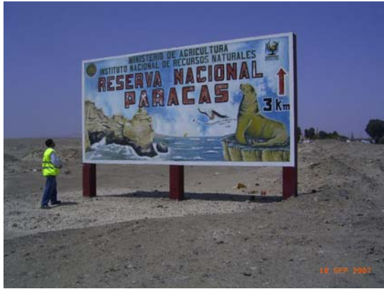
Figure 5.33 RC infilled frame billboard near the Paracas National Reserve
