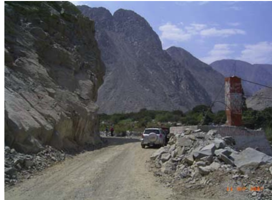
Figure 3.11 Rock fall that hit the abutment of a pedestrian bridge crossing the Cañete river (see point No.2 in Figure 3.8 for location)
