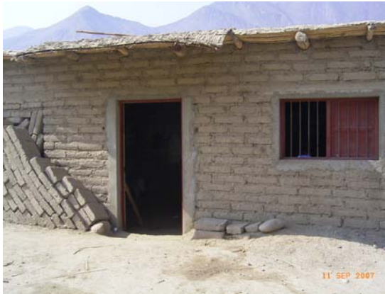
Figure 5.12 Low height adobe houses up the valley of river Cañete showing no damage
