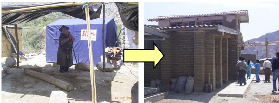
Figure 15.2 A sustainable reconstruction process should lead to the transition from temporary shelters built after the disaster to earthquake resistant designs using local materials and workmanship (Photos from Cañete river valley near Huangáscar)
