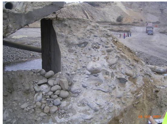
Figure 6.7 Huamaní Bridge: large size round aggregate used in the concrete of abutments
