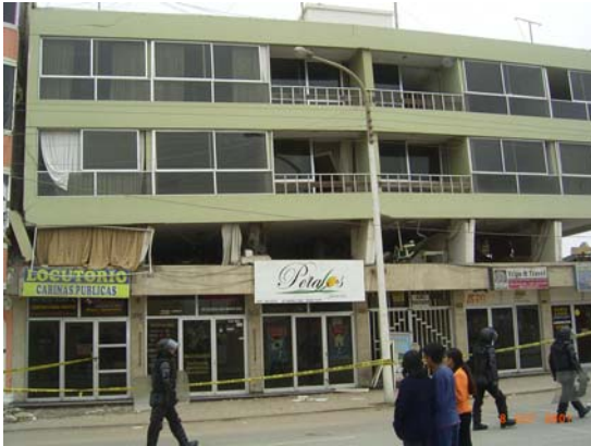
Figure 5.29 Four-storey RC infilled frame in Pisco showing soft storey collapse at 2 nd floor
