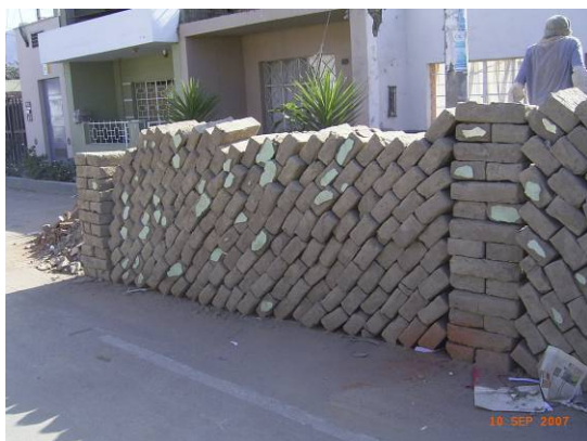
Figure 13.1 Adobe bricks ready for use in reconstruction in Chincha Alta
