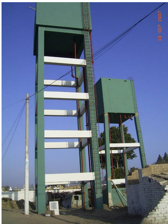
Figure 8.3 Water towers in San Juan (older tank in the background).
