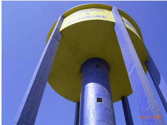
Figure 8.1 Water tank near Guadalupe.
