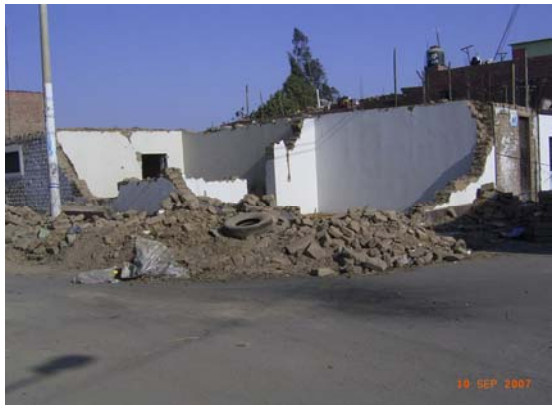
Figure 5.3 Collapsed adobe house in Ica
