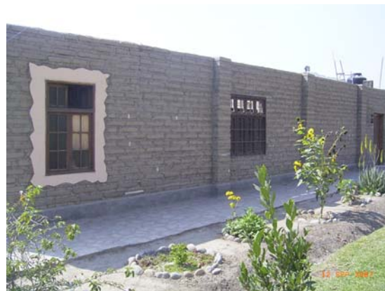
Figure 5.11 Manor in Lunahuaná showing walls laterally supported by machones
