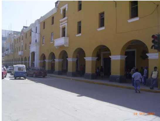
Figure 5.14 Masonry structure in Plaza de Armas, Ica, showing no damage
