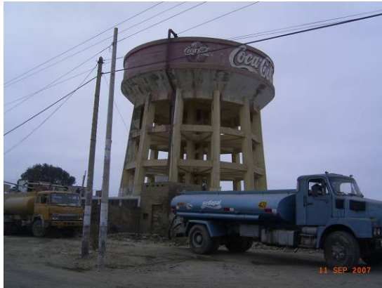
Figure 8.5 Water tower in Pisco.
