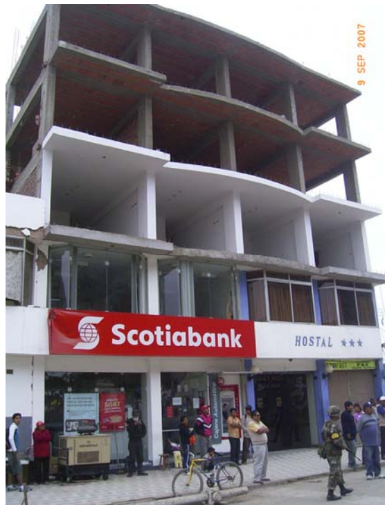
Figure 5.32 Five-storey RC building frame with flat-slabs under construction in Ica
