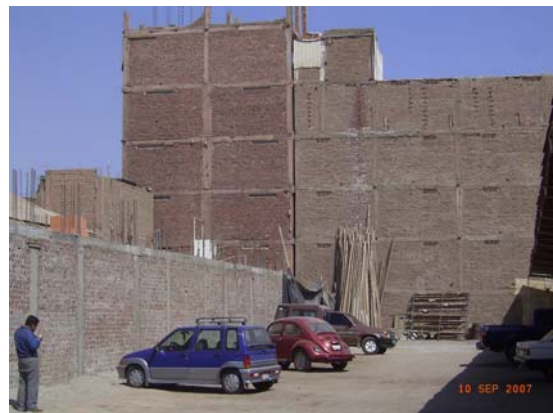
Figure 5.25 Six-storey RC confined masonry building in Ica, showing no signs of damage
