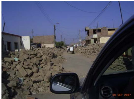
Figure 5.4 Debris of collapsed adobe houses in Ica
