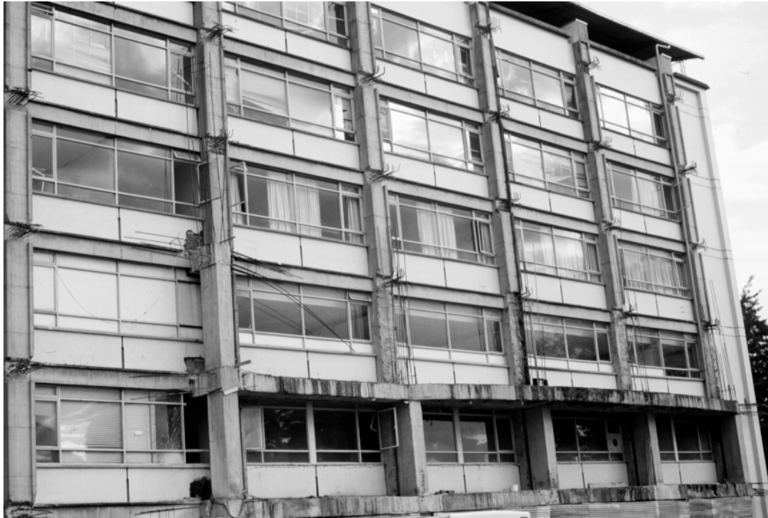
Figure 7.25: General view of Armenia main hospital, showing retrofitting work in progress
