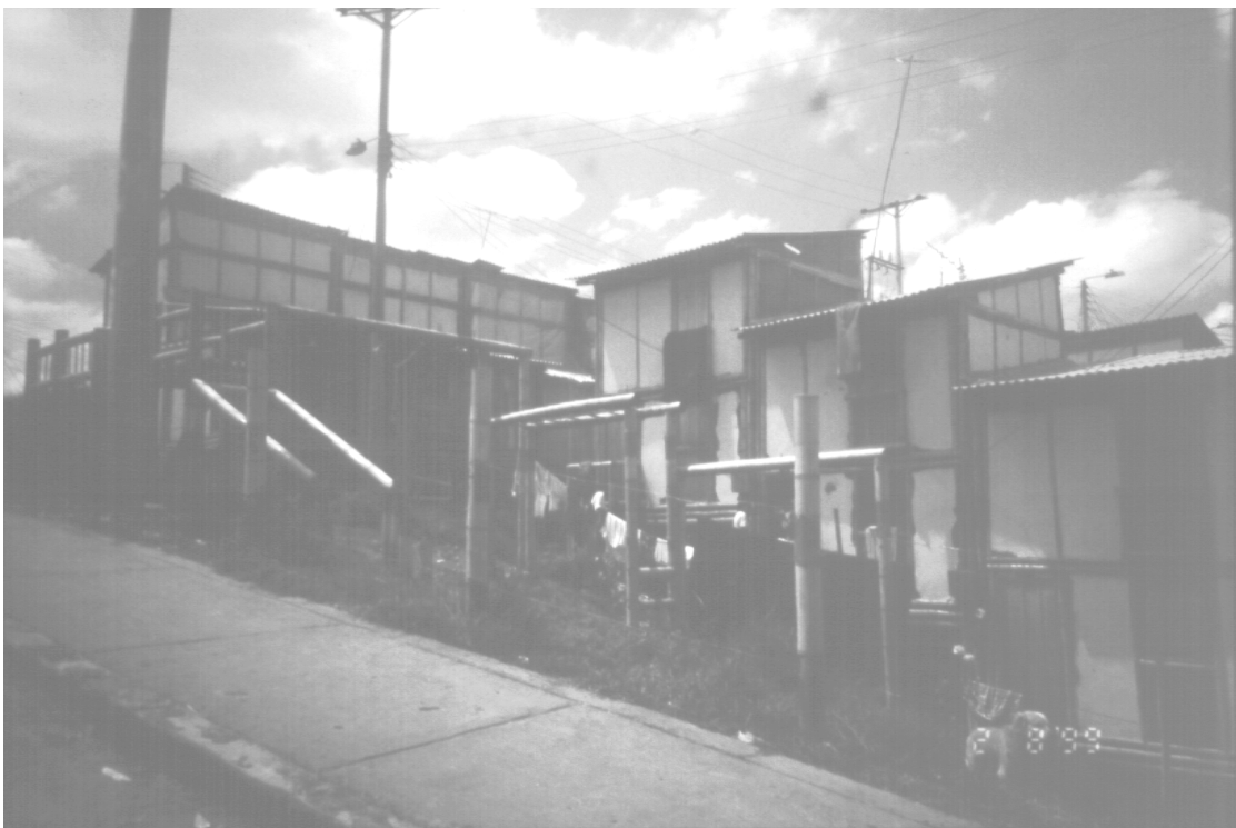
Figure 5.16: Close-up new bamboo houses in Armenia
