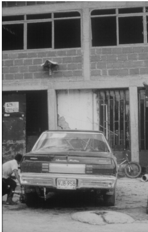
Figure 5.12: Non-coincident beam and column arrangement. Column transfers load to the centre of the beam.
