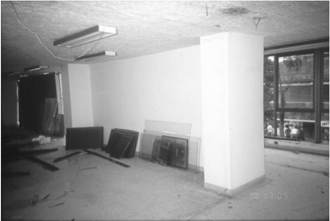
Figure 4.19: Retrofitted shear wall
