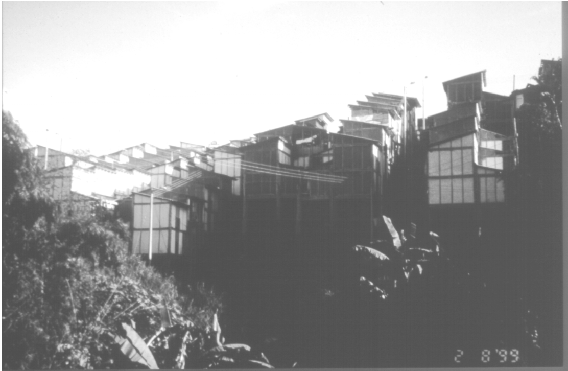
Figure 5.15: Social housing development of new bamboo houses in Armenia
