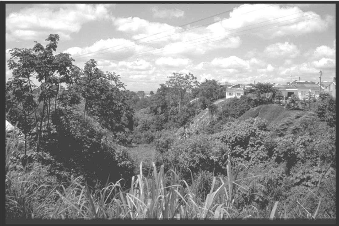
Figure 3.4: Ground failure affecting structure at top of slope
