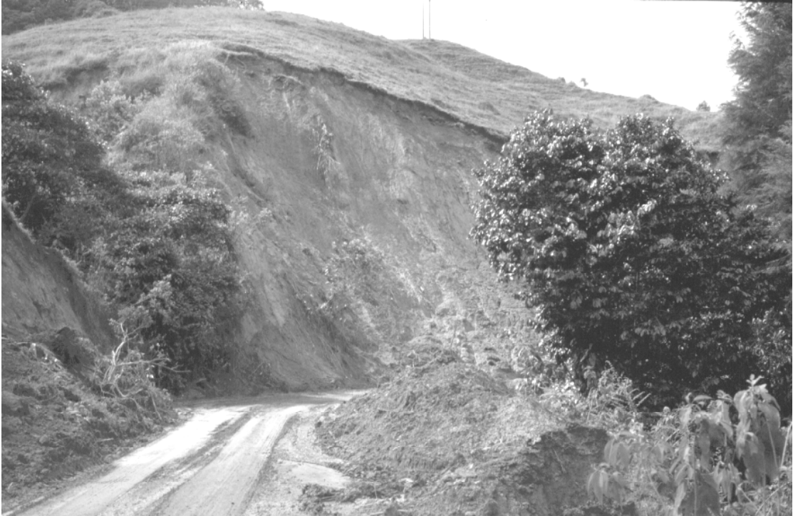
Figure 7.19: Landslides on the road to Pijao
