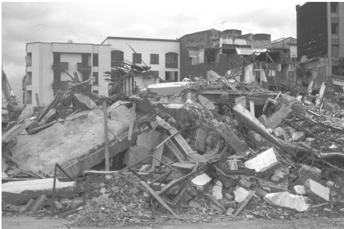
Figure 6.4: Piled debris in Armenia city centre
