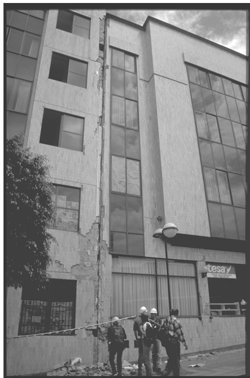
Figure 4.8: Pounding between adjacent structures
