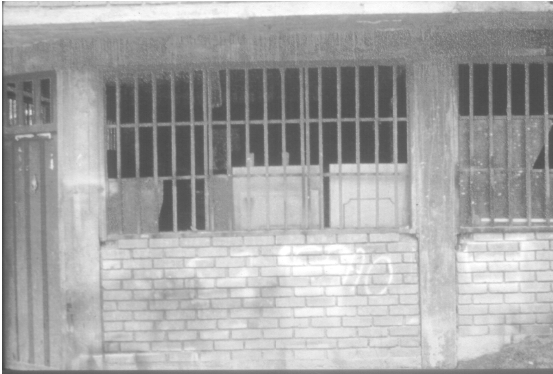
Figure 5.13: Masonry wall built between columns to half storey height to form window
