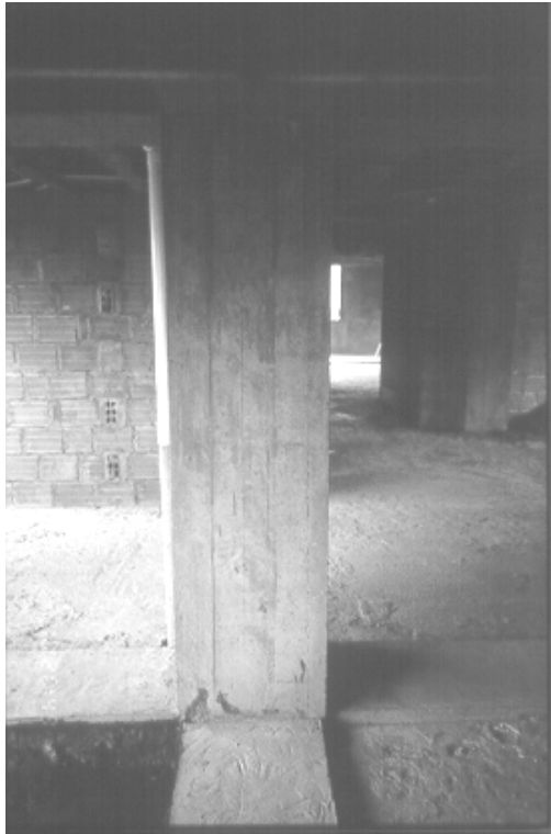
Figure 4.25: Retrofitted column, type C1
