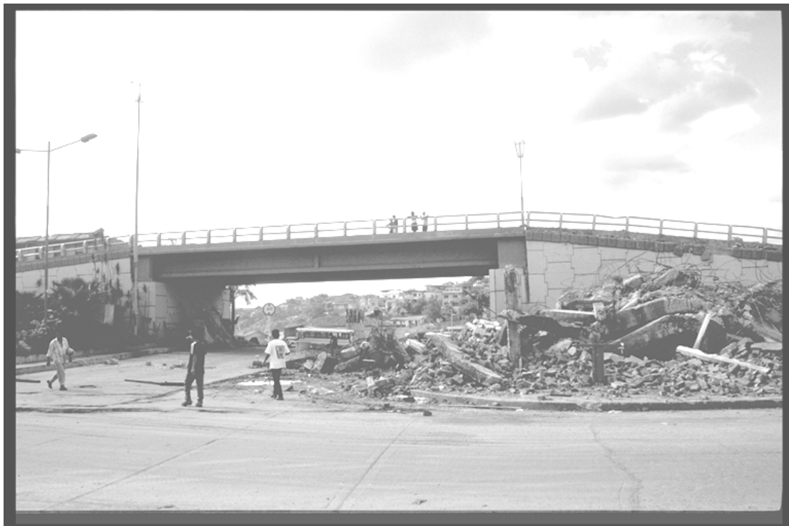
Figure 7.6: Concrete overpass recently constructed in Armenia
