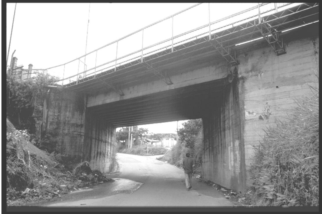
Figure 7.9: Approach bridge to above bridge
