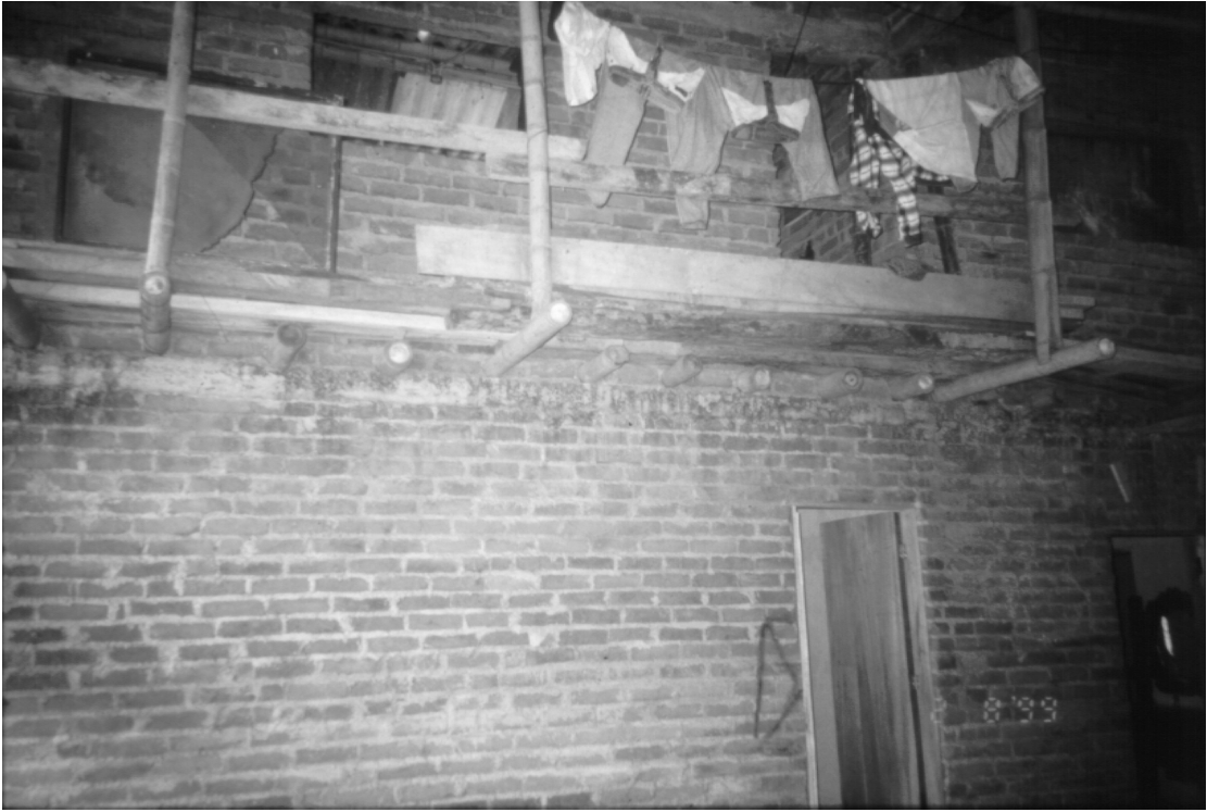
Figure 5.7: Internal wall of house shown in Figure 5.5
