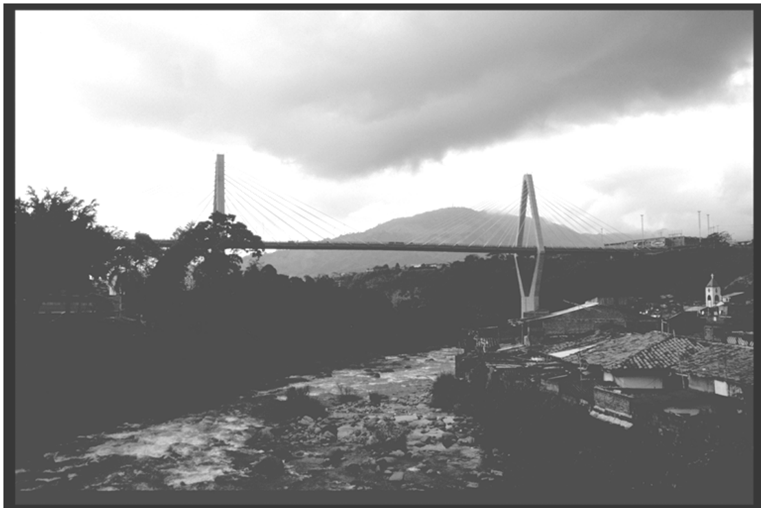
Figure 7.10: Cable-stayed bridge in Pereira
