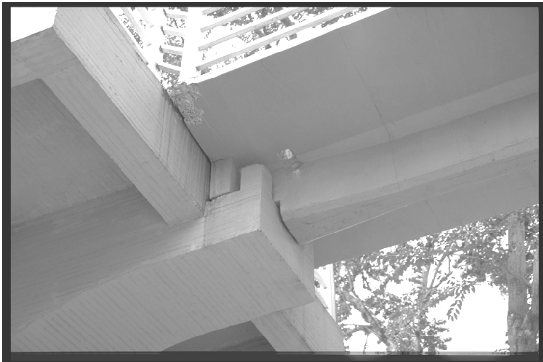
Figure 7.14: Undamaged shear key detail
