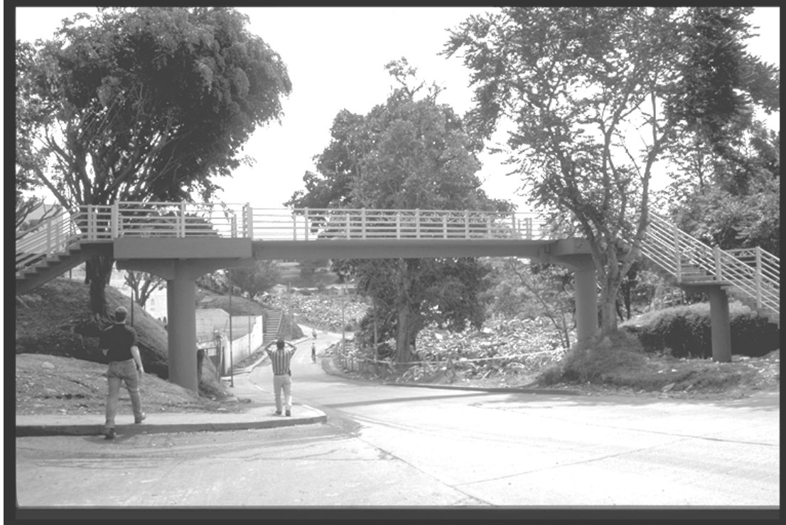
Figure 7.13: Damaged footbridge in south-west of Armenia
