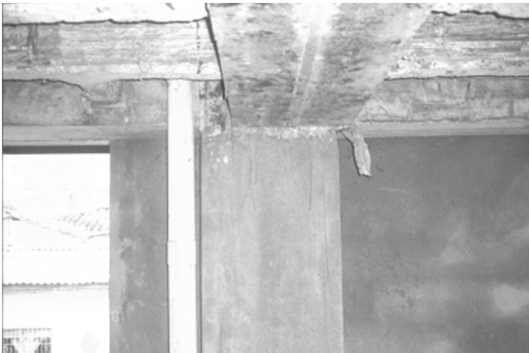
Figure 4.26: Eccentric retrofitted beam and column connection
