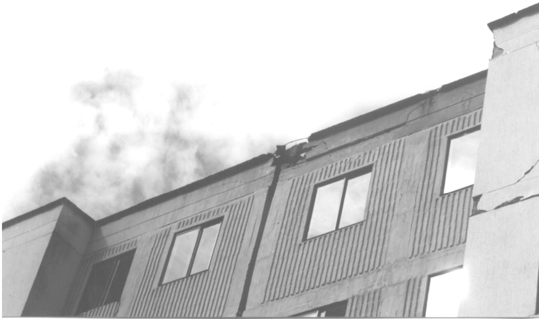
Figure 4.9: Buildings with tie spanning seismic gap
