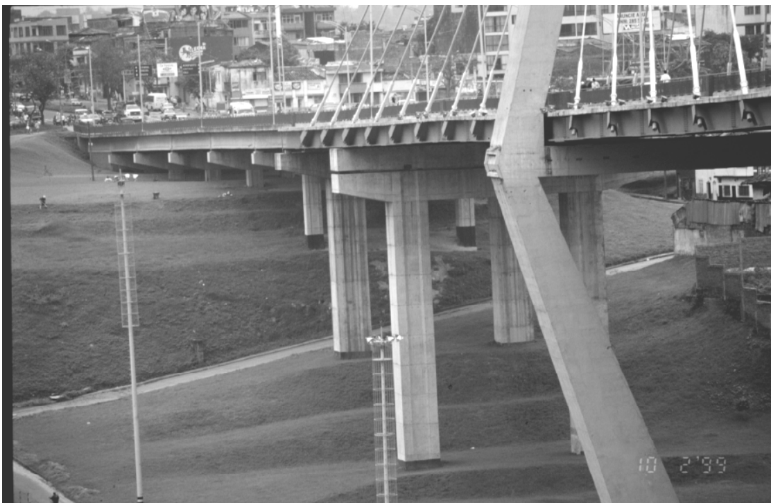
Figure 7.12: Approach viaduct to Pereira cable-stayed bridge
