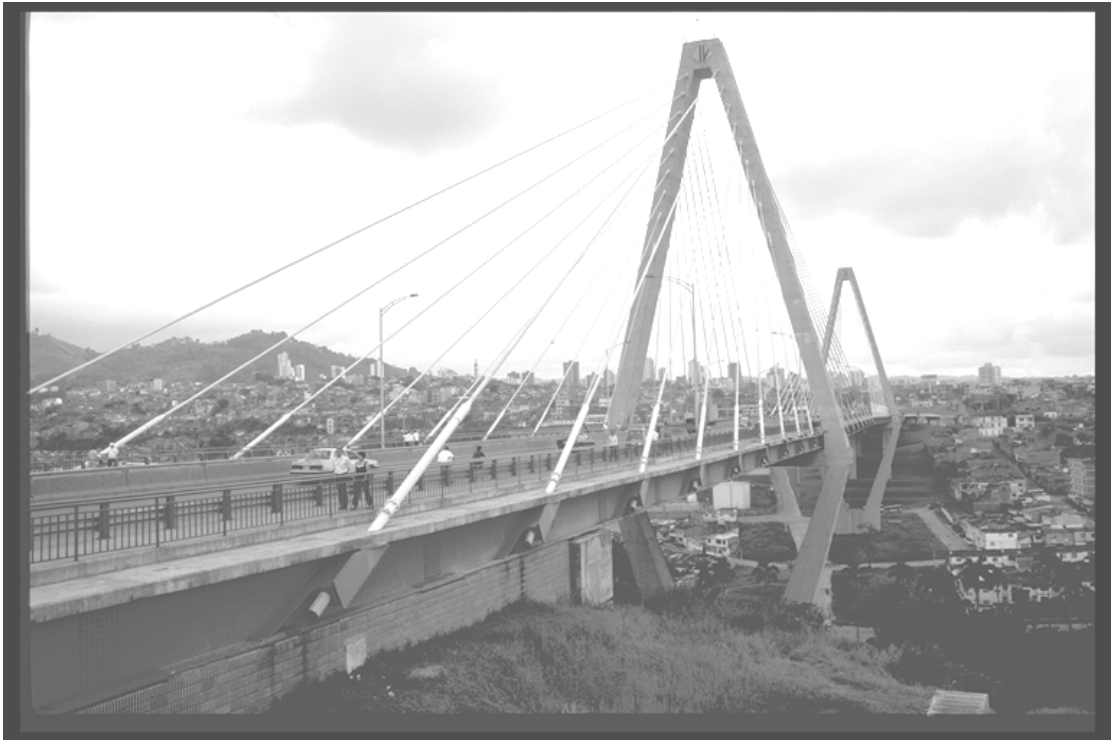
Figure 7.11: View of Pereira cable-stayed bridge from north
