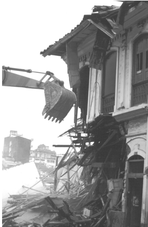
Figure 6.3: Demolition of damaged buildings in Armenia city centre
