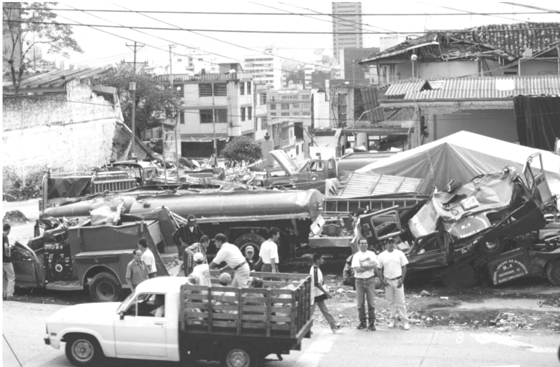
Figure 7.21: Collapse of Armenia fire station, showing heavy damage to equipment
