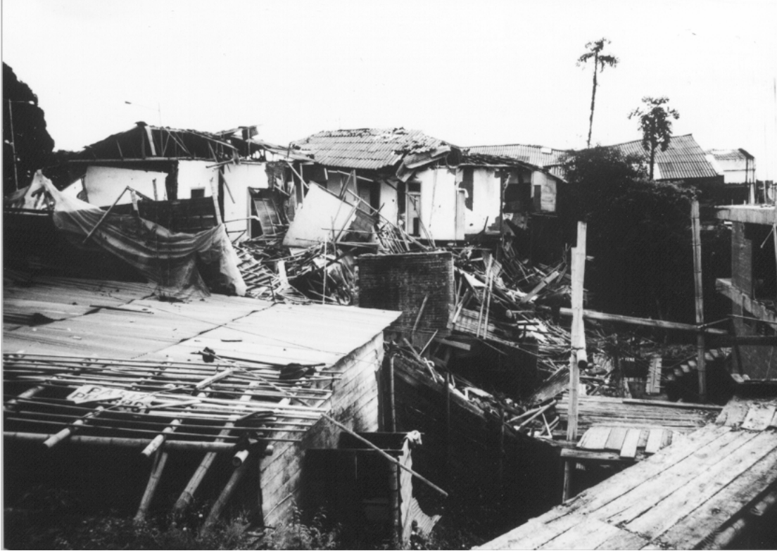
Figure 3.3: Traditional bahareque structures – Armenia (south)
