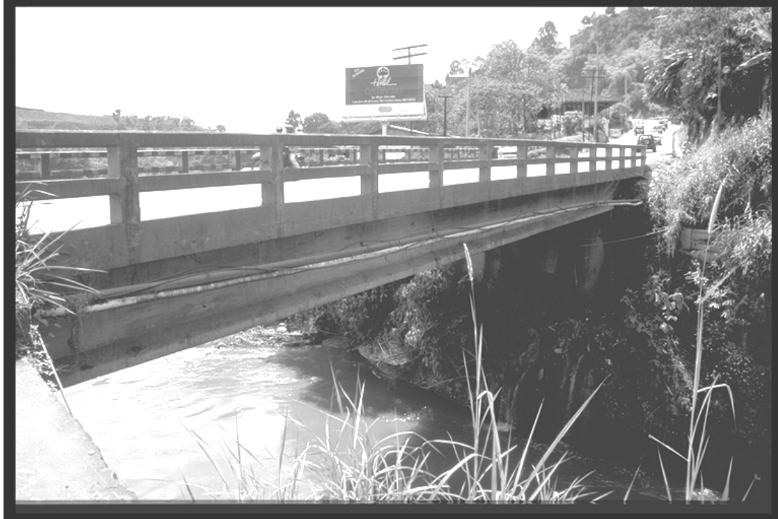
Figure 7.1: Single span concrete bridge over River Quindío on Armenia-Calarcá road
