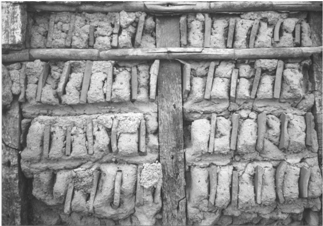
Figure 5.4: Wall construction of a bahareque building, showing tiles embedded in mud infill
