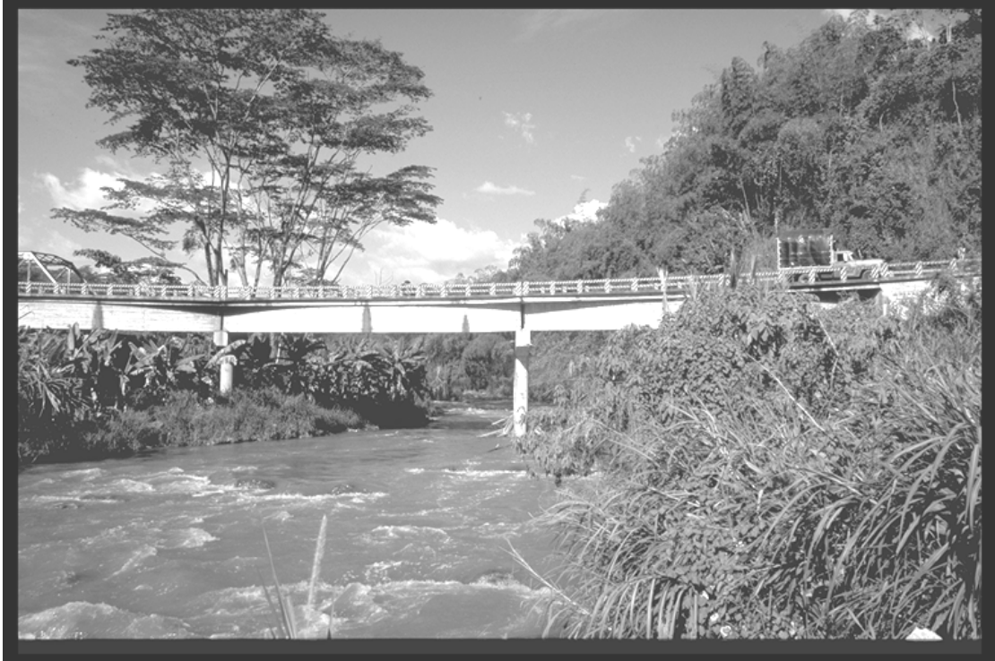
Figure 7.3: Four-span concrete bridge over the River Quindío south of Armenia
