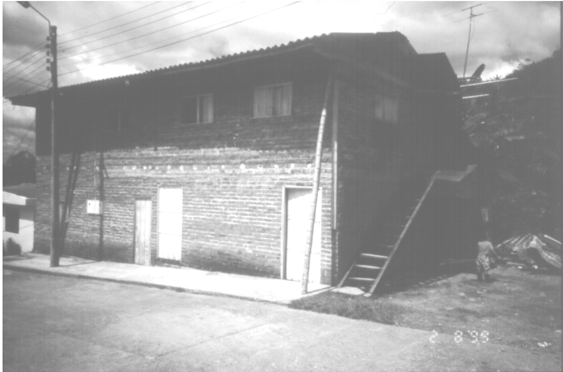
Figure 5.5: Masonry building with ring beams at first floor and roof level. Note bamboo sections above ring beam forming the main structural floor members.
