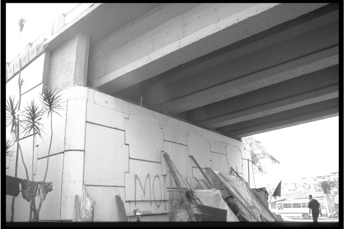
Figure 7.7: Detail of above bridge
