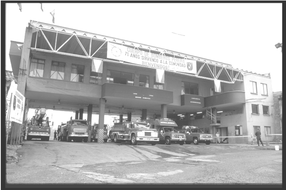
Figure 7.23: The fire station in Pereira, which suffered very little damage
