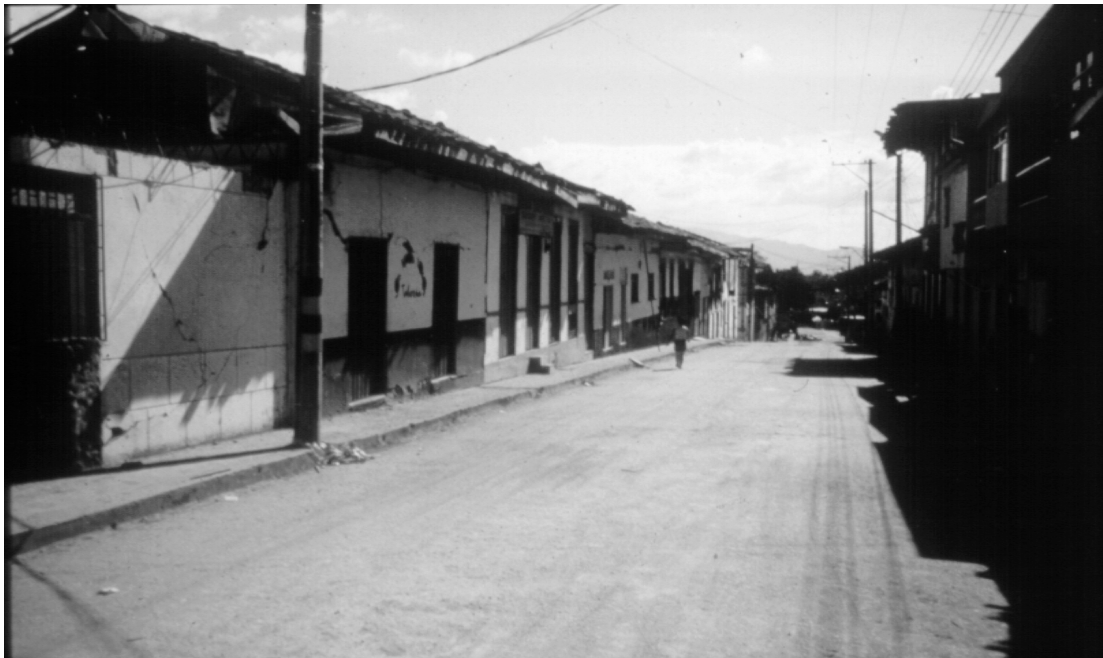
Figure 5.2: Terrace of relatively undamaged bahareque buildings in Barcelona
