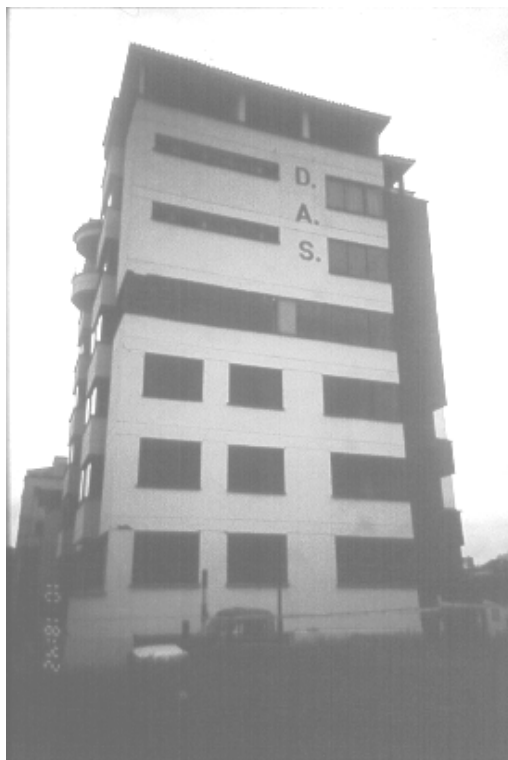
Figure 4.22: The D.A.S. Building
