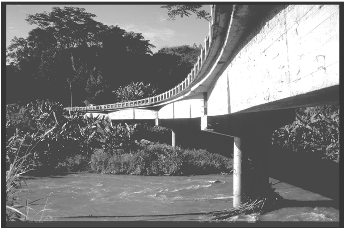
Figure 7.4: Above bridge, showing curve
