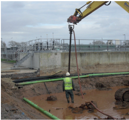
Figure 3 Wellpoint dewatering. Installation on site, using jetting tube
