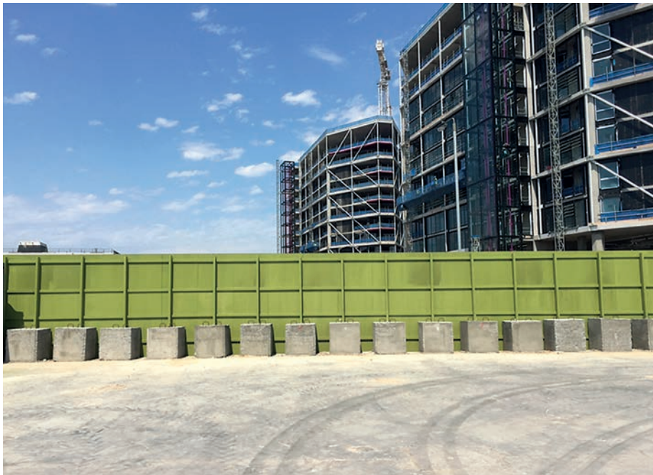
Figure 2 Example of kentledge hoarding seen from site side
