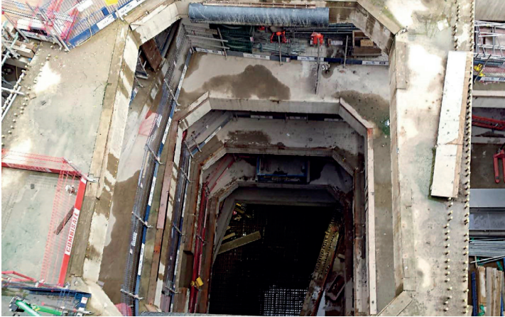
Figure 15 Top-down construction of trapezoidal shaft SH-E3 with provision for construction access
