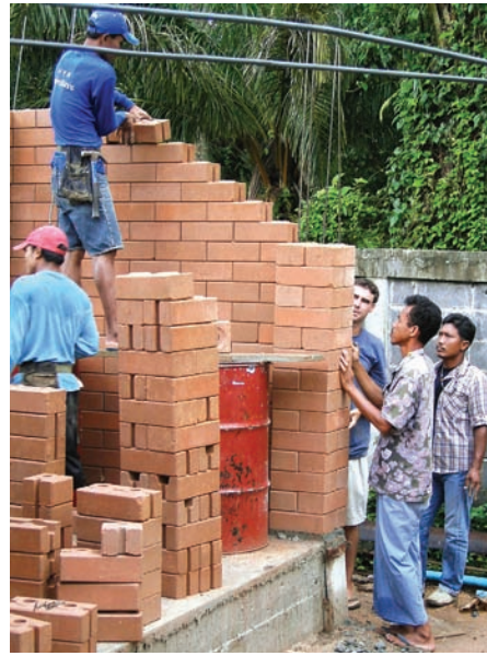
Figure 1 In Thailand with charity Habitat, Julia's role was to develop designs for house construction that could be built by homeowners and unskilled volunteers. In addition to the standard RC frame with block infill walls prescribed by the charity, she developed designs using locally manufactured cement stabilised interlocking earth blocks; a more sustainable solution.
