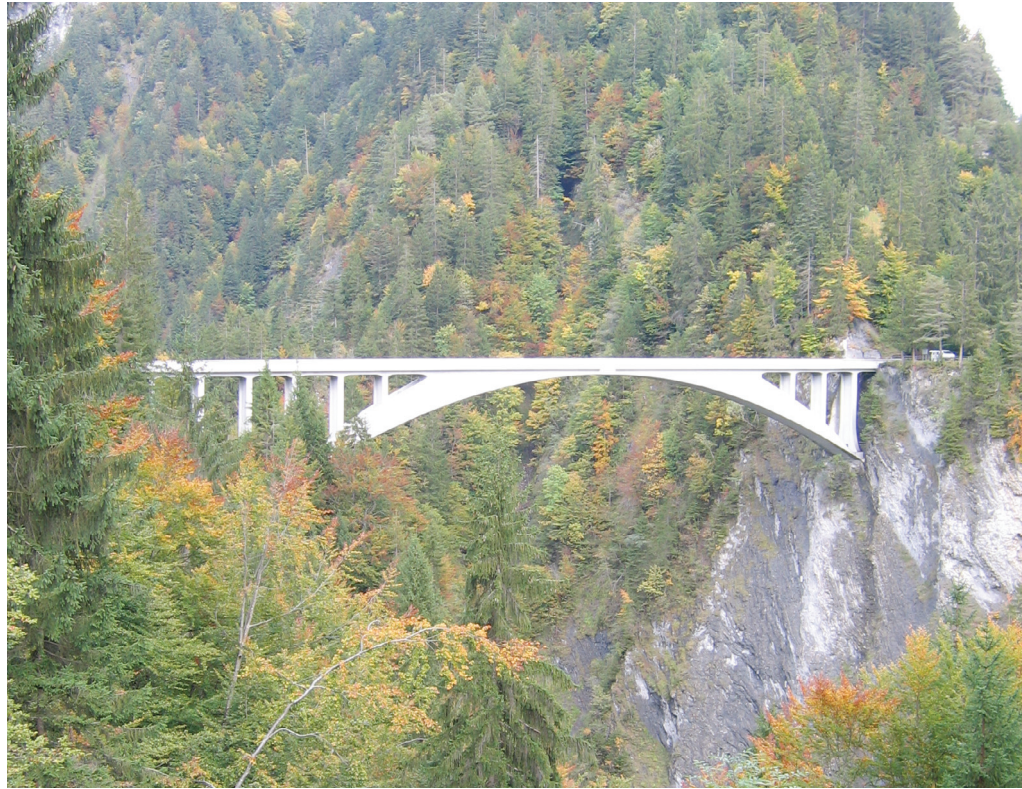
Figure 9 R. Maillart, Salginatobel Bridge, Switzerland
