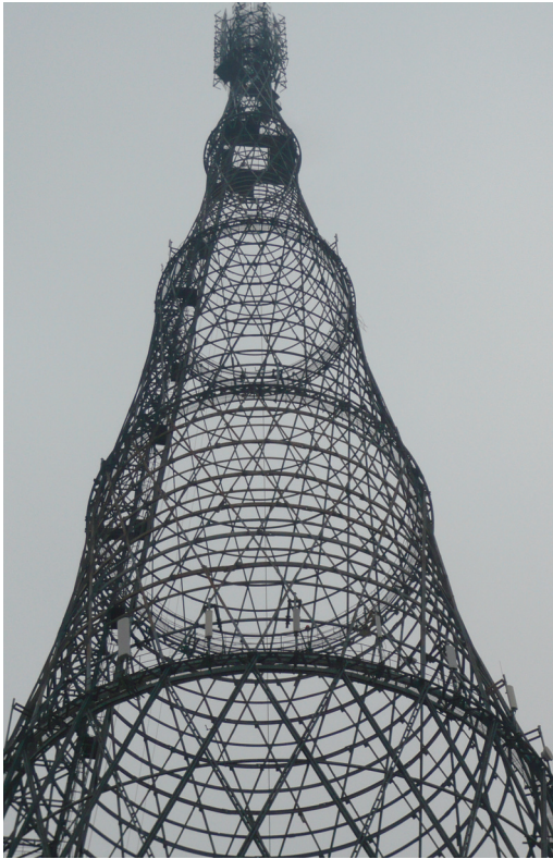
Figure 8 V. Shukhov, Shabolovka Tower, Russia
