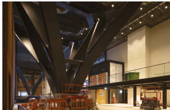
➤ Boiler House's tree-shaped steel structure supports
