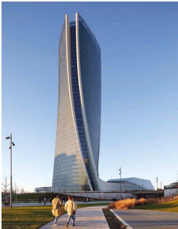
▼ FIGURE 1: The unique twisting form of the Generali Tower in Milan by Zaha Hadid Architects was realised by Williamson-Taylor's AKT II team
