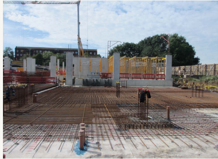
↓FIGURE 4: Typical below-ground site – ready for concrete slab pour
