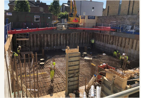
↓FIGURE 5: Below-ground site – prior to watertight concrete pour
